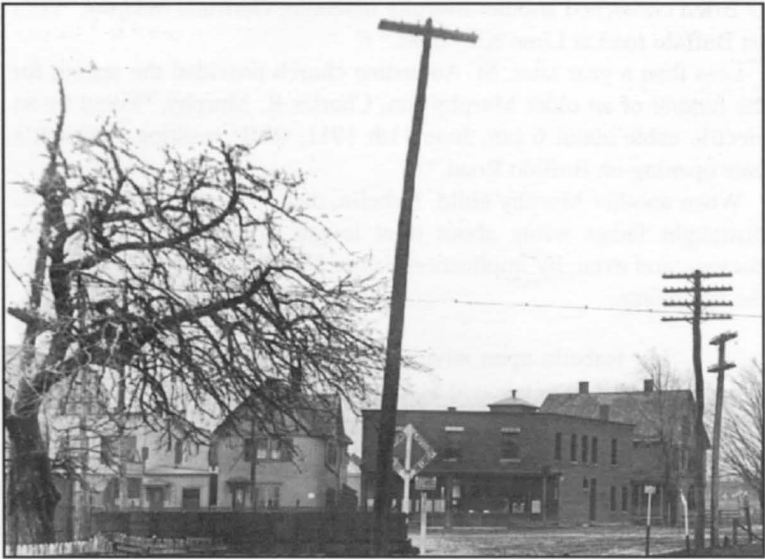
The Western end of West Avenue at Cairn Street was part of Lincoln Park, home of many immigrant and working class families. Railroad tracks made it a dangerous place for children to play. General Railway Signal, one of the Lincoln Park factories, is at right in this January 12, 1908 photograph. (From the Stone Negative Collection, Rochester Museum & Science Center.)
