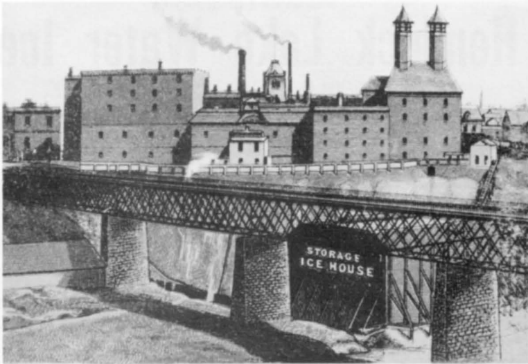
The Bartholomay Brewery Co. kept its ice below ground level to maintain coolness. Local History Division, Rochester Public Library.
