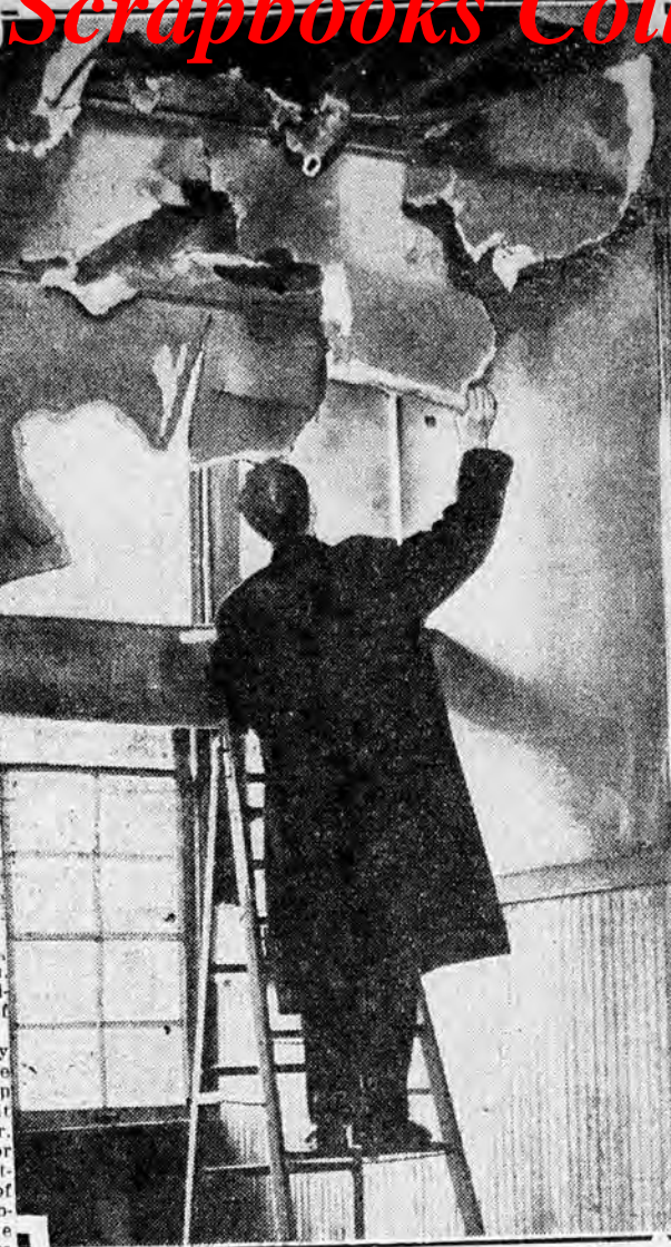
Paper composition partitions in the frame annex, shown above, led to the Fire Department condemnation of the school structure.
