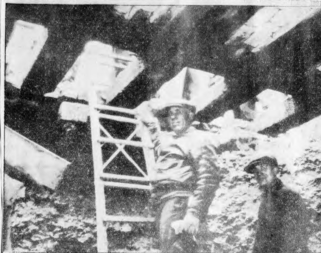
While bustling traffic roared overhead in the heart of Rochester, water was trickling—trickling—building catacombs under the pavement of Main Street for some hapless vehicle. But for the vigilance of a policeman, disaster probably would have resulted. Above is an interior view of the treacherous cavern, near the wall of the Genesee River. Joe Durnher, Times-Union photographer, took chances to set up his camera in the large hole. Below is Traffic Policeman Louis Ricey, who drove his motorcycle over a loose brick and immediately reported the menace. Beside him is Edwin A. Miller, city superintendent of maintenance, overseeing the repair job.
