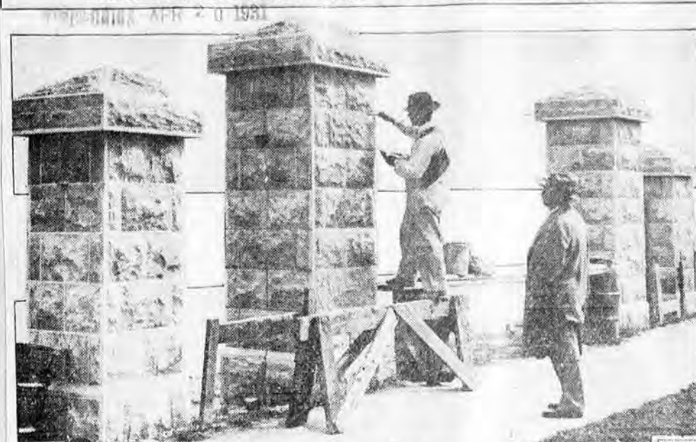
Stone piers at the Elmwood Avenue entrance to Mount Hope Cemetery were completed today when Frank Hamilton, mason, of 305 Hurstbourne Road, pointed the last bit of cement. He is seen giving the final touch. Each capstone topping the piers averages a ton in weight. Iron grills are to be hung by Wednesday, and the entrance opened to the public May 1.
