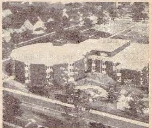
The new Lakeview School #7, Dewey Ave. at Bryan St., will open Fall 1968. Along with providing an exceptional educational opportunity, it will also offer superb recreational facilities for neighborhood children.
