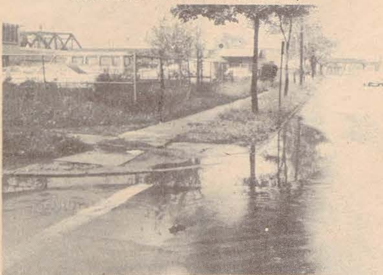
Flooded conditions at Wren and Driving Pk.
