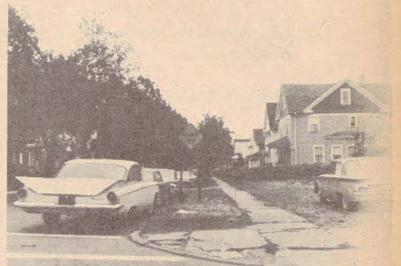
Broken sidewalks, Karnes & Otis Sts.
