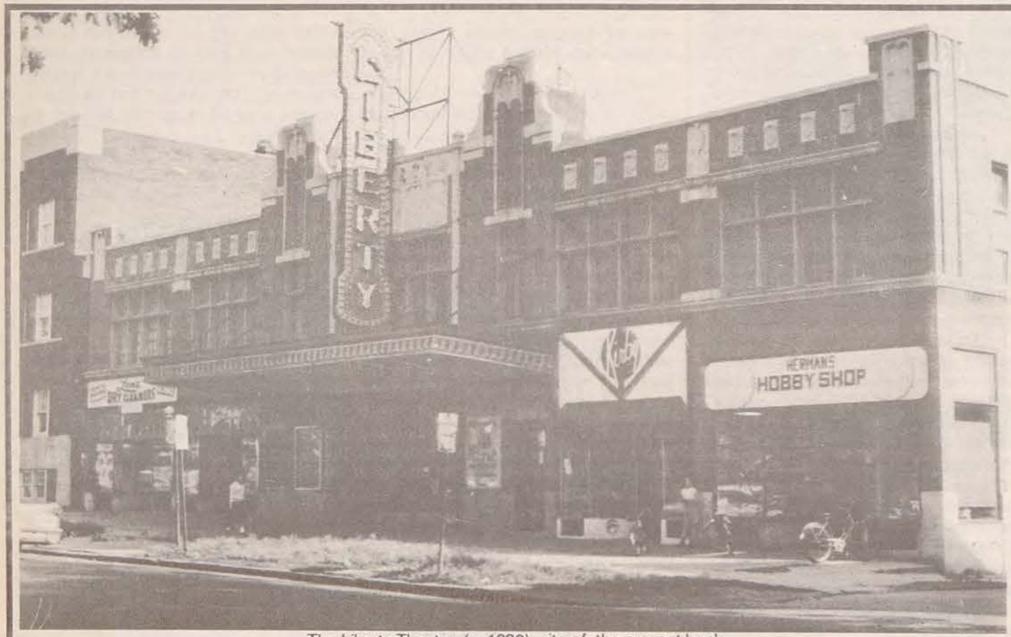
The Liberty Theater, (c. 1930), site of the present bank photo courtesy of Marine Midland Bank
