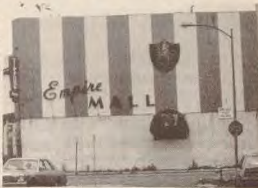
The front view of the Empire Mall building, at 266 Lyell Ave, which has remained vacant since a drug raid three years ago.
