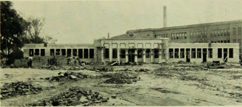
Cafeteria Building in Construction
