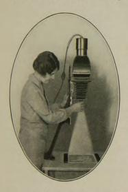
The enlarger focuses itself. As the camera is moved up or down to form an image of the desired size a camand-lever arrangement maintains the focus at critical sharpness. Enlarging with this outfit is therefore as rapid and easy as contact printing. And the Kodak Anastigmat lens supplied assures big prints that are professional in quality.
