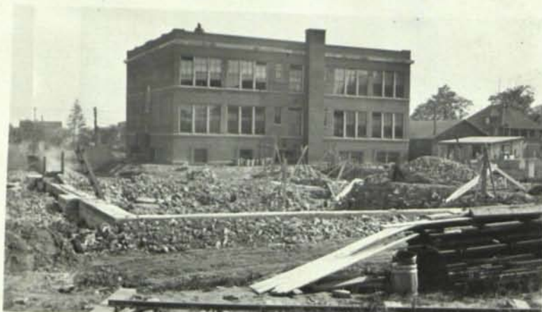
SCHOOL NO. 43 5/27/VI. SHOWING EXCAVATION AND FOUNDATION WALLS FOR ADDITION LOOKING NORTHEAST
