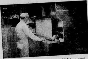
Total film output exceeded that of 1947 by a good margin. Here film is being coated with emulsion.
