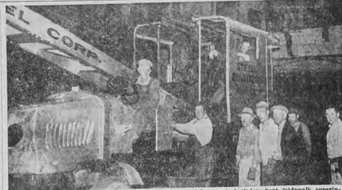
Here's the Crane Crew whose dextrous manipulations of heavy steel girders kept "sidewalk superintendents" goggle eyed during bridge construction. They were part of volunteer union labor which erected entire structure.
