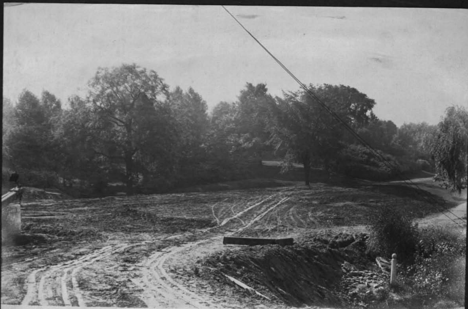
11450 South approach to Elmwood Ave bridge looking south Cont 59 Sept 14 1917
