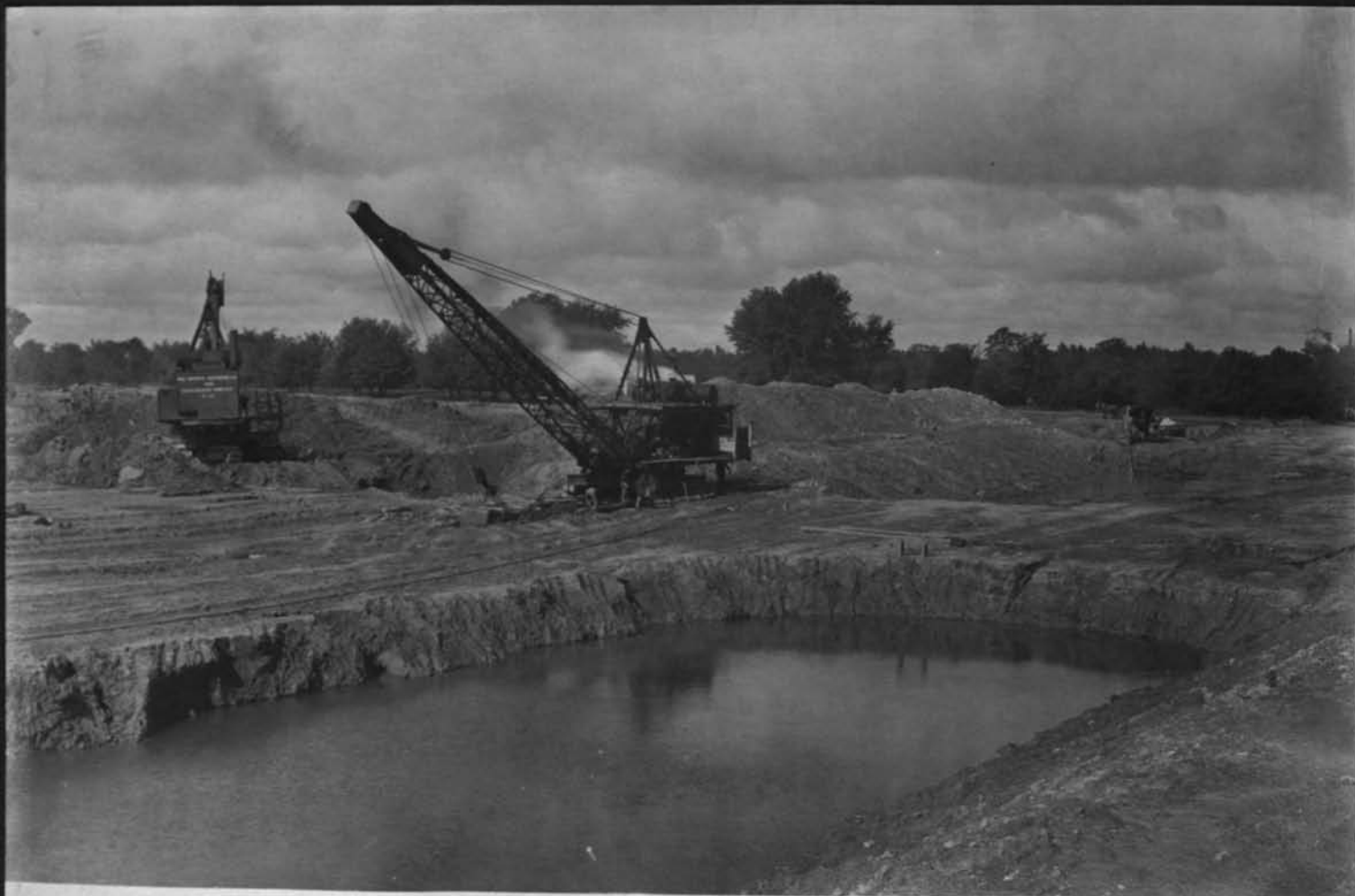
11442 Looking S W toward site of west foot bridge South Park Cont 59 Sept 10 1917
