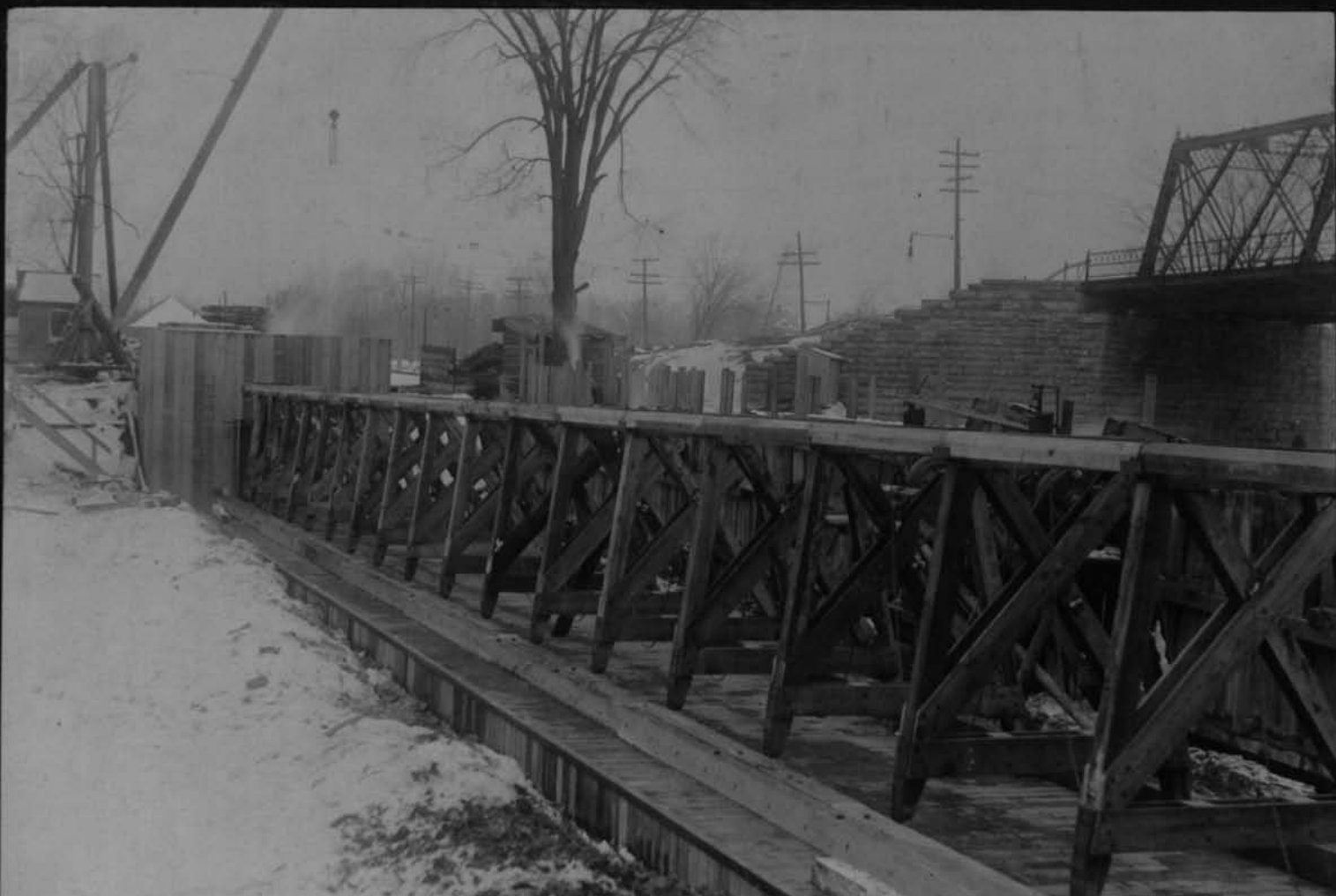
11593 "A" frames in temporary dam erected Cont 59 Poiré's dam
