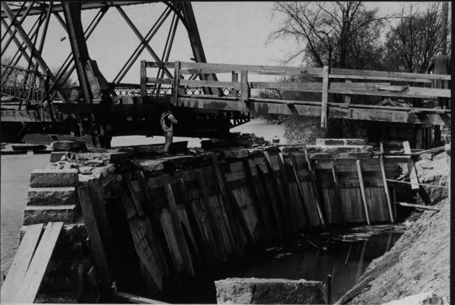
11296 East abutment Elmwood Ave. bridge. Cont. 59. May 14, 1917.
