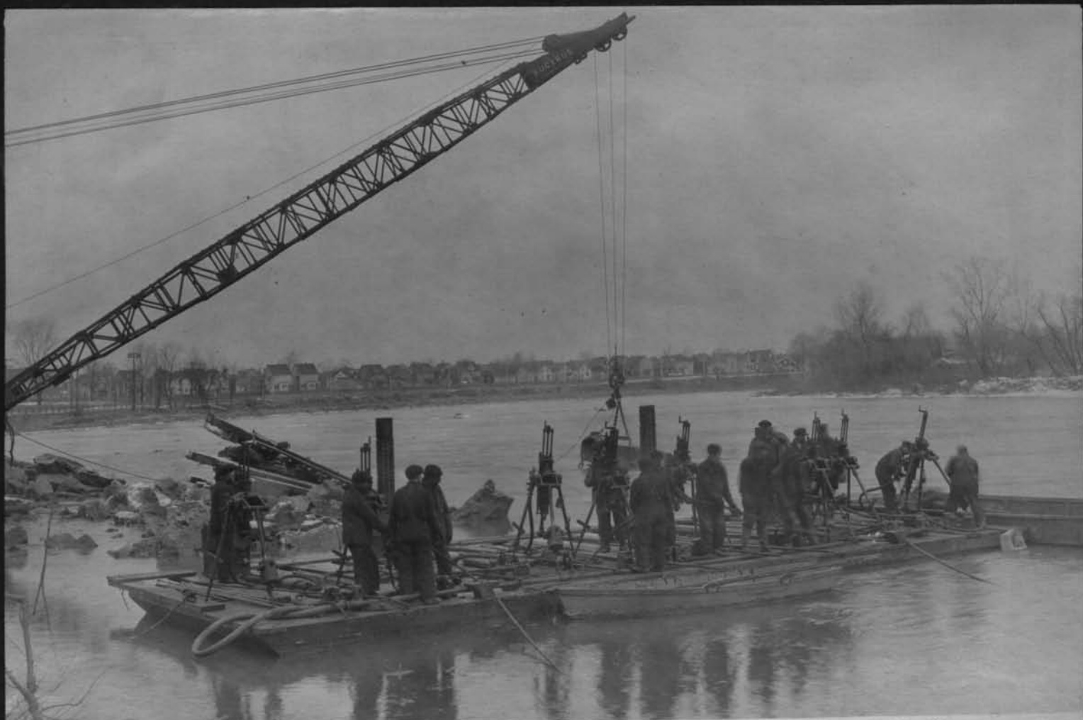
11573 Drill-boats preceding drag-line at Plymouth Ave South Park Cont 59 Dec 5 1917
