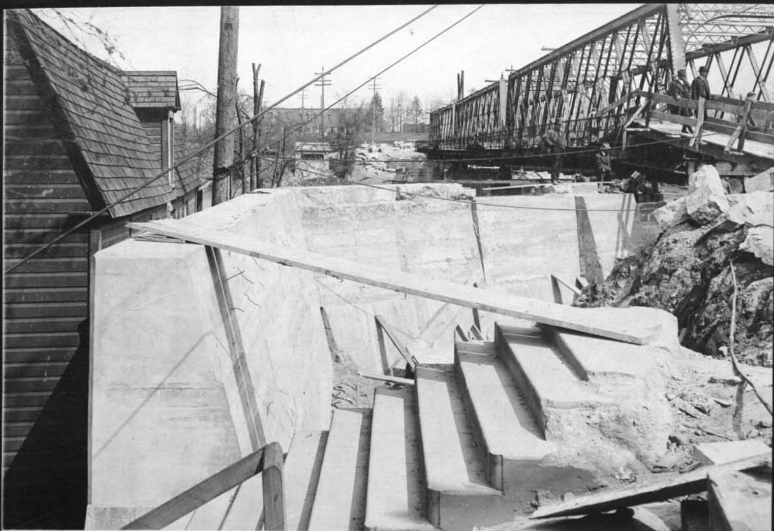
11294 North wing of west abutment Elmwood Ave. bridge. Cont. 59. May 14, 1917.
