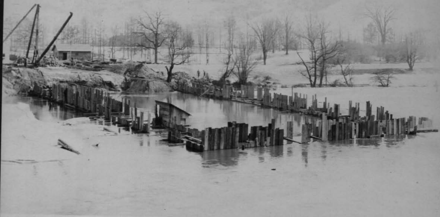
11646 Temporary dam at high water Looking east from Elmwood Ave bridge Cont 59 Feb 13 1918
