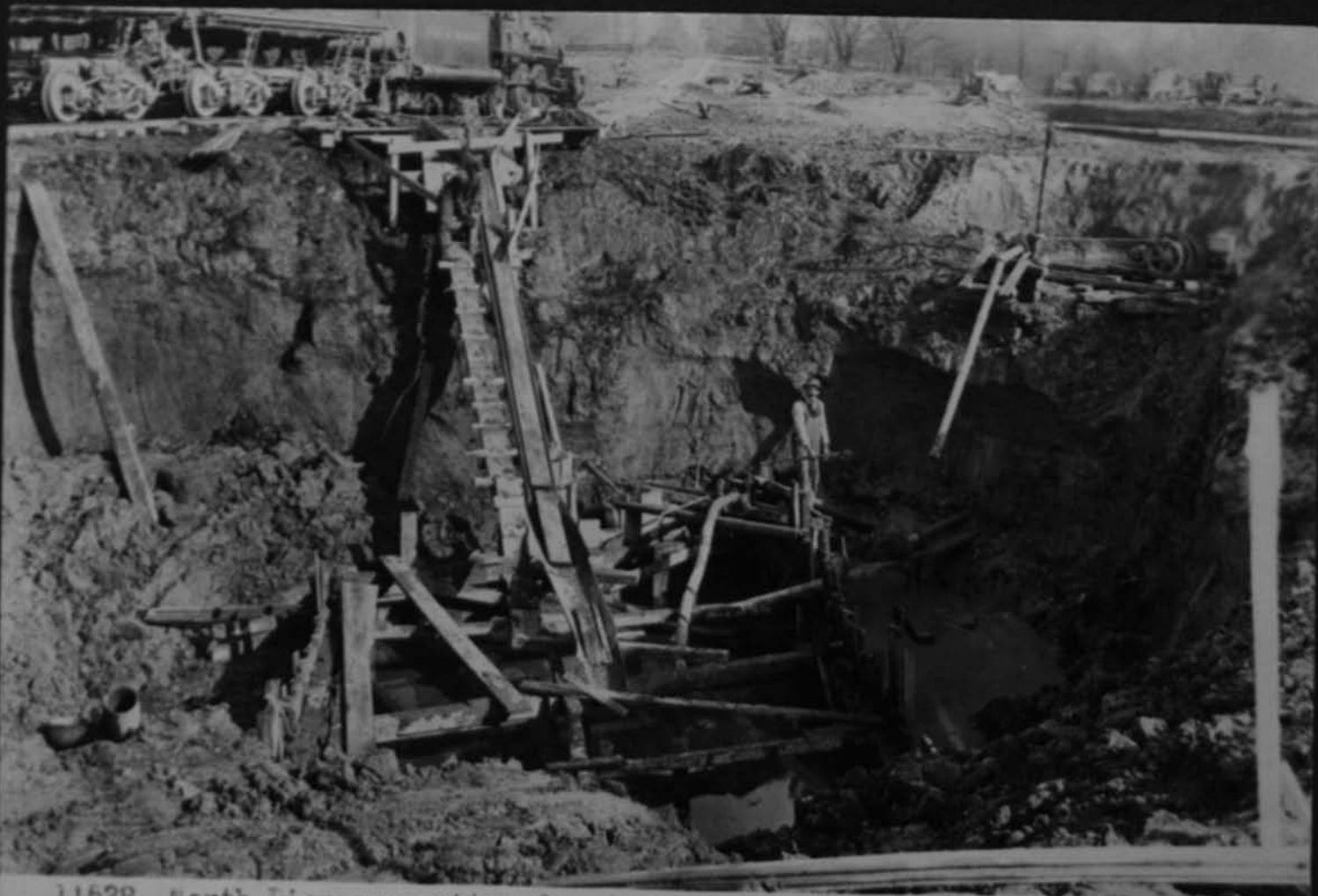
11538 North Pier excavation for foot bridge West side of Genesee Cont 59 Nov 13 1917
