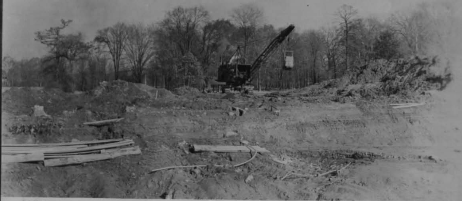
11535 Dregline near Red Creek Looking north Cont 59 Nov 5 1917
