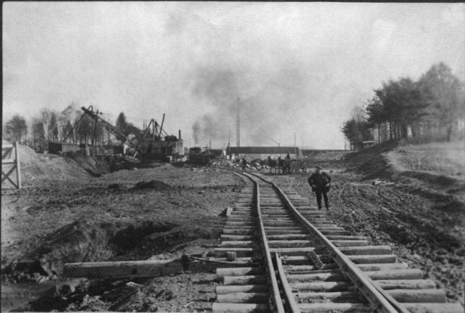
11533 Dragline near site of old Main Road Looking east Cont 59 Nov 5 1917
