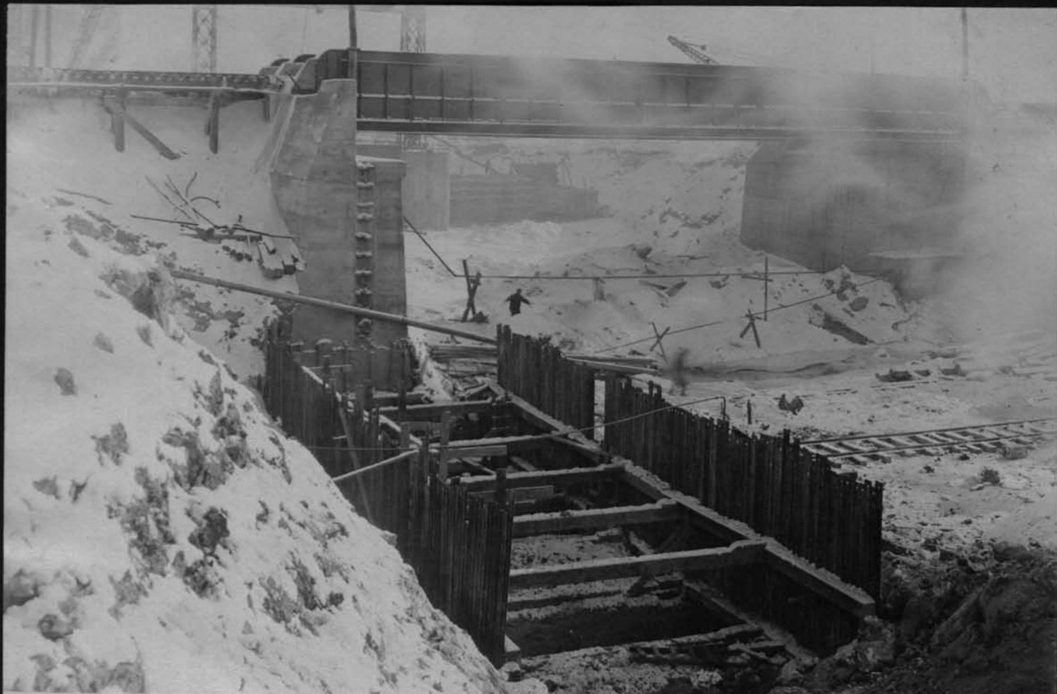
11627 Excavation for north pier for Erie R R crossing Looking east Cont 59 Jan 4 1918
