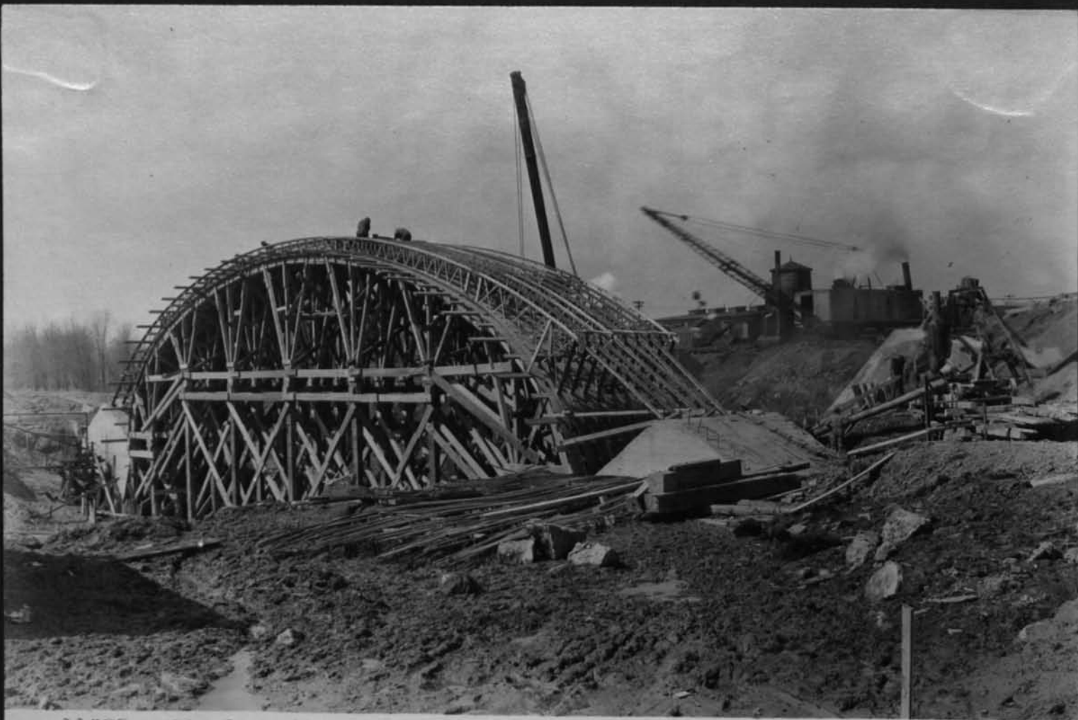
11685 Steel work and centering on Foot Bridge west side of Genesee Cont 59 March 28 1918
