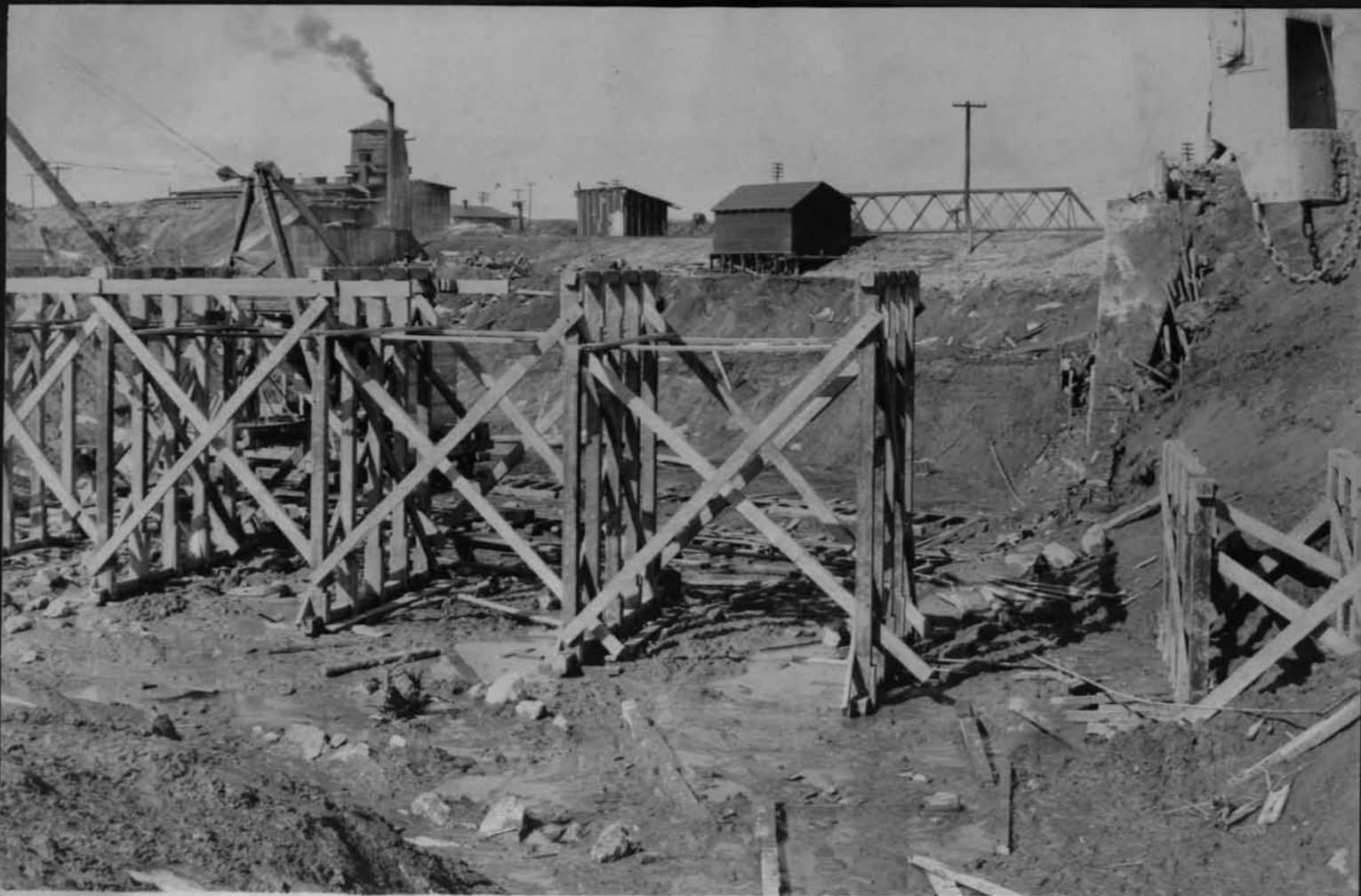
11671 Abutments for Penna crossing and centering for foot bridge Cont 59 March 13 1918
