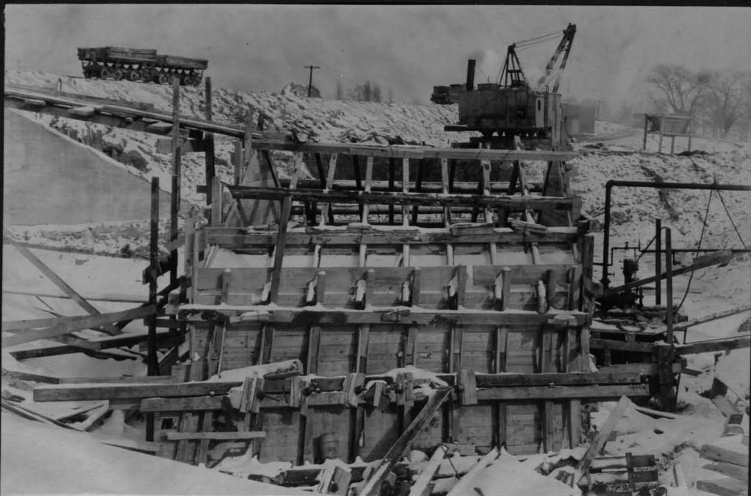
11635 South abutment for foot-bridge on west side of Genesee Looking N Cont 59 Jan 25 1918
