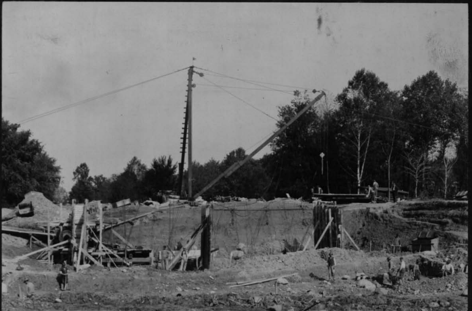
11517 Forms for north abutment Main drive bridge South Park Cont 59 Oct 17 1917
