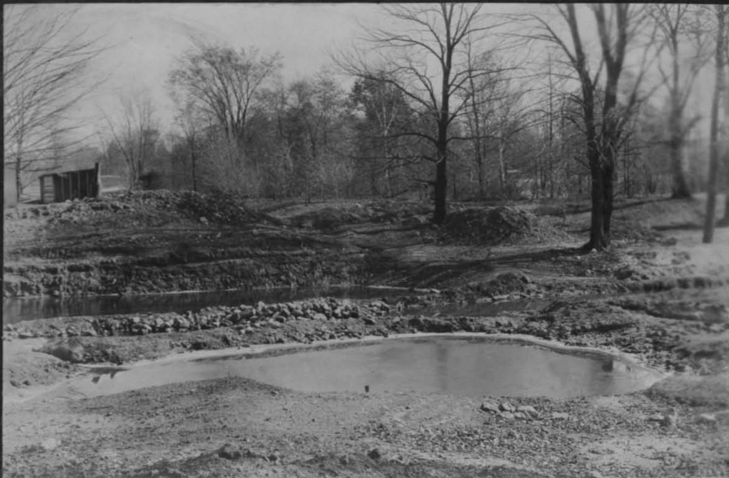
11542 Excavation on upper bridge site Looking east Cont 144 Nov 5 1917
