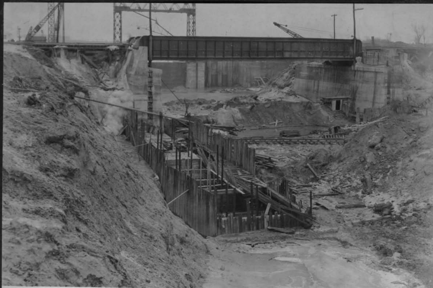
11643 North abutment for Erie R R crossing Cont 59
