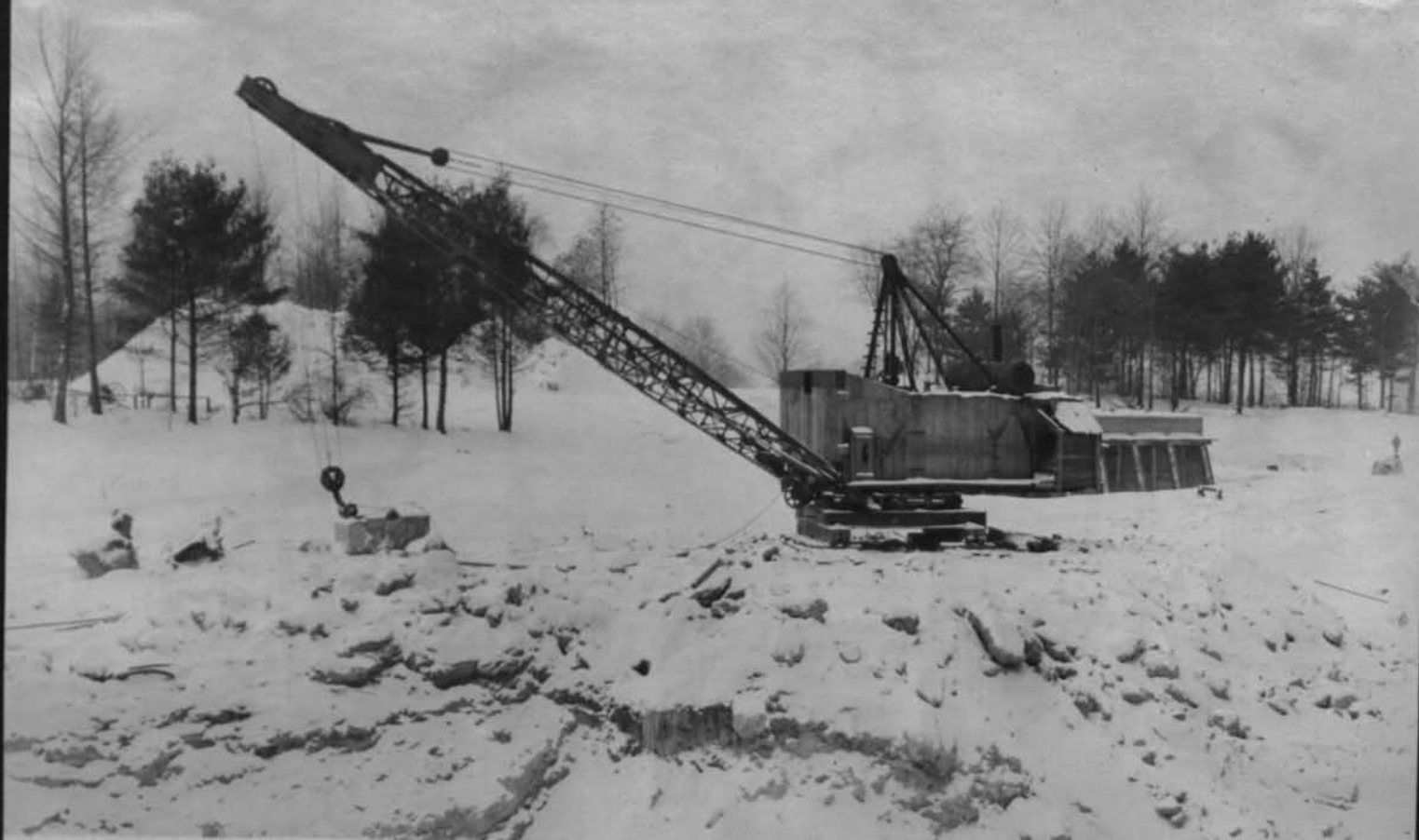
11632 Drag-line laid up just west of Erie R R crossing Looking south Cont 59 Jan 25 1918
