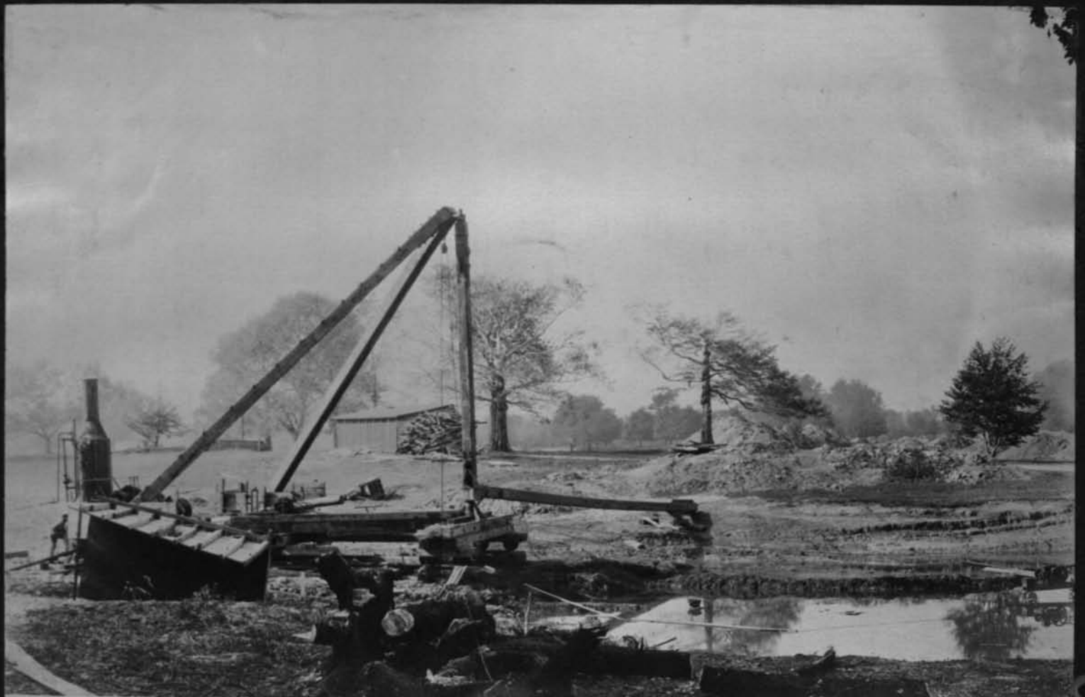
11503 Derrick on north bridge site South Park Cont 144 Oct 17 1917
