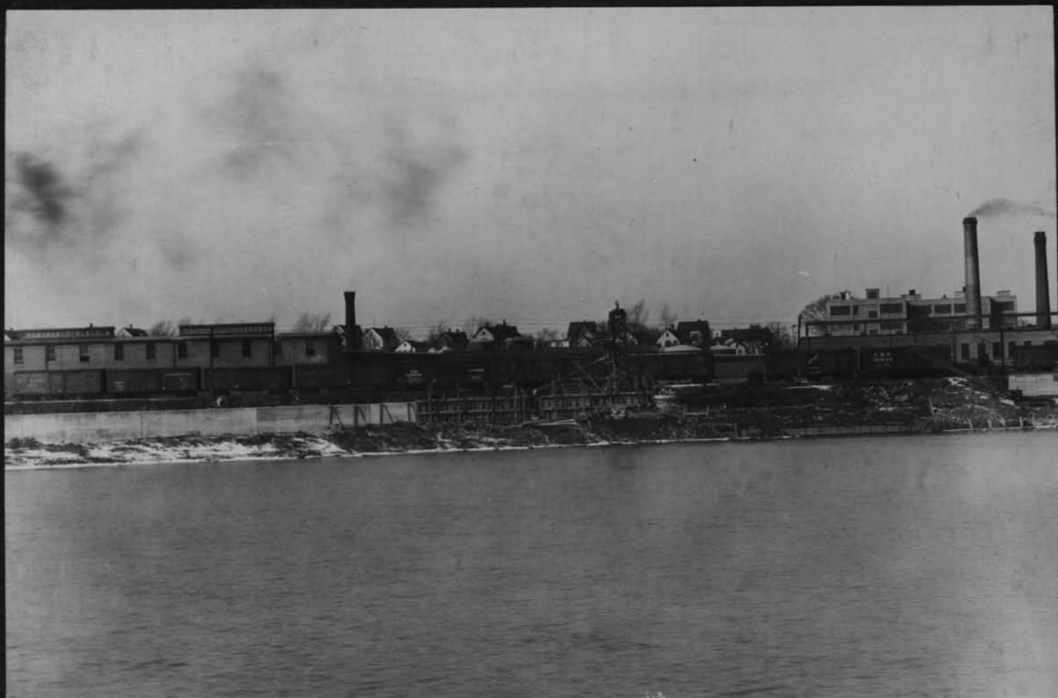
11572 River wall north of Erie Bridge Looking west Cont 59 Dec 5 1917
