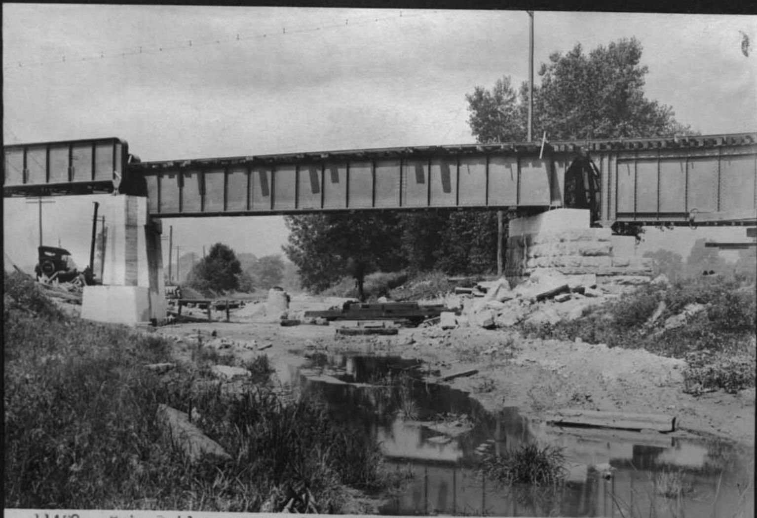
11408 Erie Bridge over feeder Looking west Cont 59 Aug 7 1917
