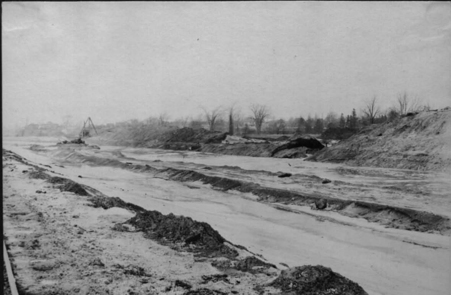
11645 Break in Spoil bank on N side of canal at Red Creek Cont 59 Feb 13 1918
