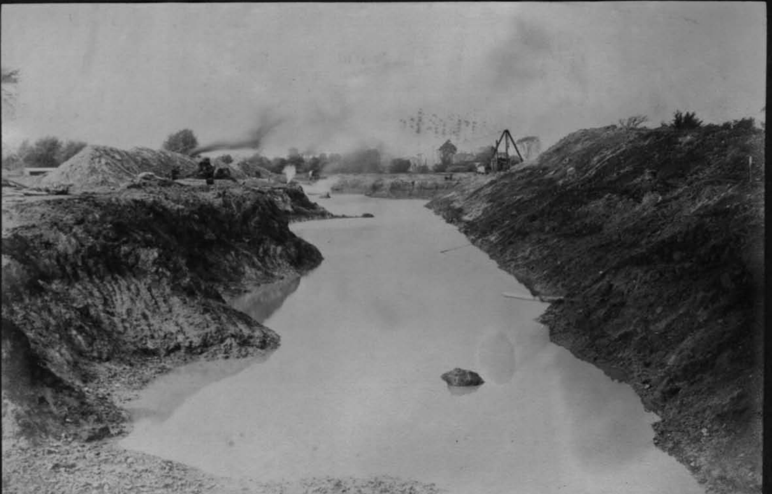
11518 Prism excavation west from Red Creek Cont 59 Oct 17 1917
