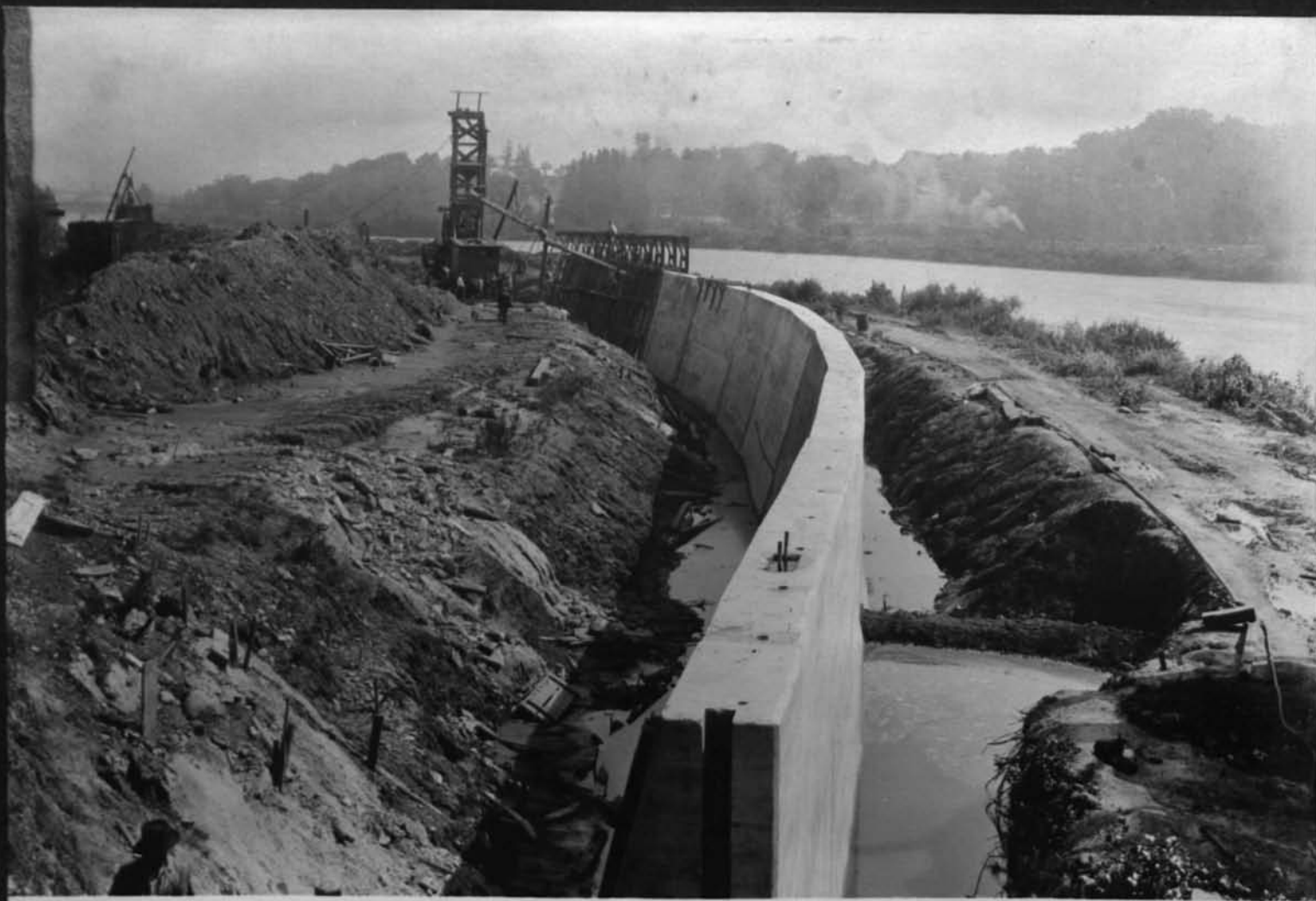
11412 River wall near Erie Bridge Looking north Cont 59 Aug 19 1917
