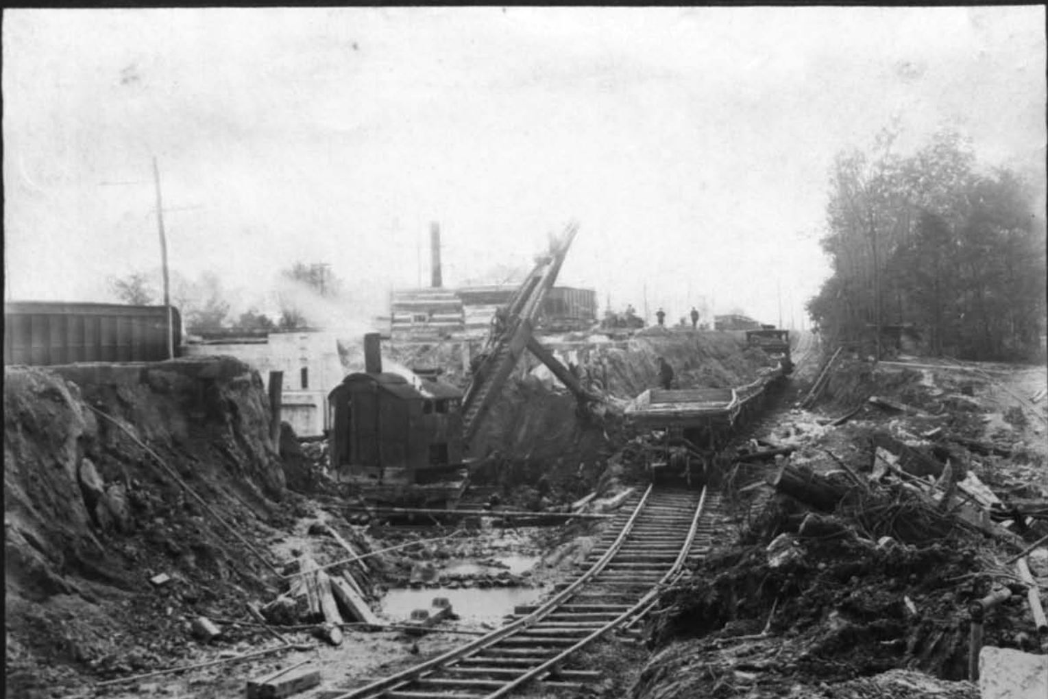
11515 Excavation for Erie crossing Looking south Cont 59 Oct 16 1917
