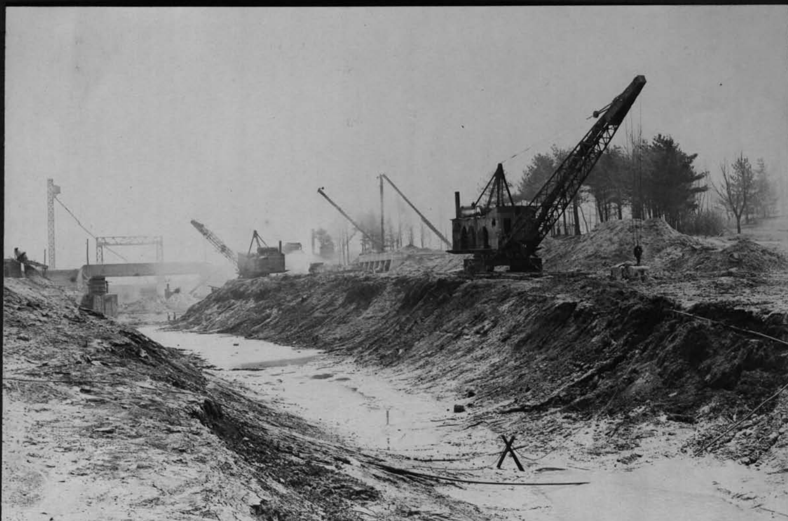
11725 Looking east toward Erie R R crossing South Park Cont 59 April 15 1918
