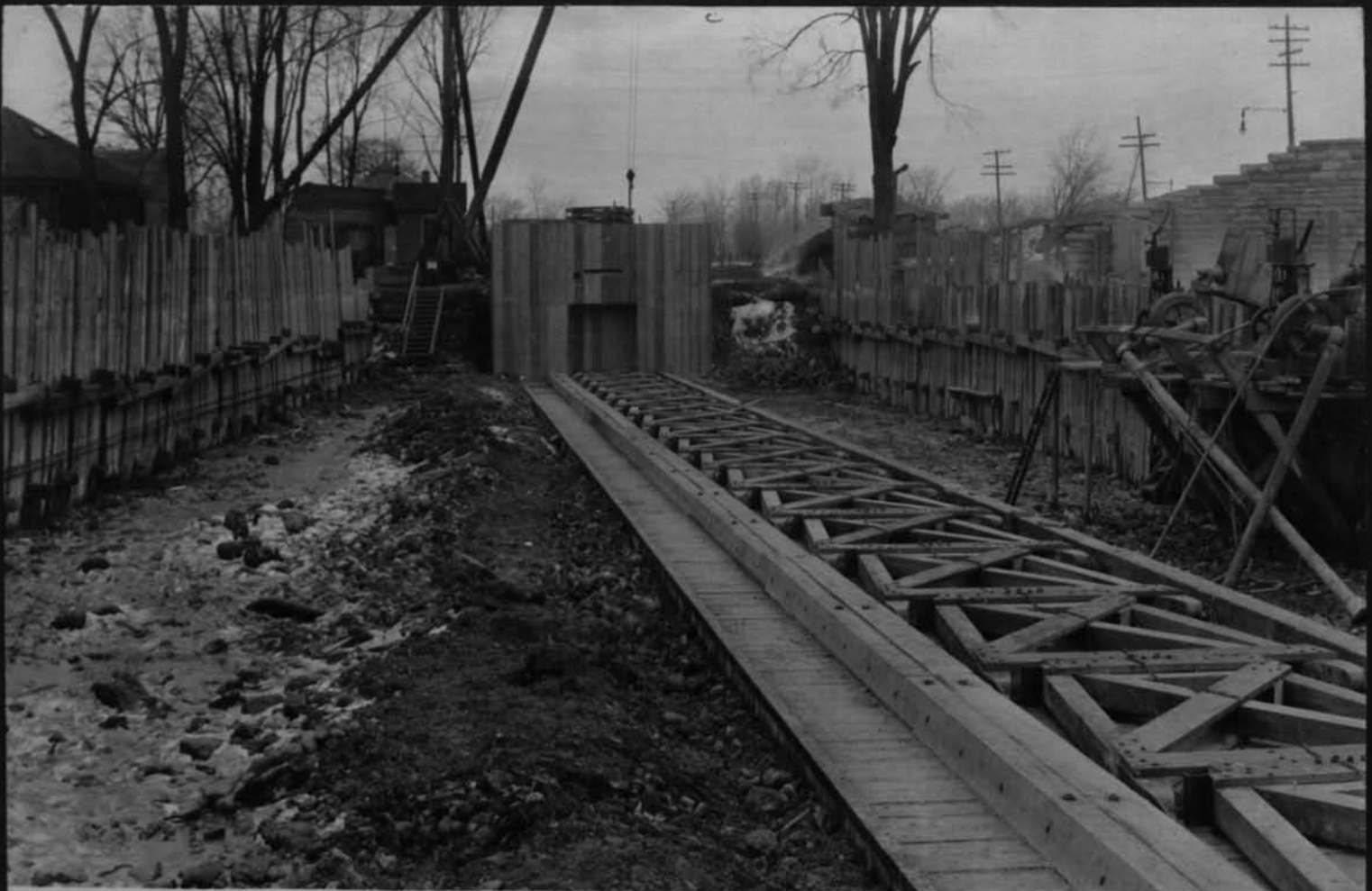
11592 "A" frames in temporary dam laying down Looking west Cont 59 Dec 24 1917
