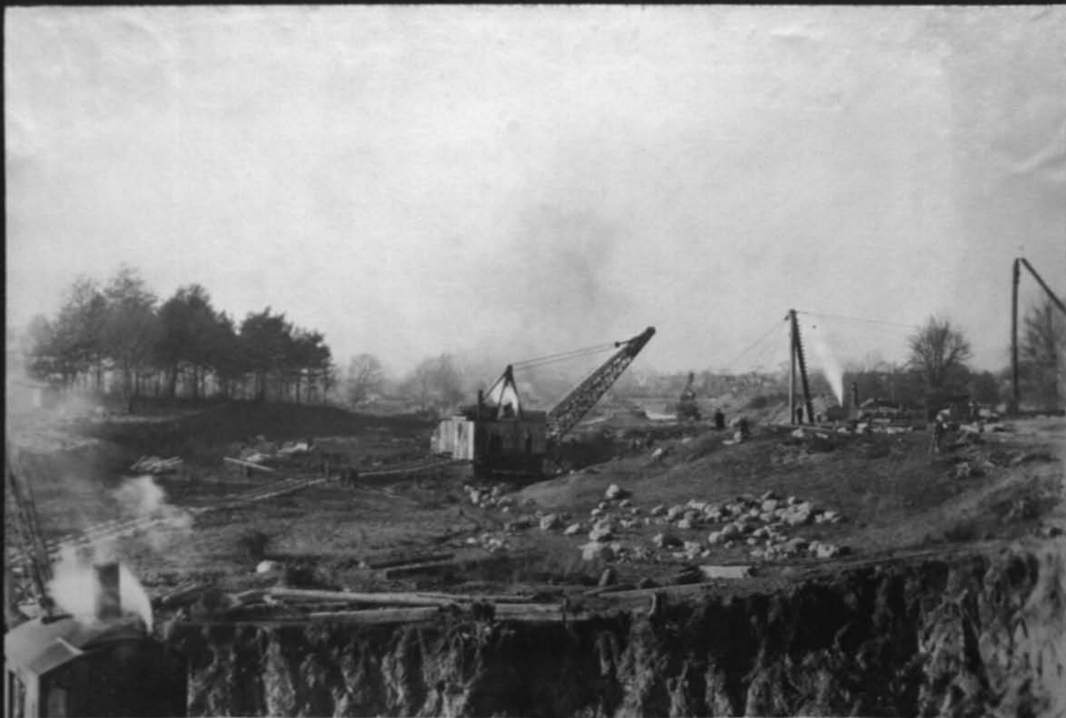
11540 Looking west from Erie Bridge toward Genesee Cont 59 Nov 13 1917
