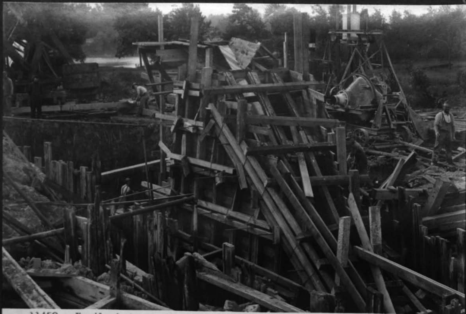
11459 North abutment for Penna crossing Cont 59 Sept 21 1917
