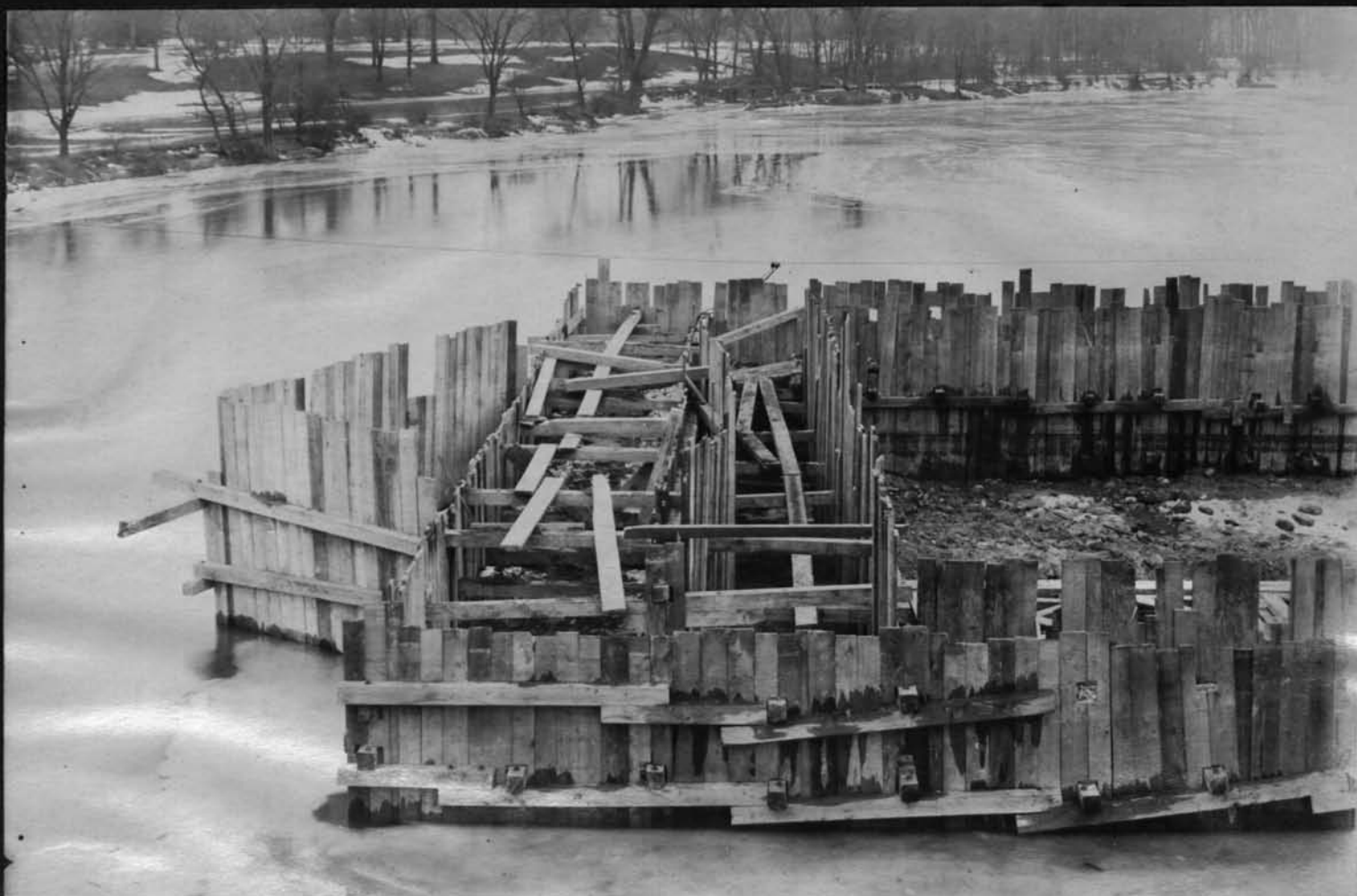
11594 Bulk-heads in east end of coffer-dam at Elmwood Ave bridge Cont 59
