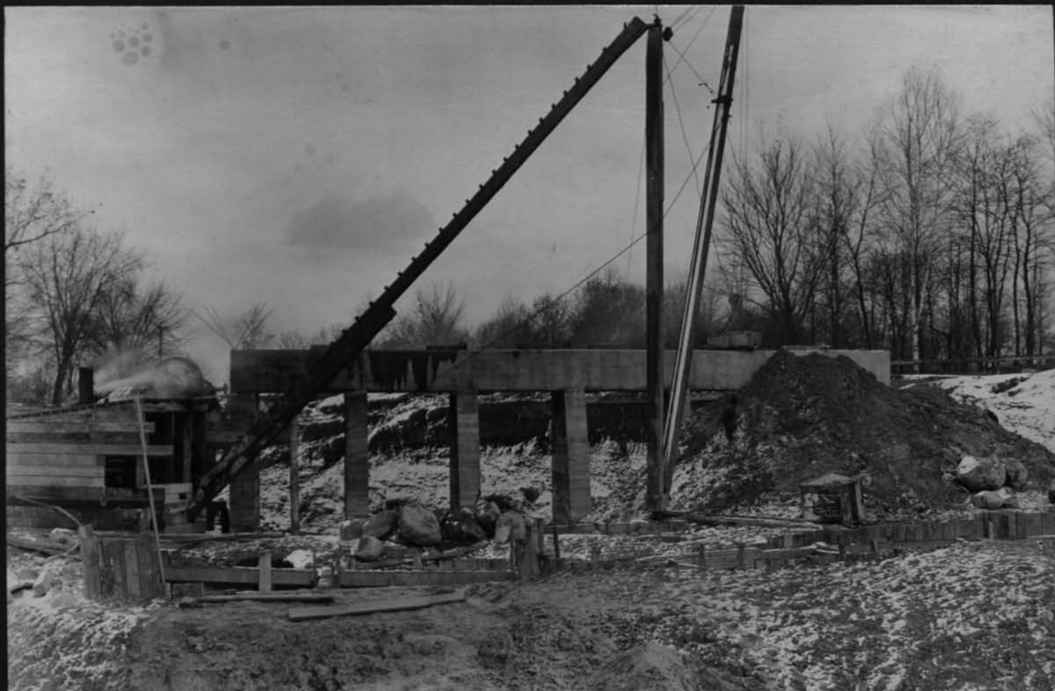
11575 North abutment for Main drive bridge South Park Cont 59 Dec 5 1917
