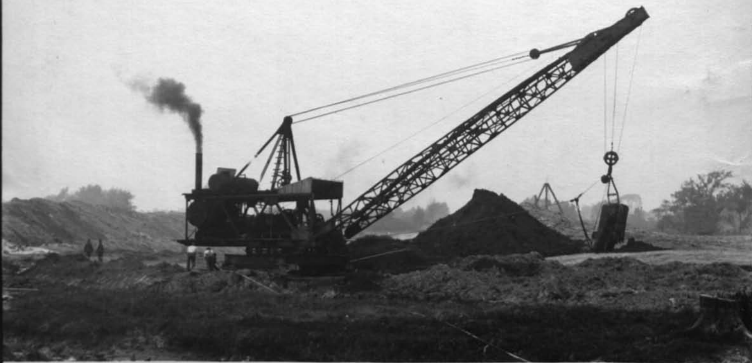
11455 Drag line just west of Red Creek in South Park Cont 59 Sept 20 1917
