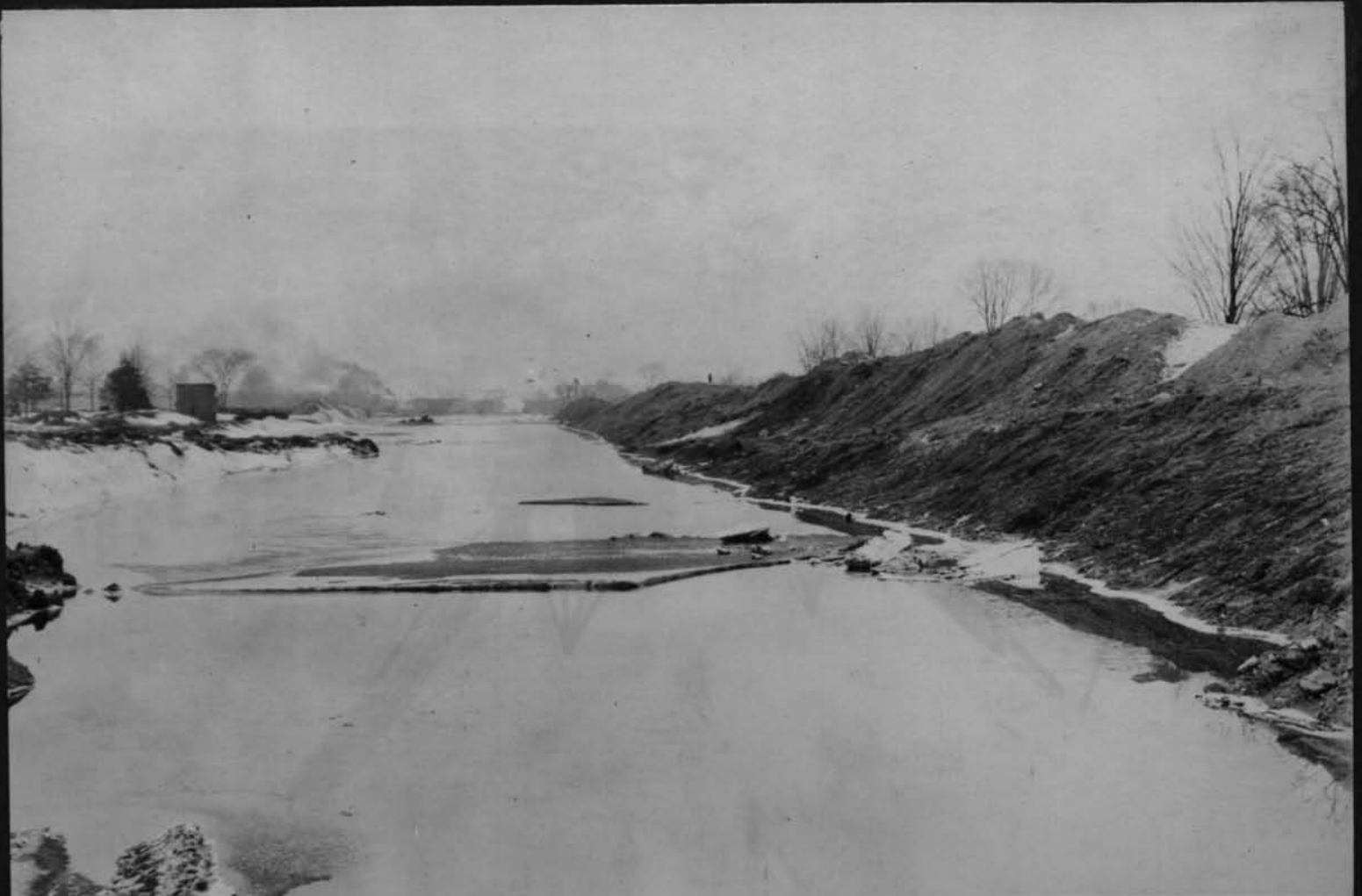
11649 Looking west from Main drive bridge during high water Cont 59 Feb 14 1918
