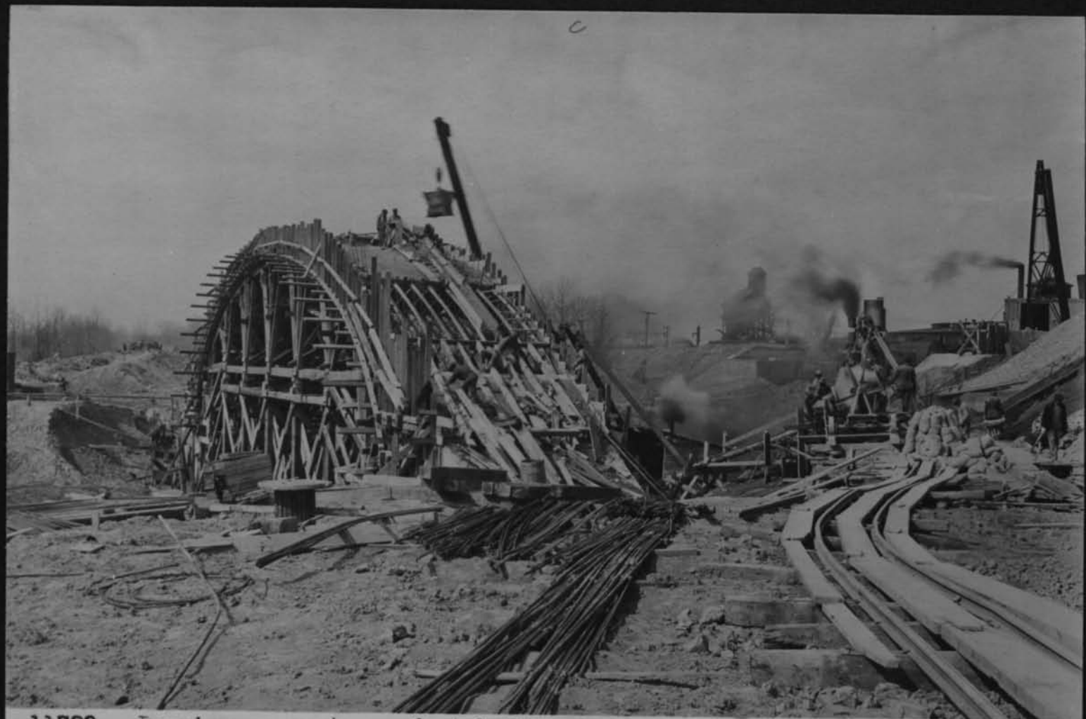
11723 Pouring concrete on foot-bridge W side of Genesee Looking S Cont 59 April 10 1918
