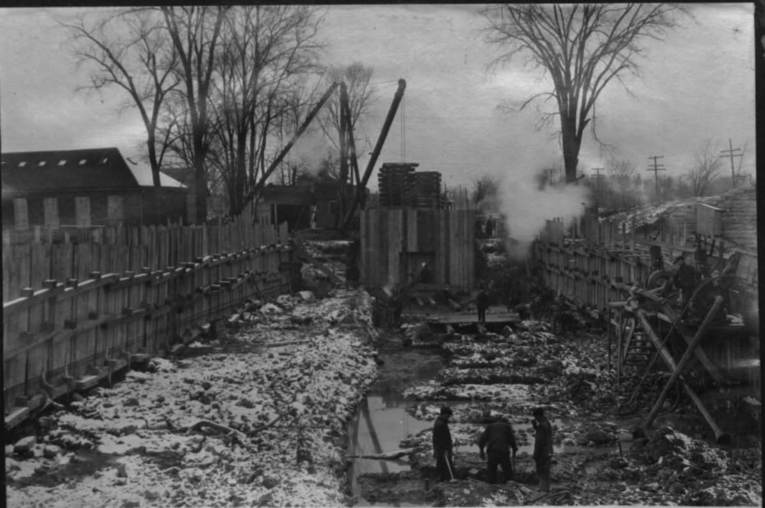
11591 Laying foundation for temporary dam at Elmwood Ave bridge Cont 59 Looking west Dec 18 1917
