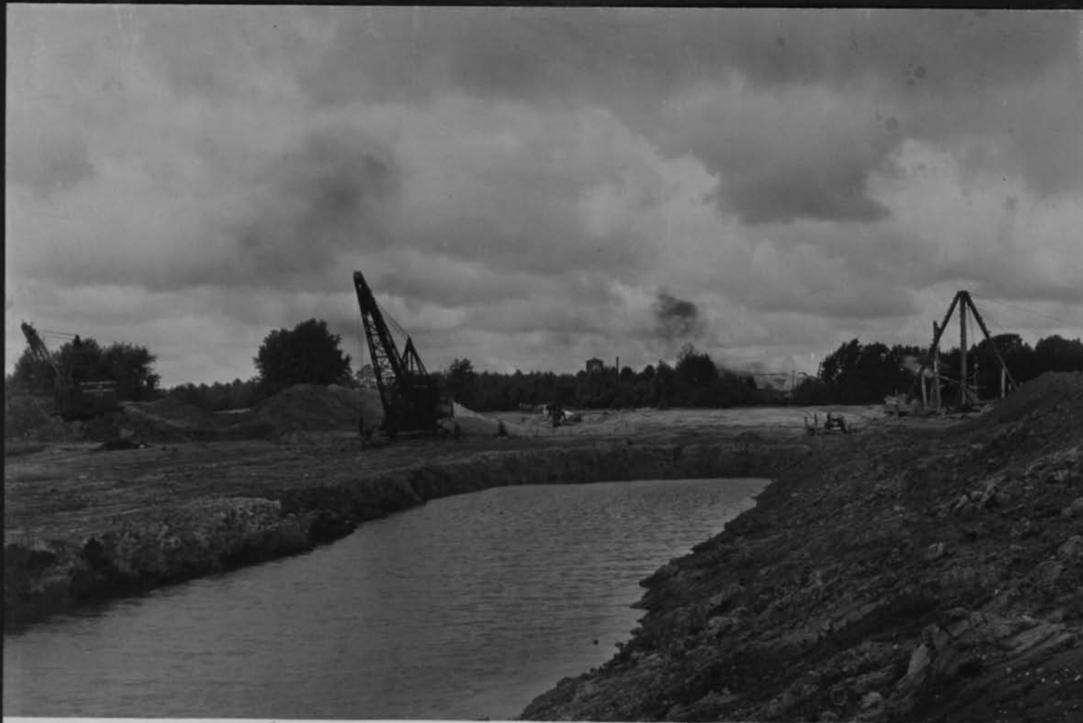
11441 Prism excavation looking toward river in South Park Cont 59 Sept 10 1917
