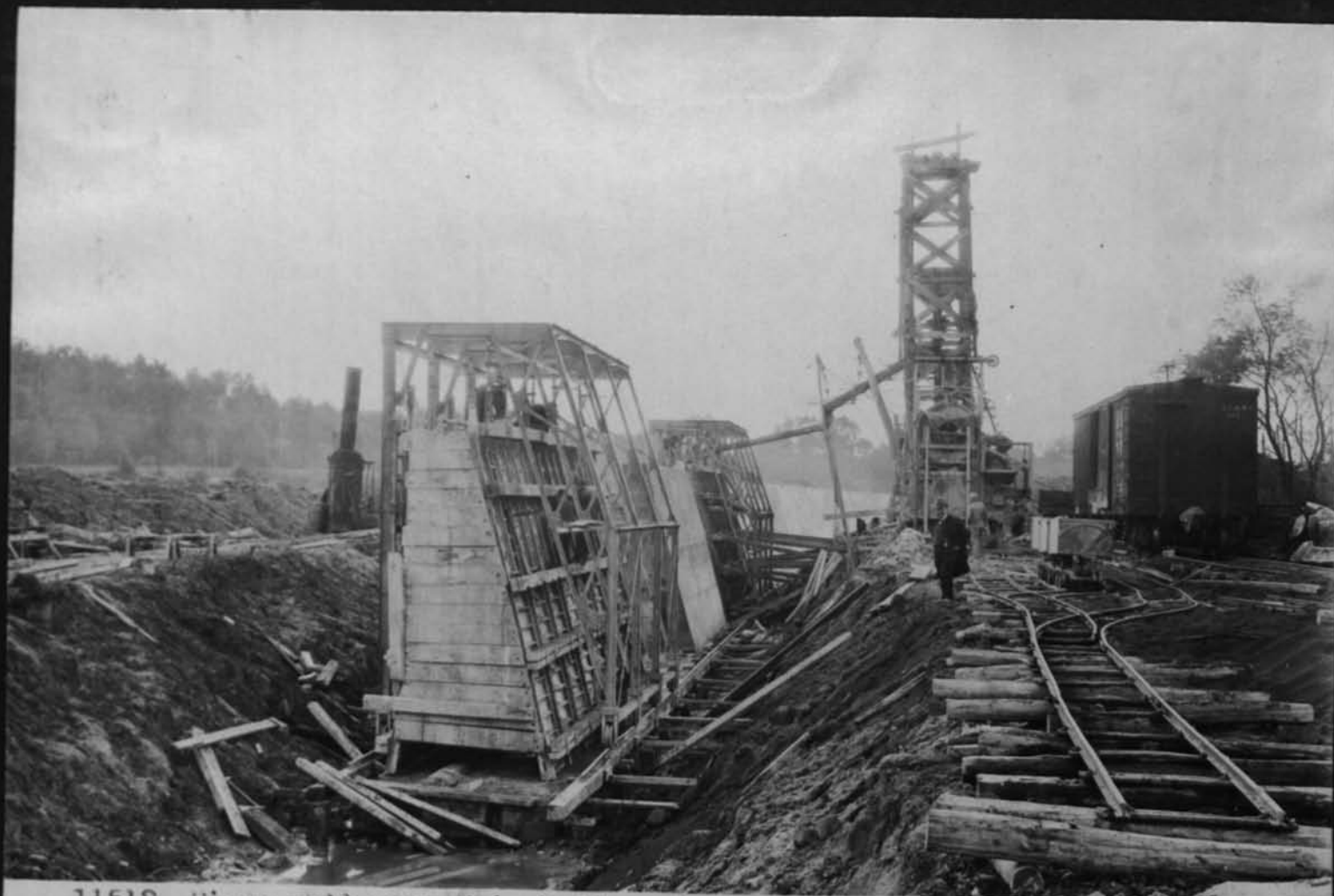
11512 River wall near Erie bridge Looking south Cont 59 Oct 16 1917
