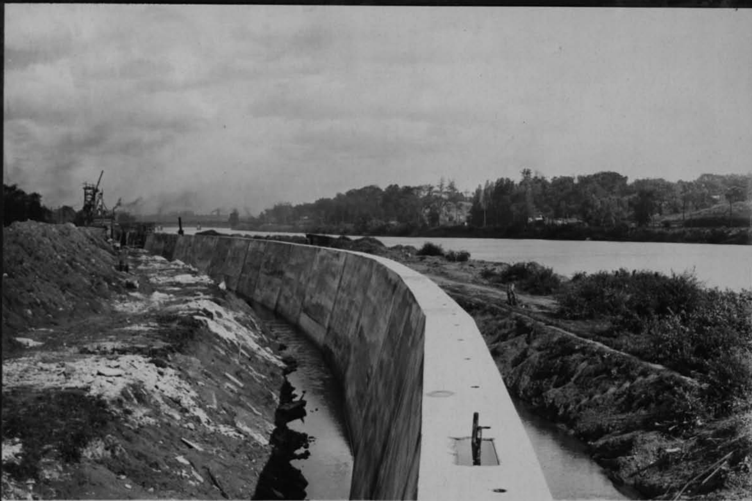
11513 River wall near Erie bridge Looking north Cont 59 Oct 16 1917
