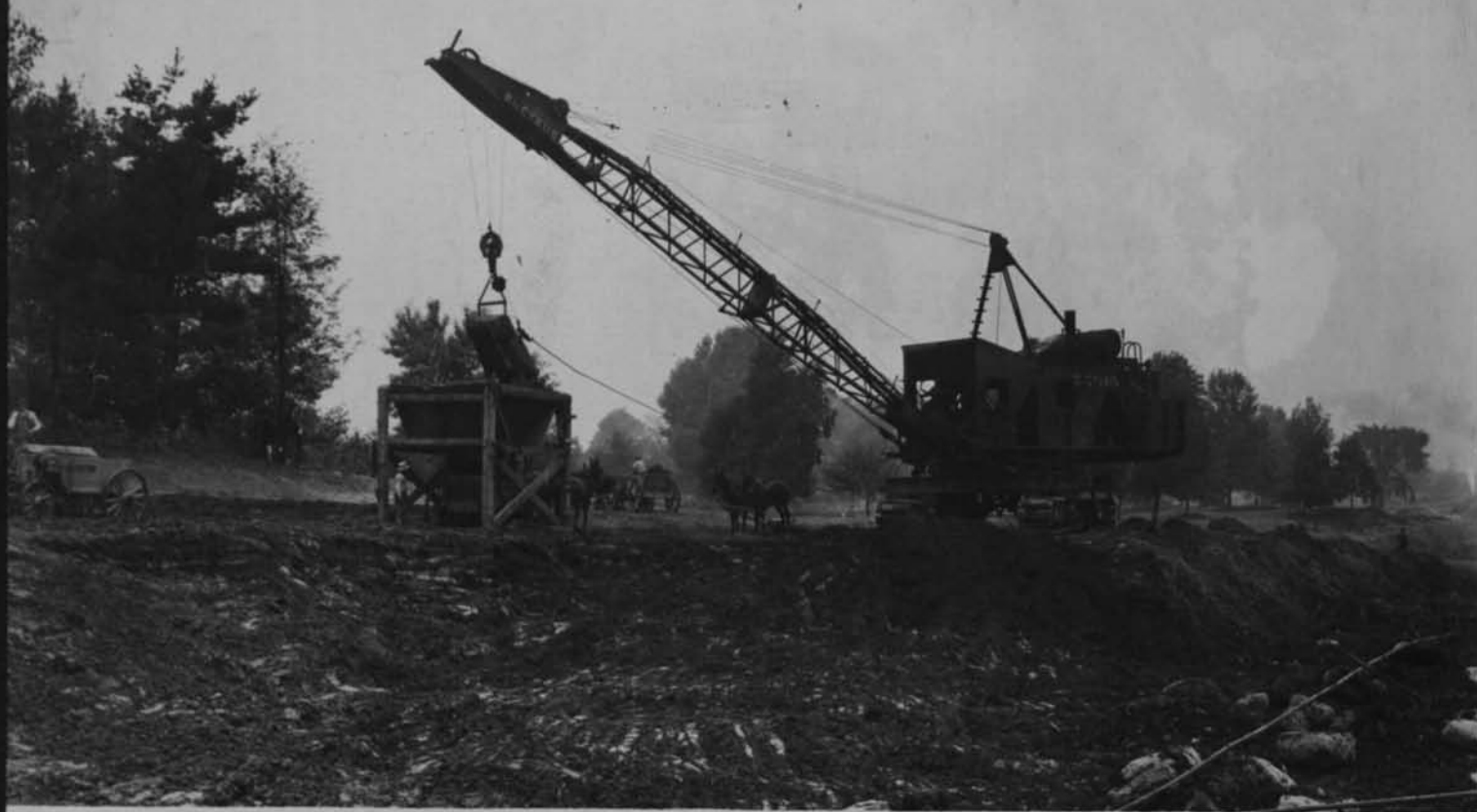
11453 Drag line on site of old main road in South Park Cont 59 Sept 20 1917
