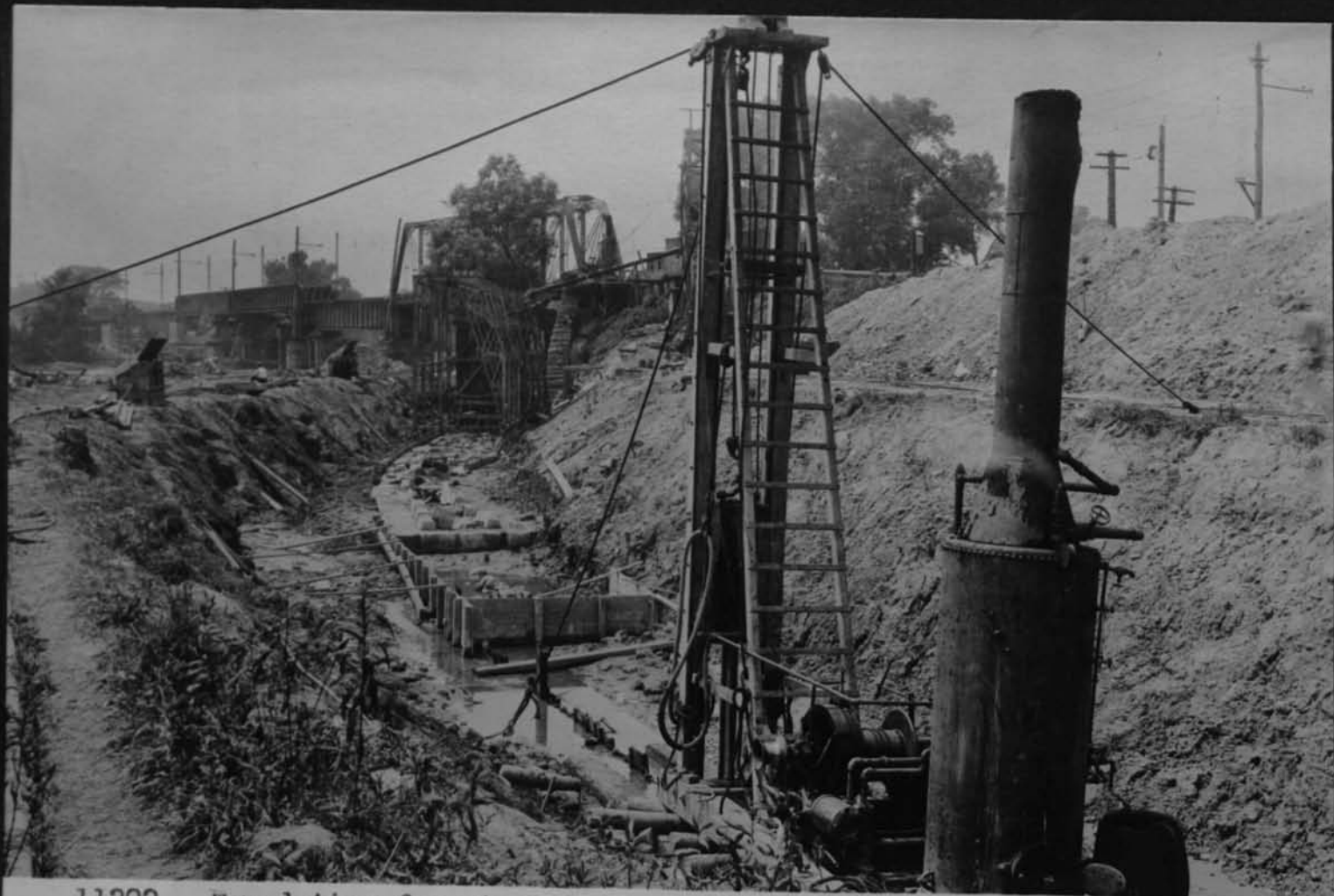
11393 Foundation for river wall near Erie bridge Cont 59 July 24 1917
