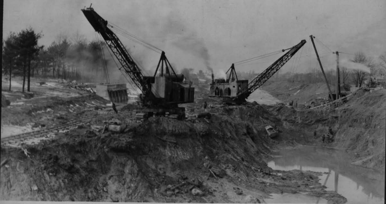
11670 Dragline operating west of Erie crossing Looking west Cont 59 March 13 1918
