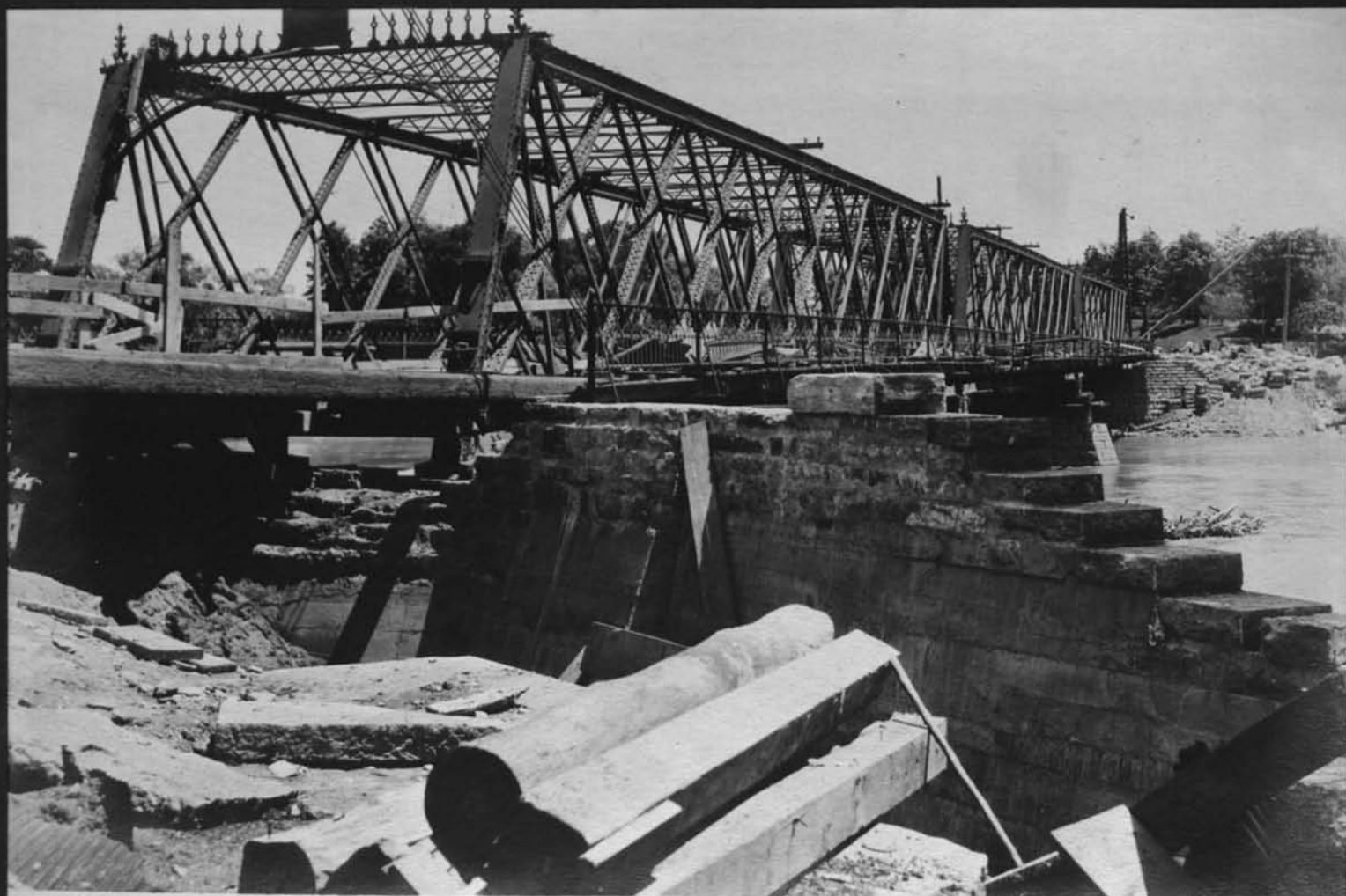
11328 West pier Elmwood Ave bridge looking east Cont 59 June 25 1917
