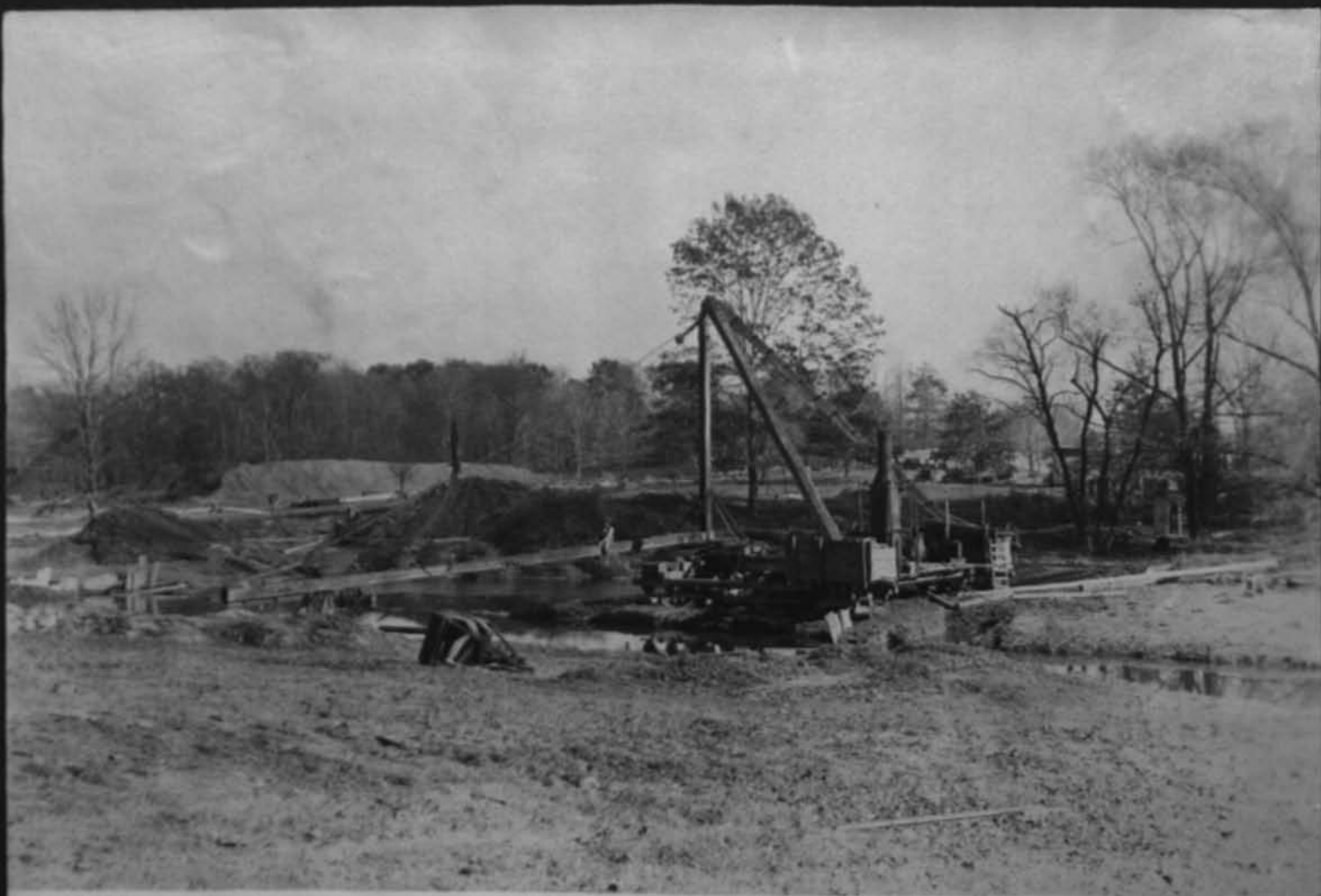
11541 Equipment for lower bridge construction Looking north Cont 144 Nov 5 1917
