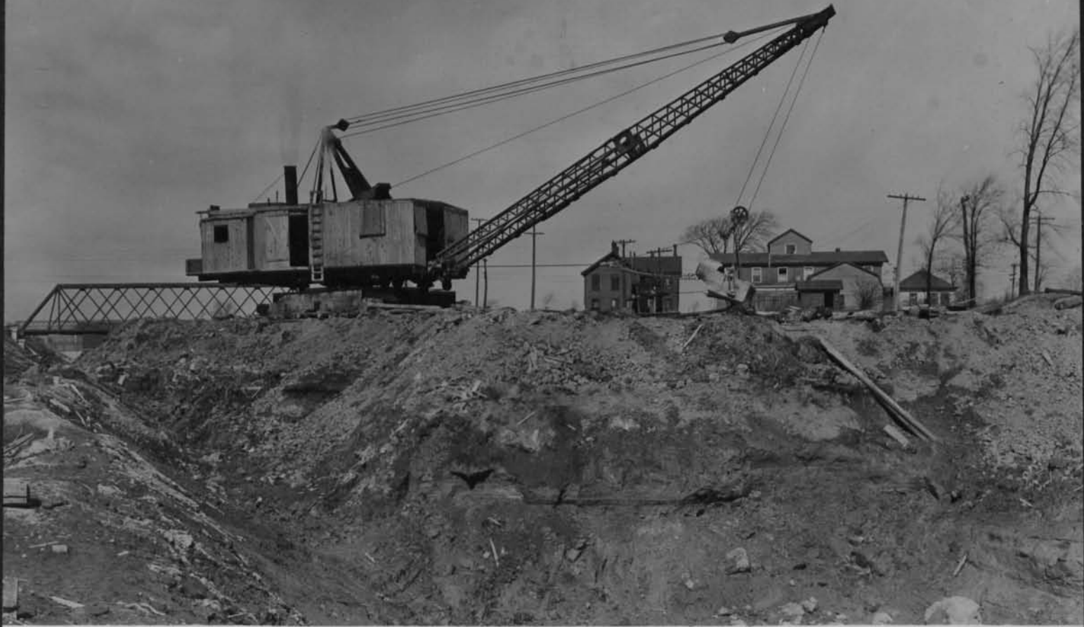
11686 Drag line operating on west side of Genesee at Penna crossing Cont 59 March 28 1918
