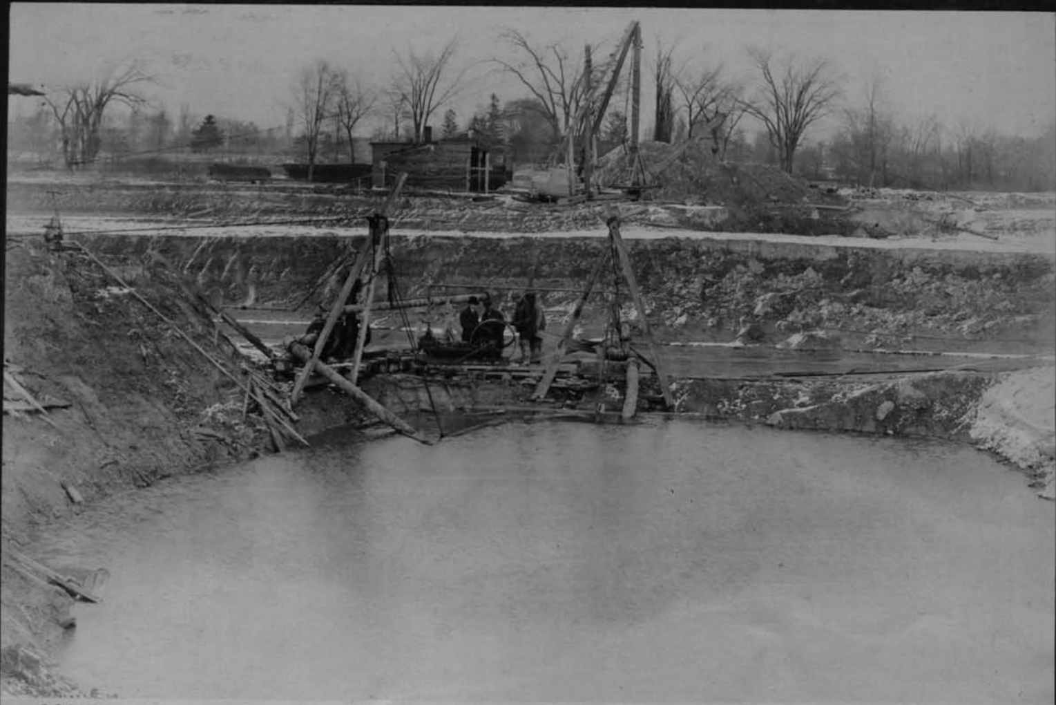
11576 Excavation for west foot-bridge east side of Genesee Looking N Cont 59 Dec 5 1917
