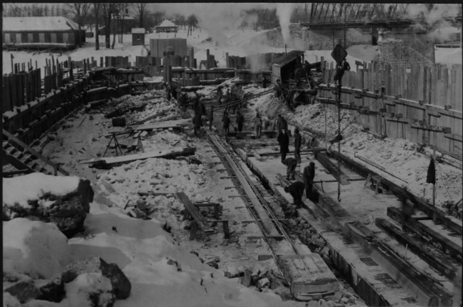
11641 Construction on temporary dam at Elmwood Ave bridge Looking west Cont 59 Feb 8 1918
