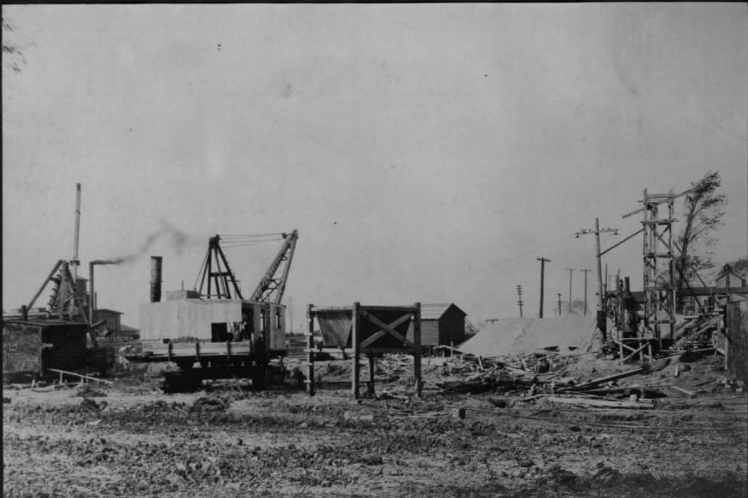
11523 Equipment on west bank of Genesee Looking west Cont 59 Oct 18 1917
