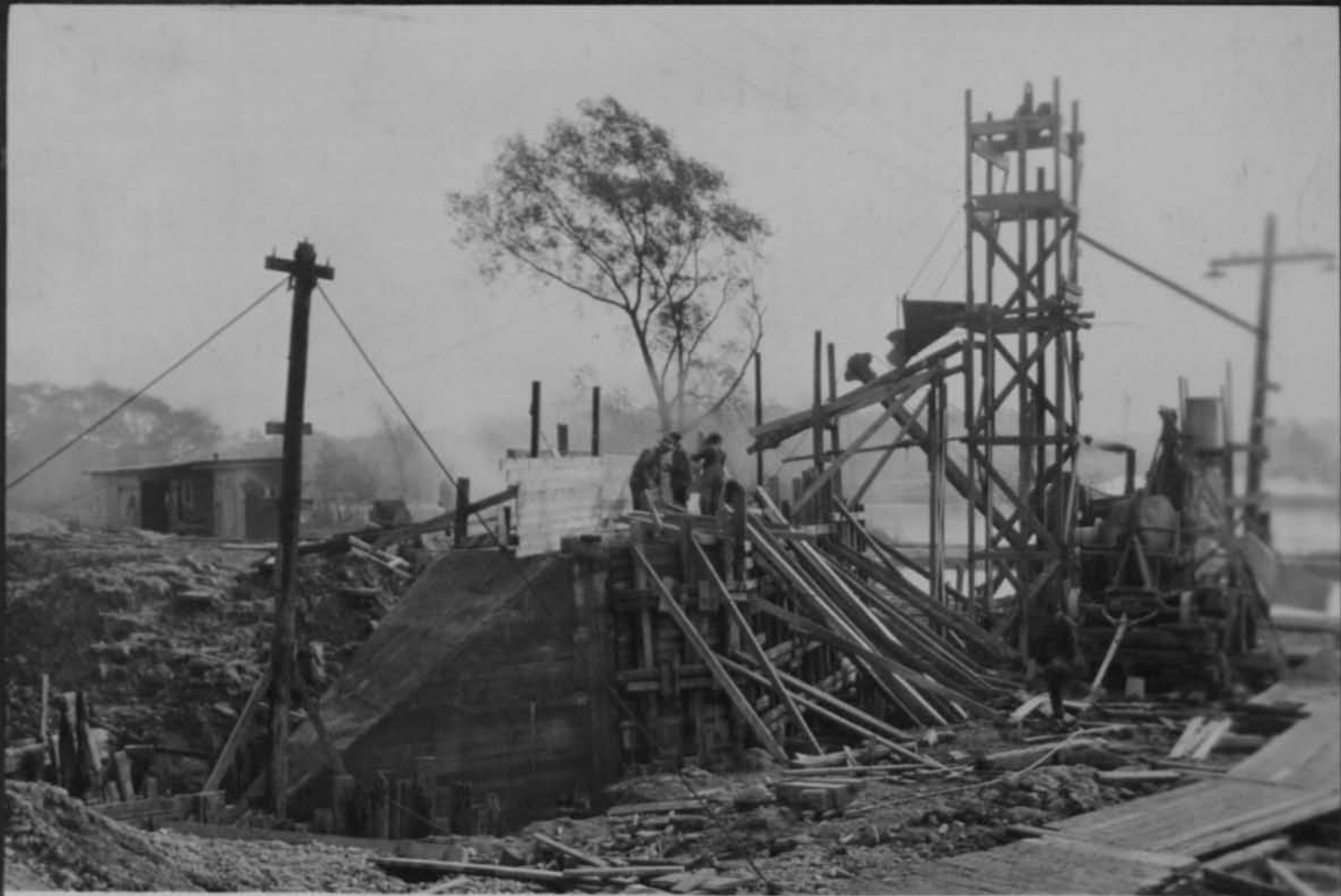
11530 North abutment of Penna crossing Looking east Cont 59 Oct 27 1917
