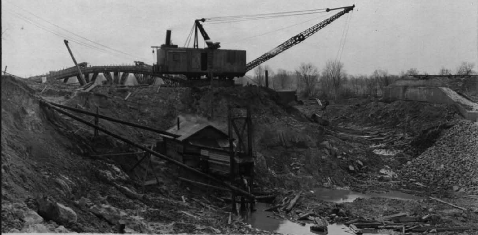
11722 Drag-line operating on west side of Genesee at Penna R R crossing Cont 59 Looking east April 10 1918
