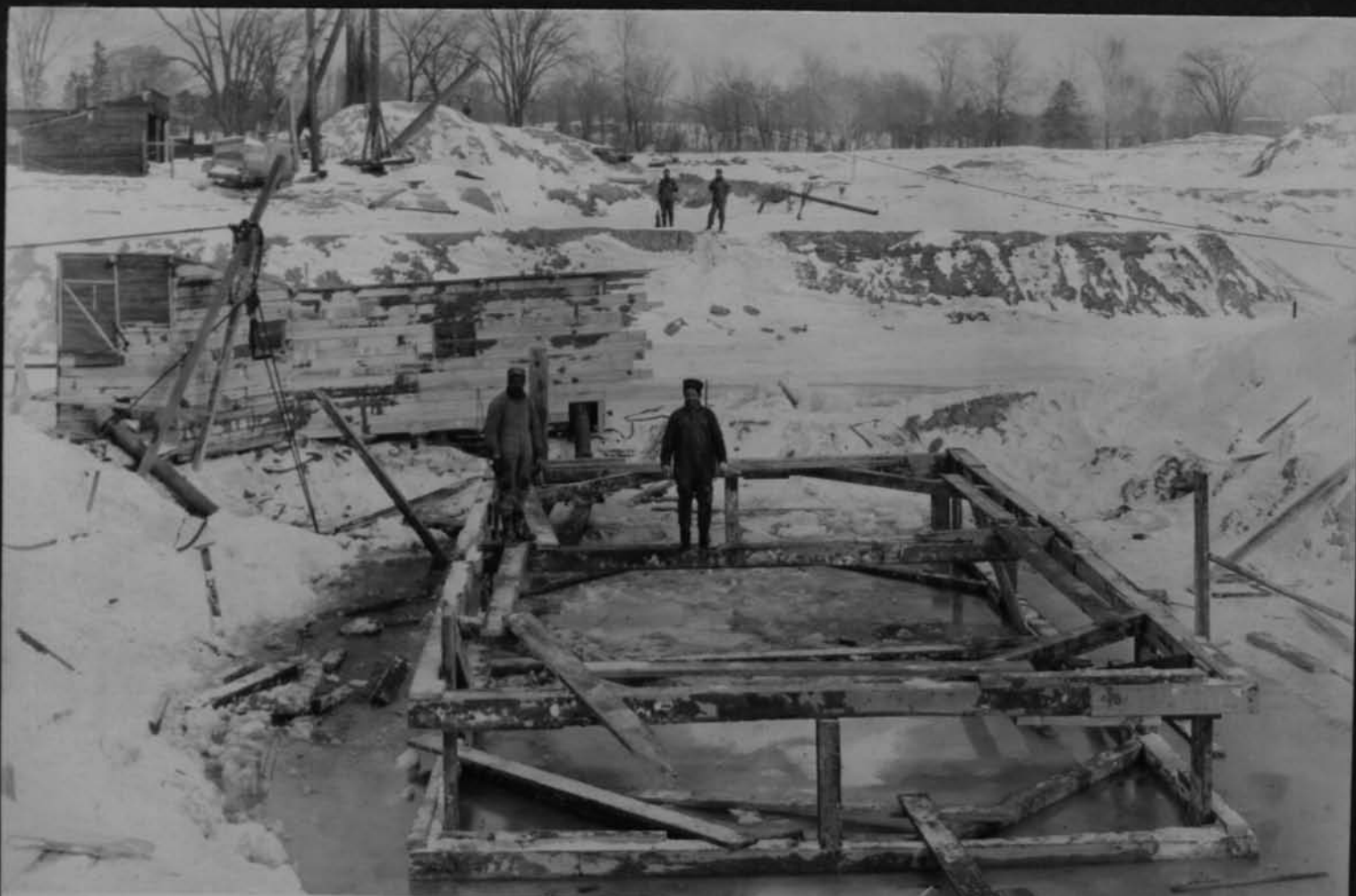
11633 Excavation for foot-bridge on east side of Genesee Looking north Cont 59 Jan 25 1918
