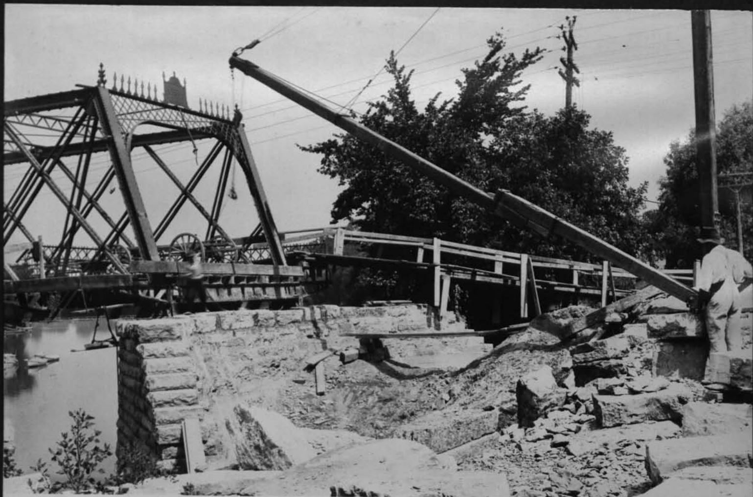
11409 East abutment Elmwood Ave Bridge Cont 59 Aug 7 1917
