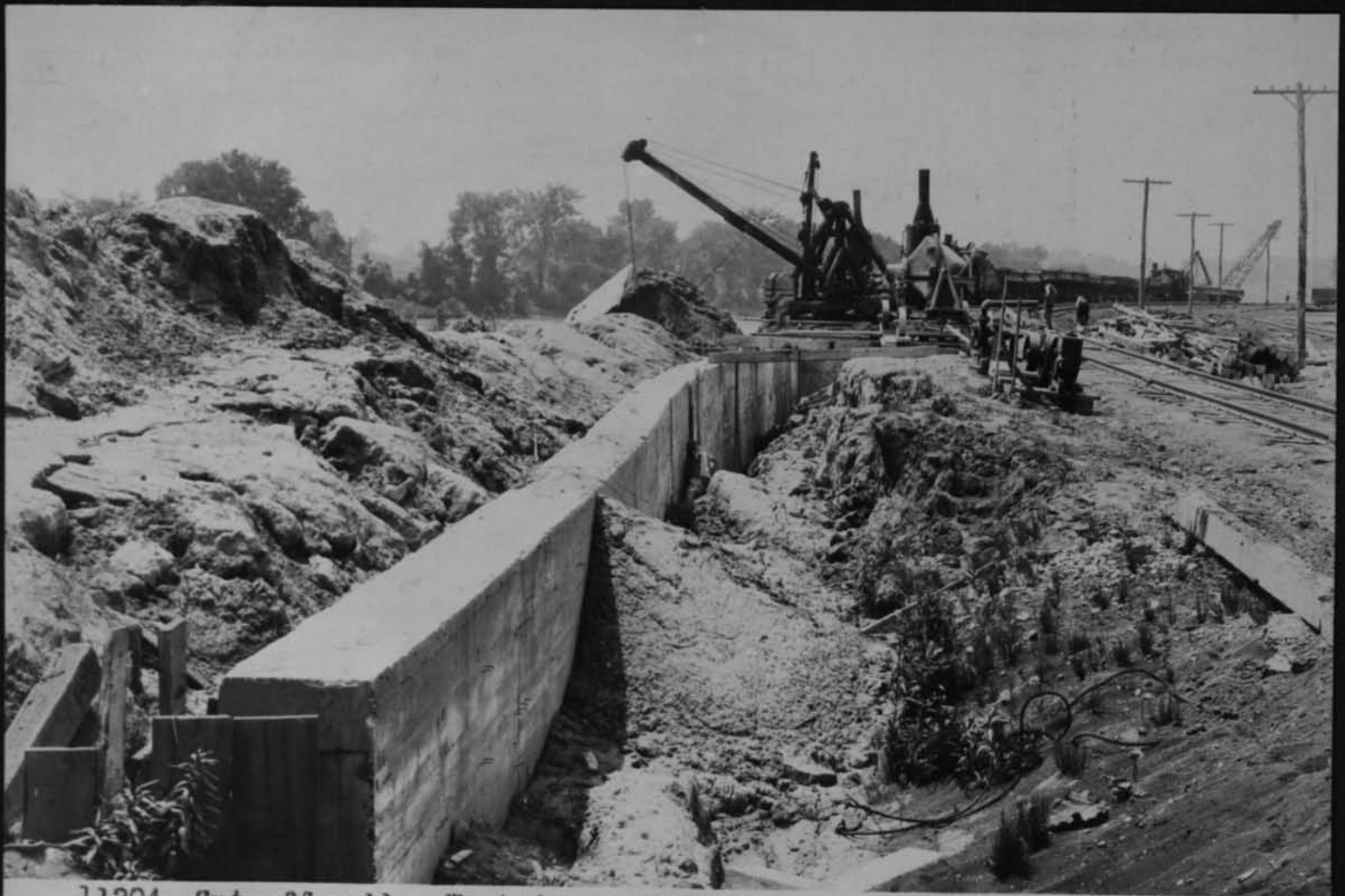
11394 Cut off wall West from Erie bridge Cont 59 July 24 1917
