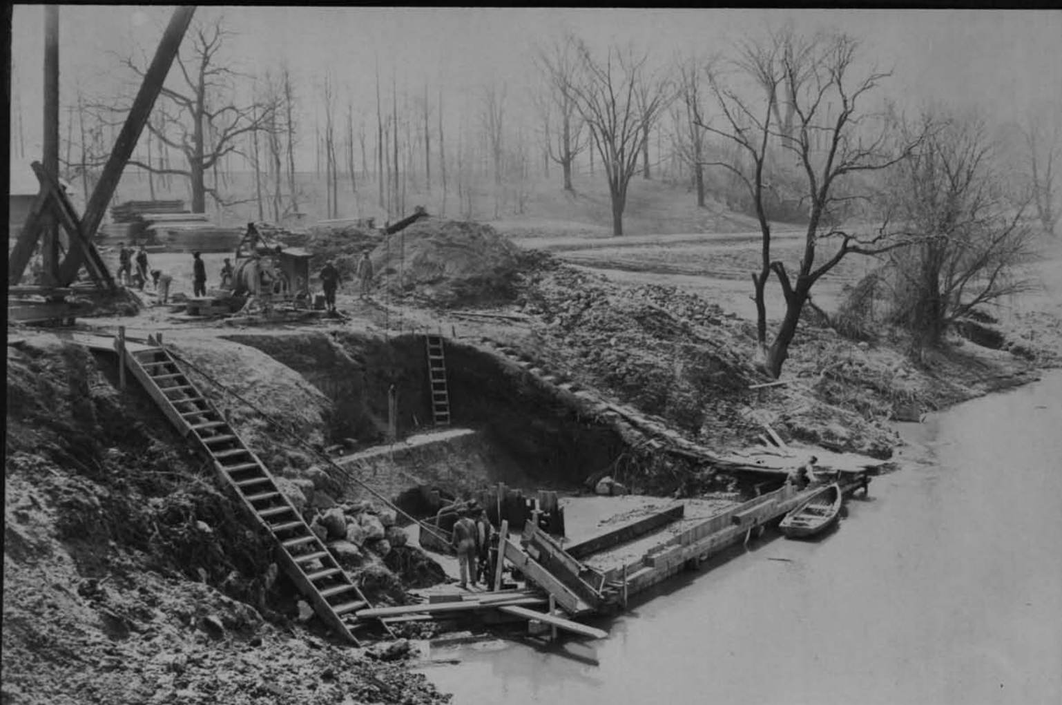
11724 East end of Temporary dam at Elmwood Ave bridge South Park Cont 59 April 15 1918
