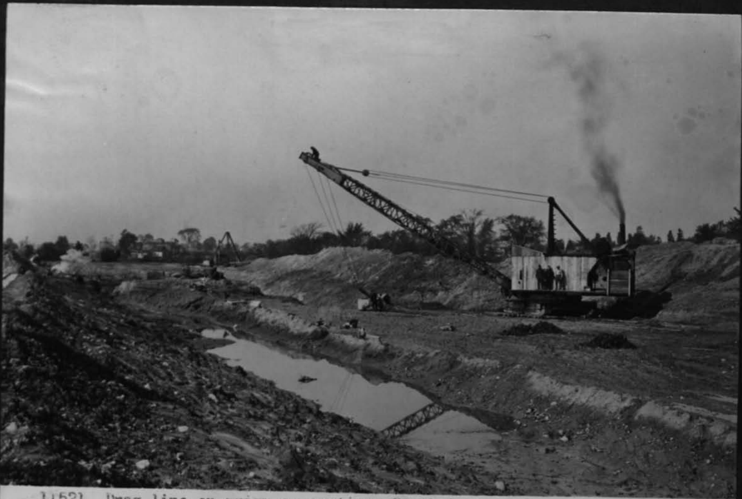
11521 Drag line on prism excavation South Park Cont 59 Oct 17 1917
