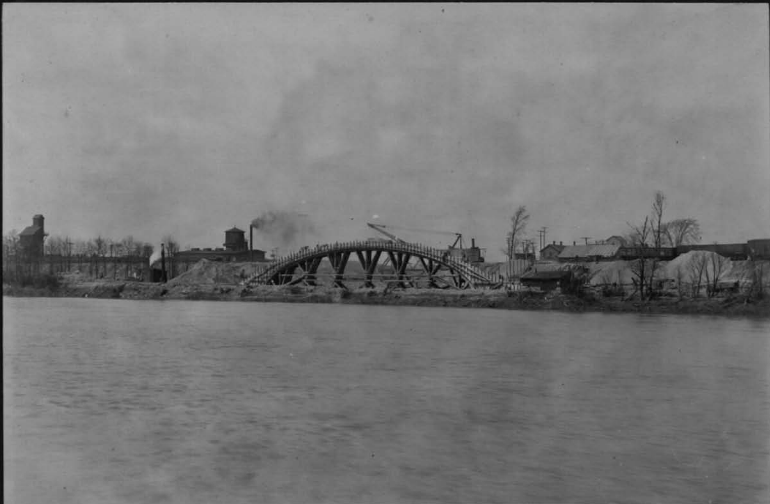
11727 West foot bridge from east side of Genesee river South Park Cent 59 April 15 1918
