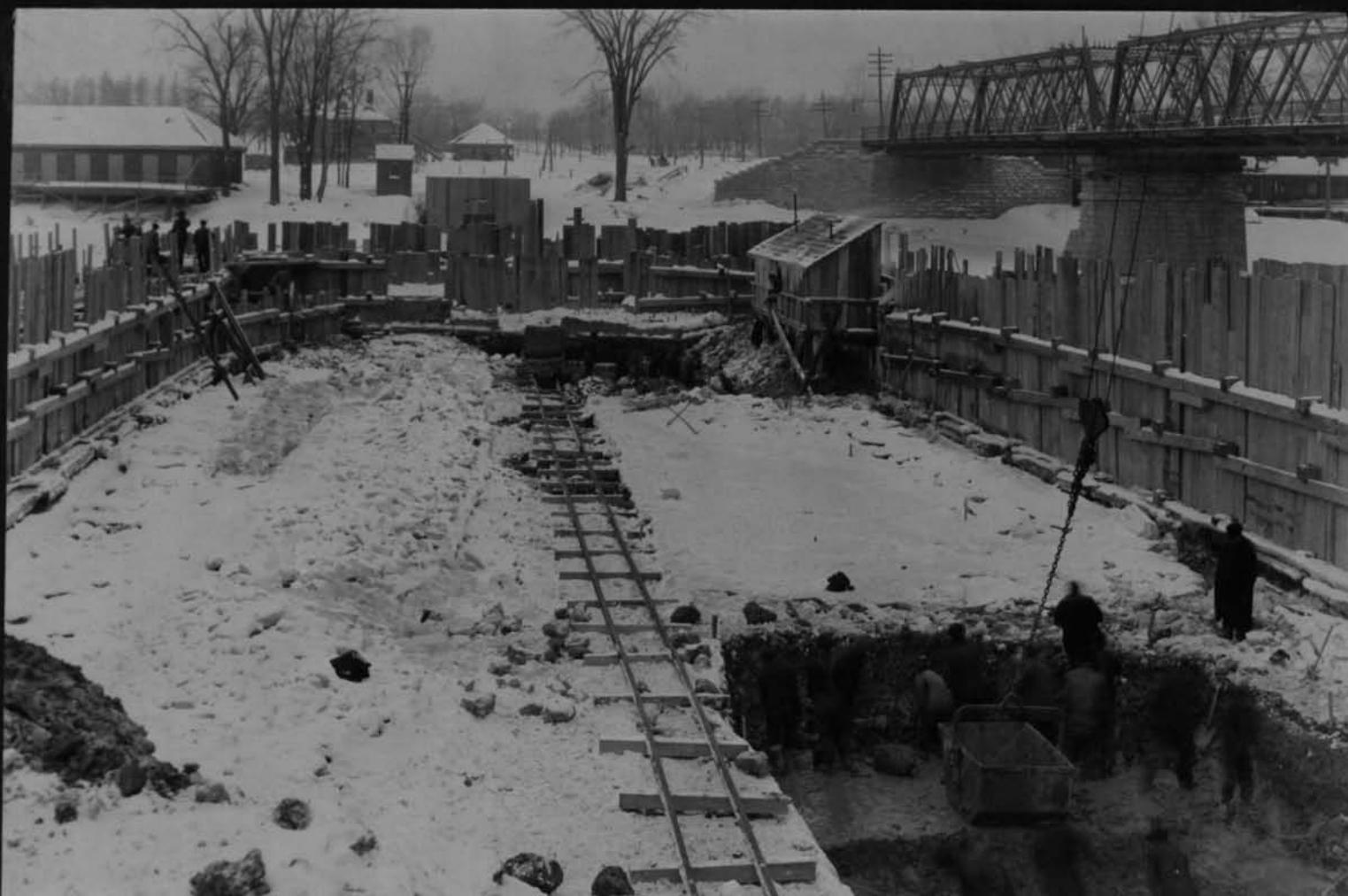
11630 Cofferdam and excavation for east end of temporary dam Looking west Cont 59 Jan 25 1918
