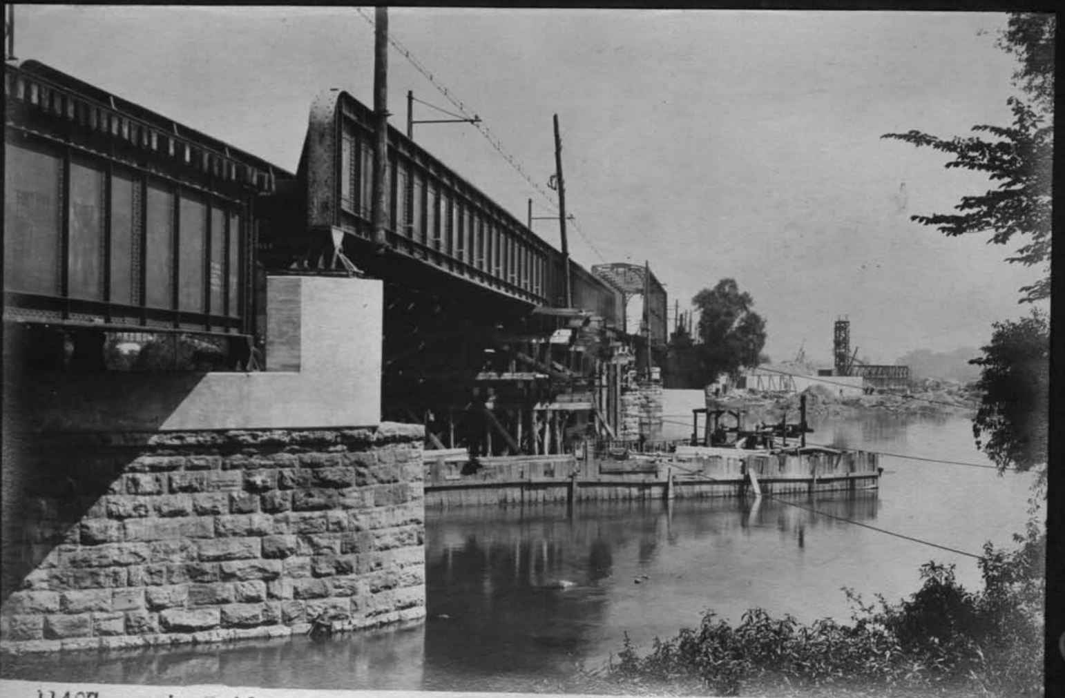
11407 Erie Bridge over Genesee Looking north Cont 59 Aug 7 1917
