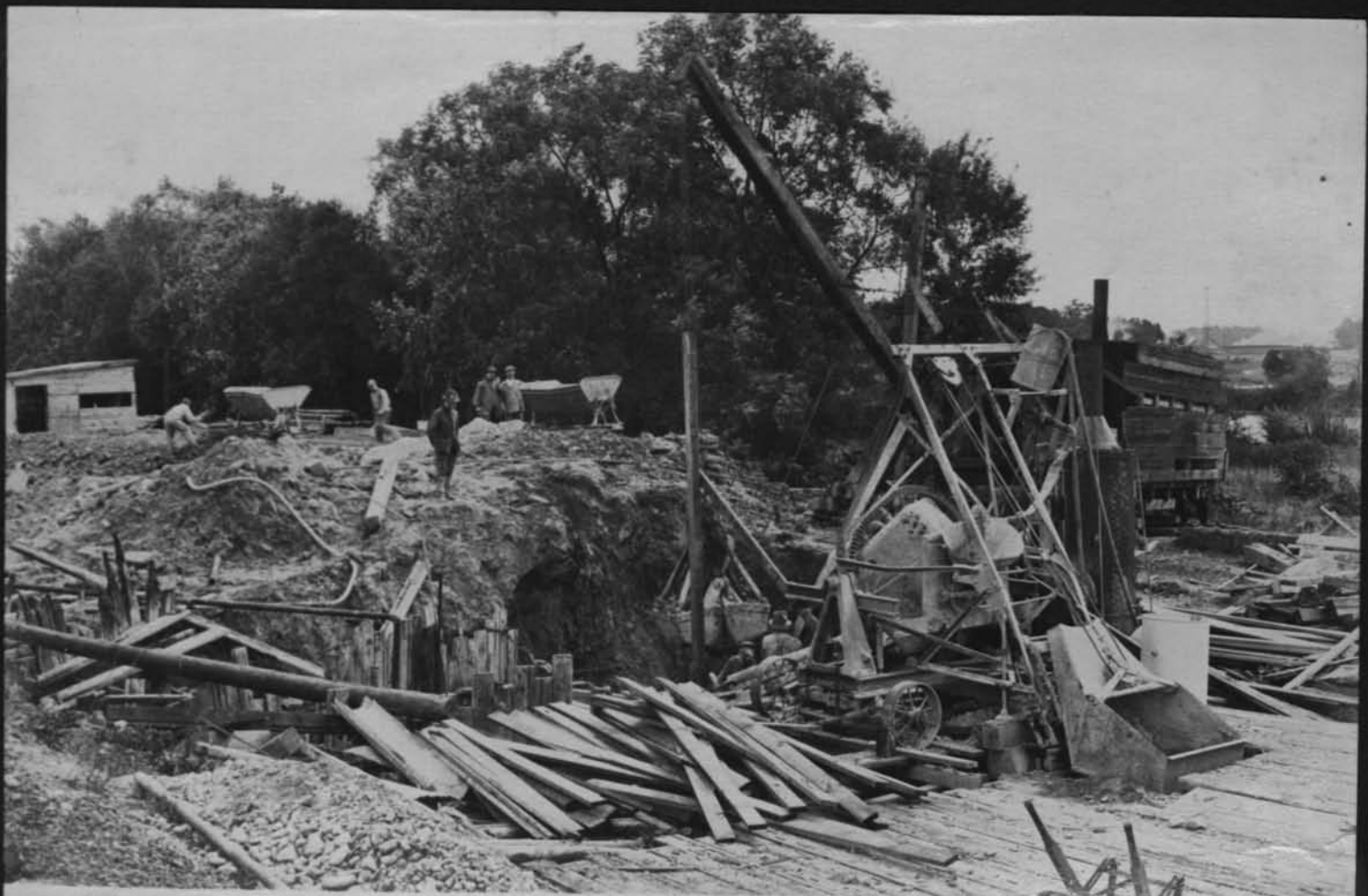
11458 Excavation for abutment of Penna crossing Cont 59 Sept 10 1917
