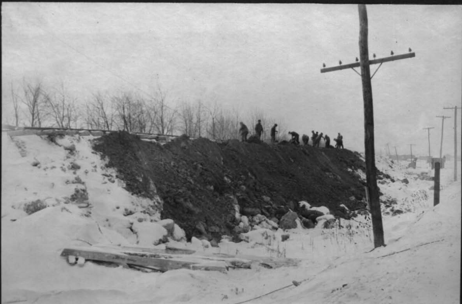
11636 Spoil-bank on south side of Canal at Penna R R crossing Cont 59 Jan 25 1918
