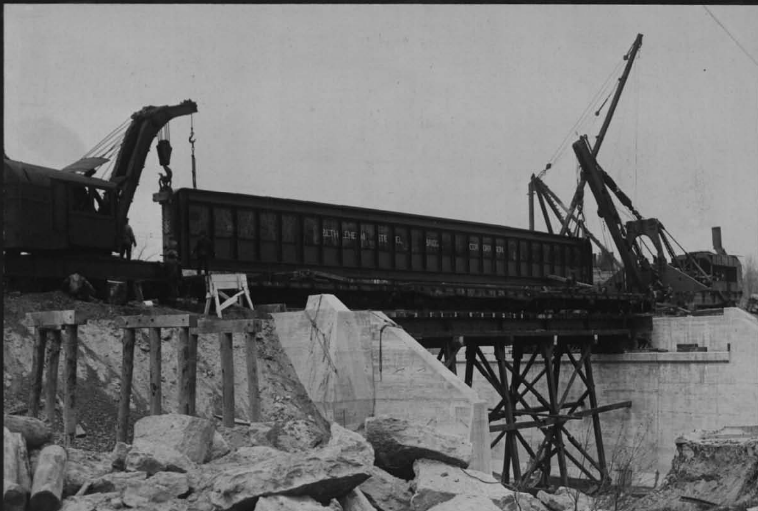
11311 Placing east girder, Lehigh Valley R. R., South Park. On Cont. 59. May 16, 1917.
