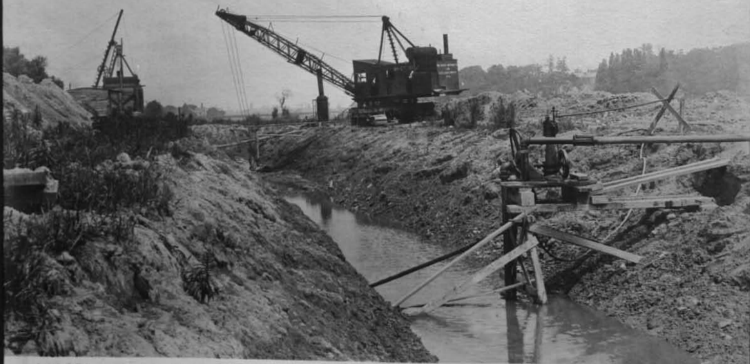
11392 Excavation for river wall near Erie bridge Looking N Cont 59 July 24 1917
