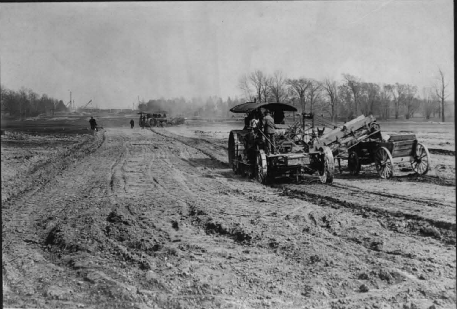
11297 Excavation in South Park west of river. Cont. 59. May 14, 1917.
