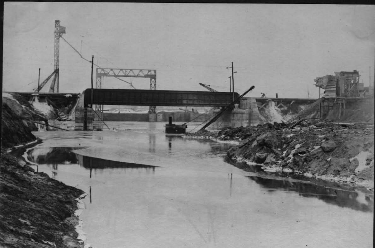
11647 Looking east toward Lehigh Valley R R from Main drive bridge Cont 59 Feb 14 1918
