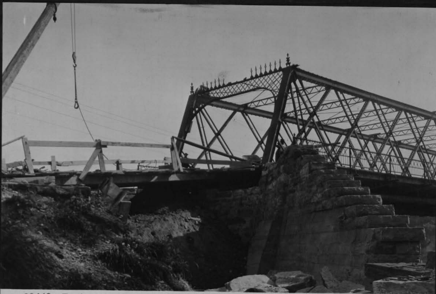
11449 West approach and abutment Elmwood Ave bridge Cont 59 Sept 14 1917
