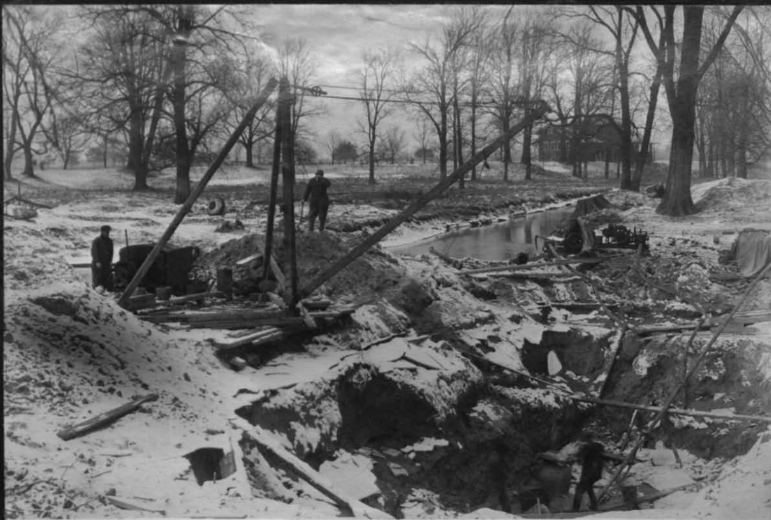
11595 Excavation on upper bridge site South Park Looking north Cont 144 Dec 5 1917
