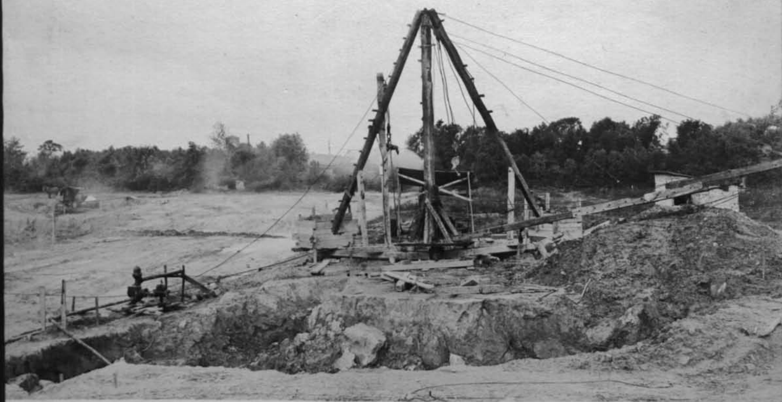
11443 Excavation for north pier of west foot bridge East of river Cont 59 Sept 10 1917
