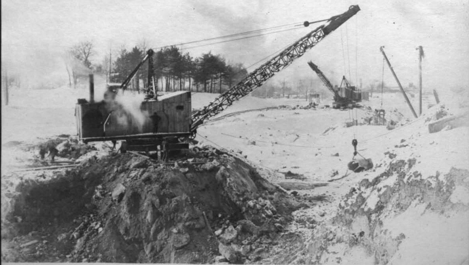
11628 Drag-line operating just west of Erie R R crossing Cont 59 Jan 4 1918
