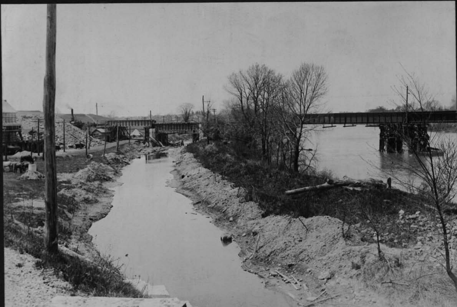
11292 Erie R. R. bridge over Genesee river looking West. Cont. 59. May 14, 1917.
