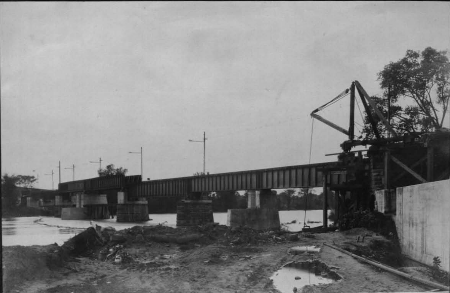
11514 Erie bridge over Genesee Looking south Cont 59 Oct 16 1917
