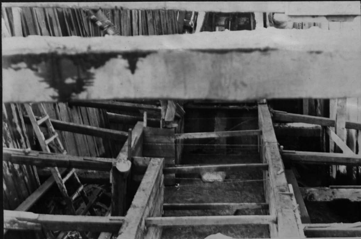
11587 Looking into pit of south abutment Penna R R crossing Cont 59 Dec 18 1917
