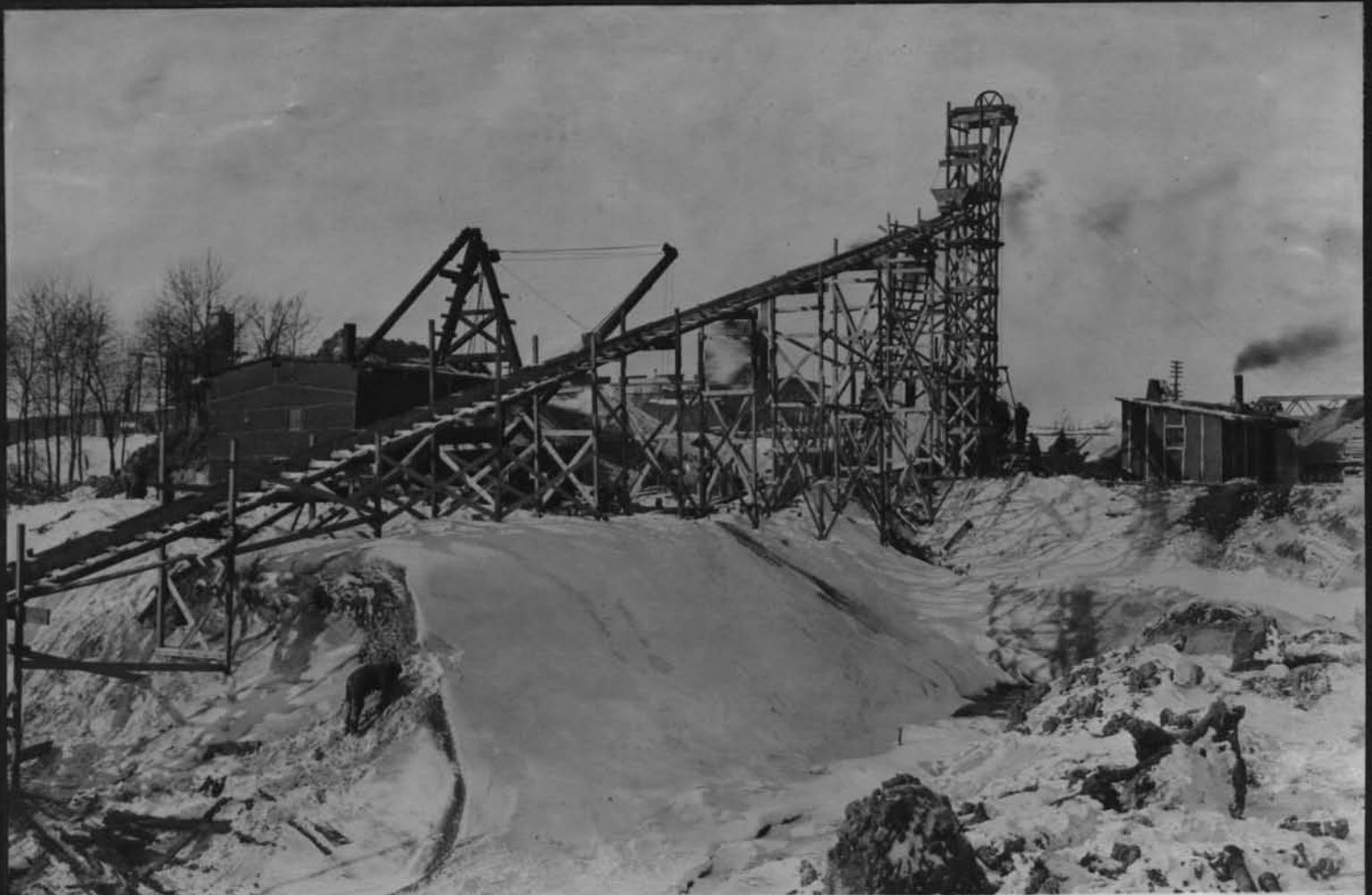
11585 Concrete Tower near Penna R R crossing Cont 59
