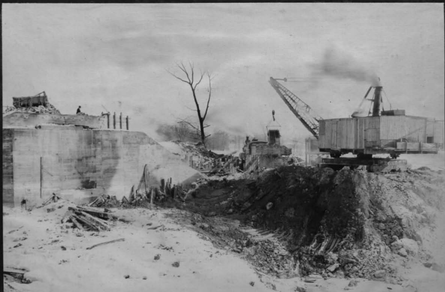
11583 North abutment of Penna R R crossing West side of Genesee River Cont 59 Dec 18 1918
