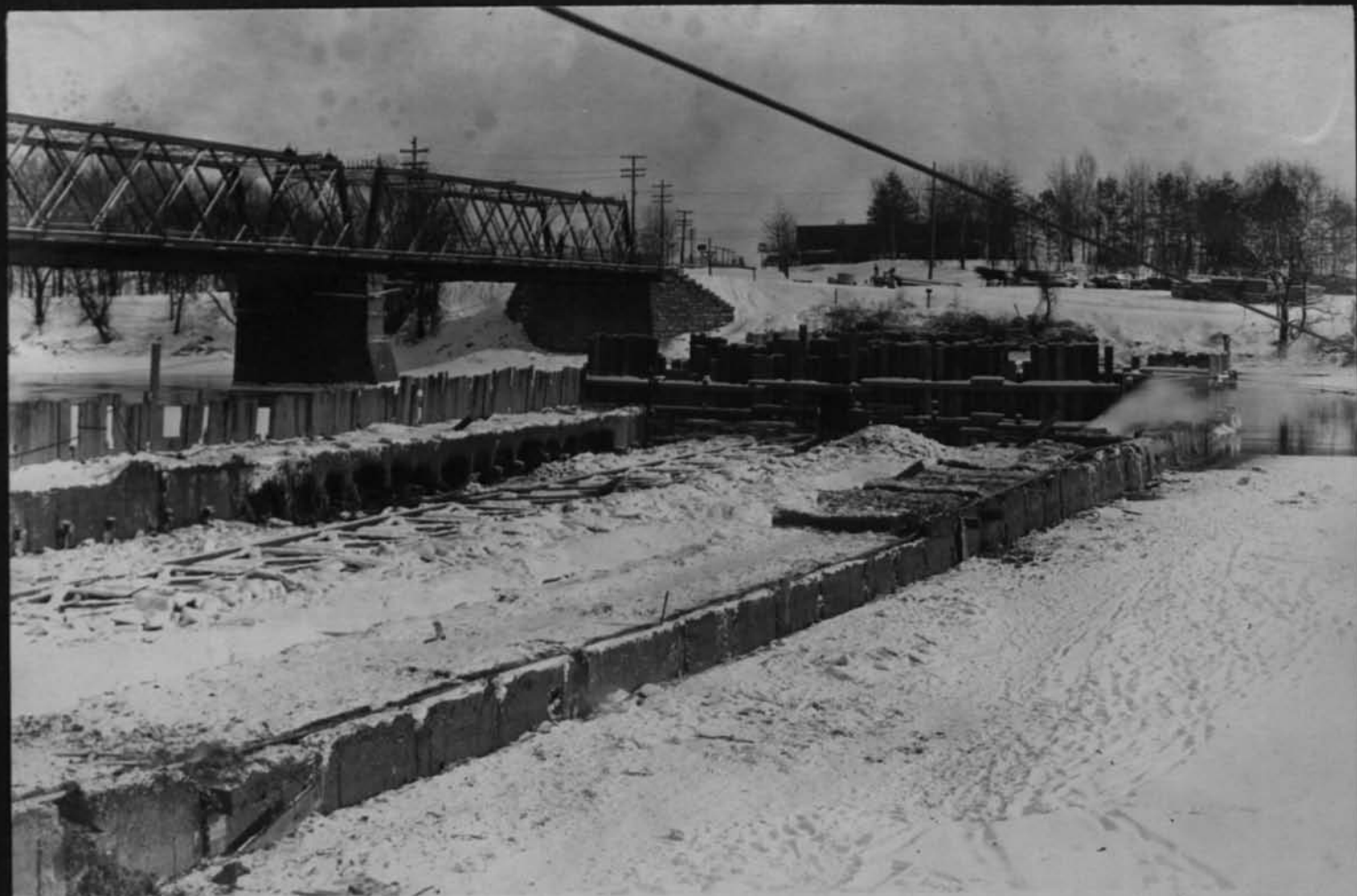
11625 Cofferdam with wood piles drawn Elmwood Ave bridge Looking east Cont 59 Jan 4 1918
