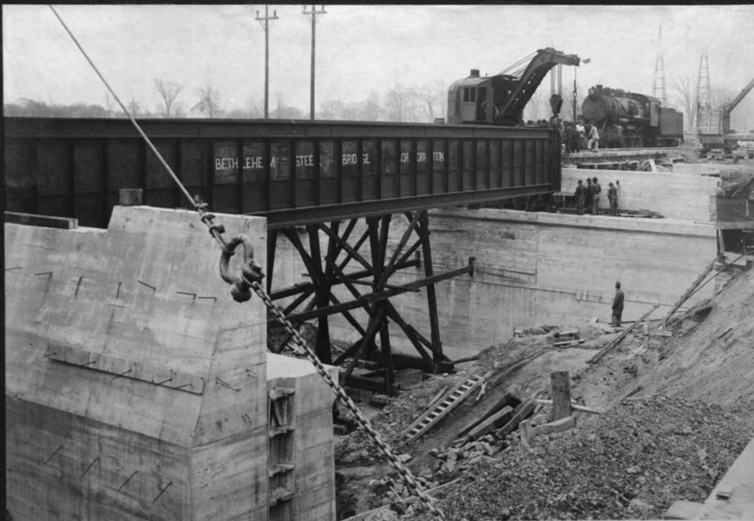
11309 South abutment and girder, Lehigh Valley R. R., South Park. On Cont. 59. May 16, 1917.
