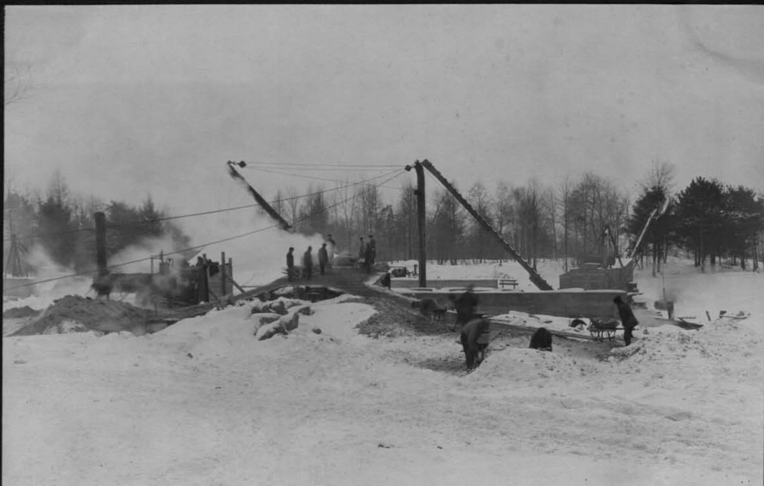
11631 Concrete plant for north abutment for Main drive bridge South Park Cont 59 Jan 25 1918
