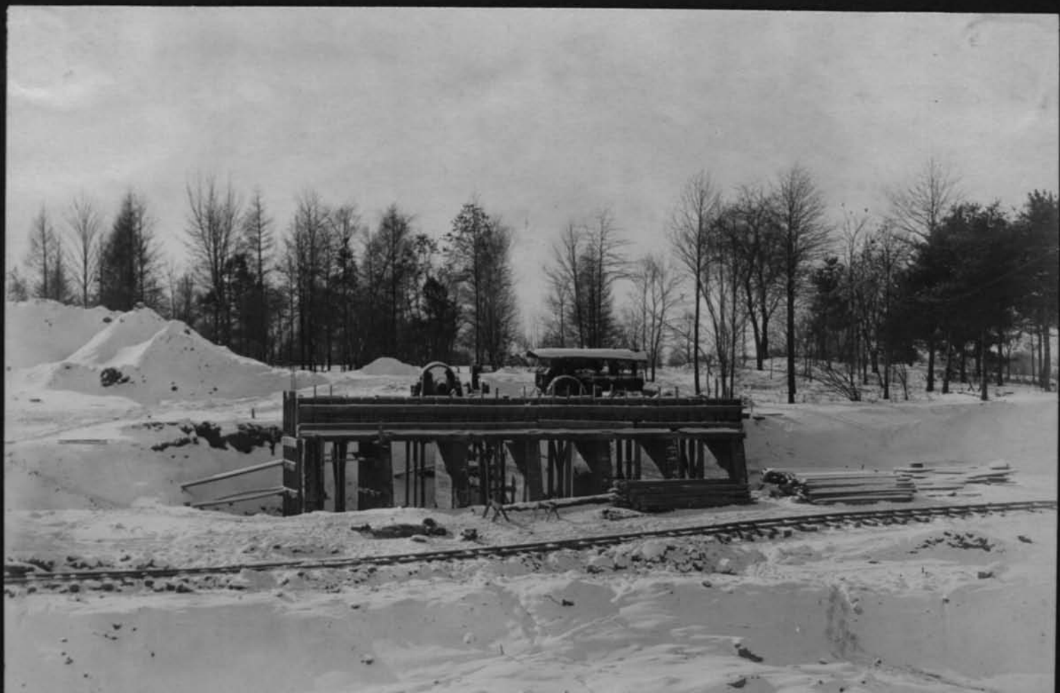
11629 South abutment for Main Drive bridge South Park Looking south Cont 59 Jan 4 1918
