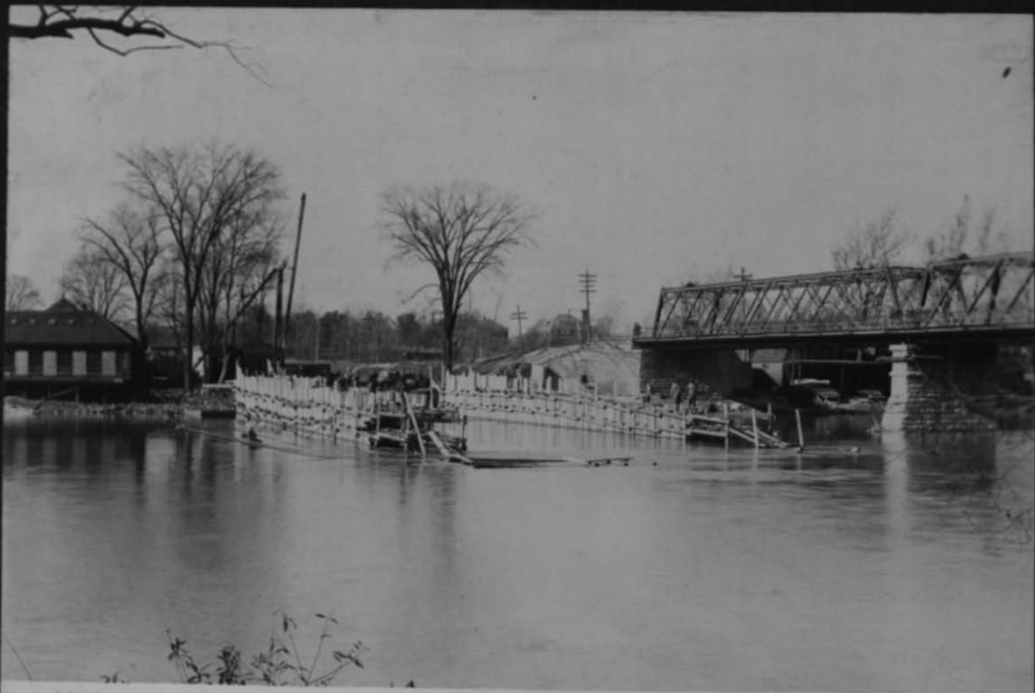
11537 Crib for temporary dam near Elmwood Ave Bridge Cont 59 Nov 13 1917
