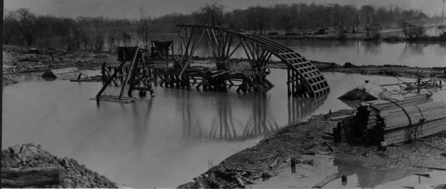
11675 Centering on west foot bridge at high water Looking east Cont 59 March 18 1918
