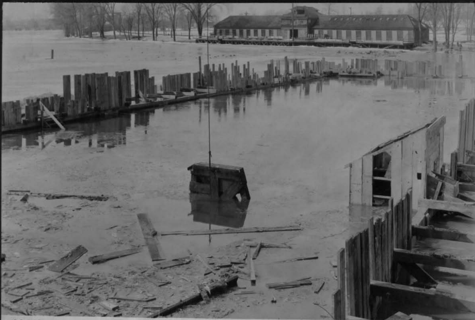
11642 Temporary dam at high water Looking west Cont 59
