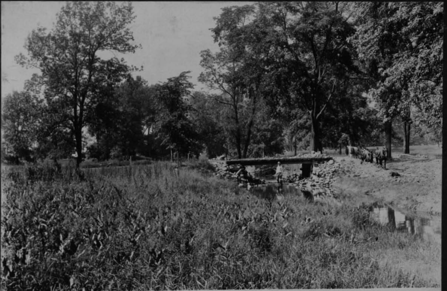
11372 South bridge site Looking north Cont 144 July 5 1917
