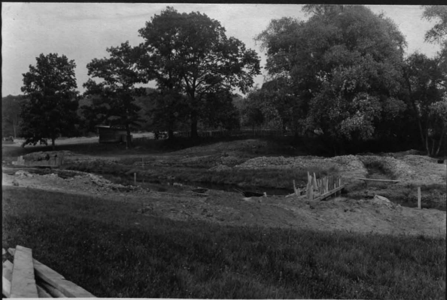
11370 Excavation on north bridge site Looking east Cont 144 July 5 1917
