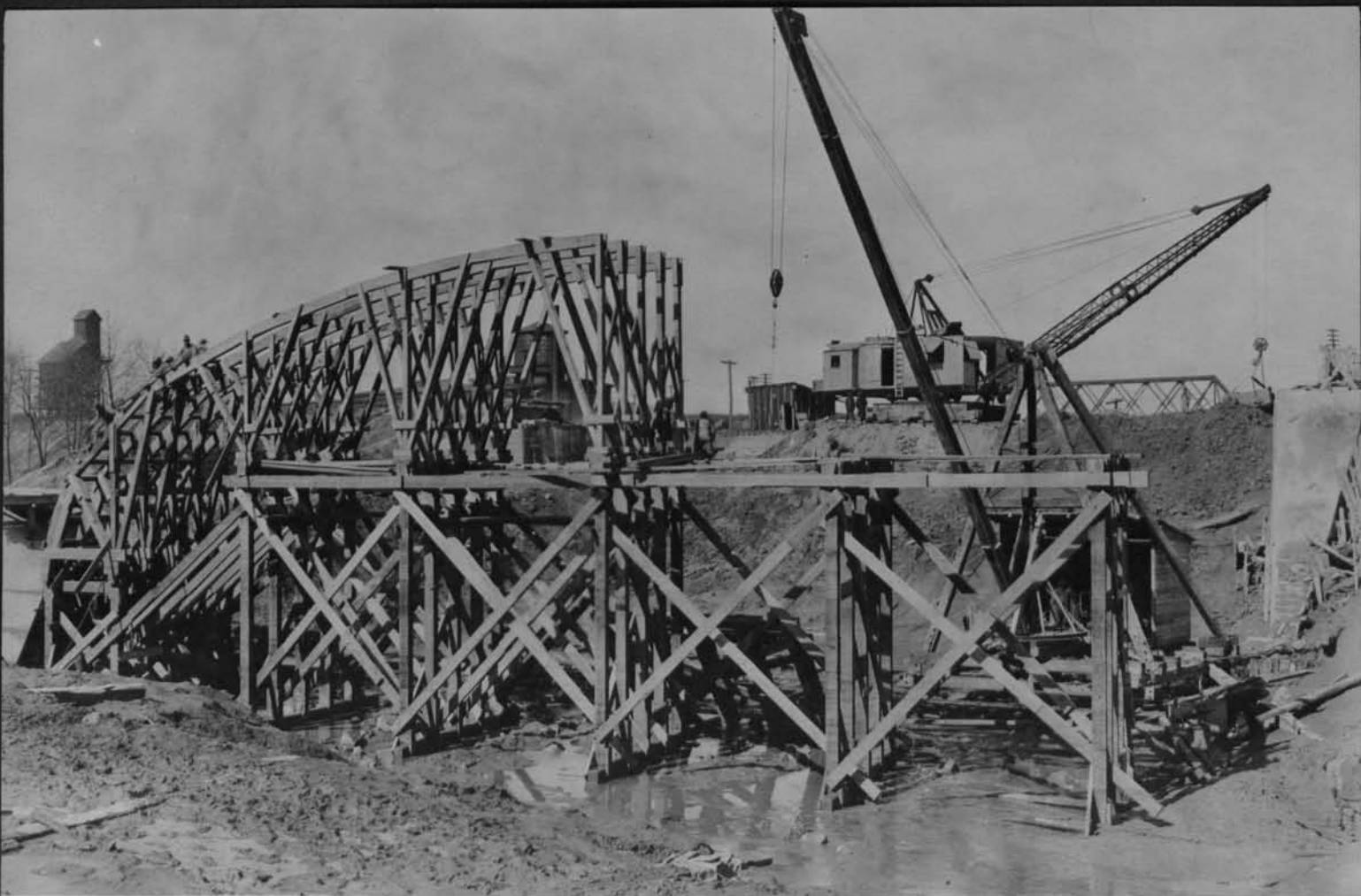
11676 False work for Foot Bridge and dragline on west side Genesee Cont 59 March 22 1918
