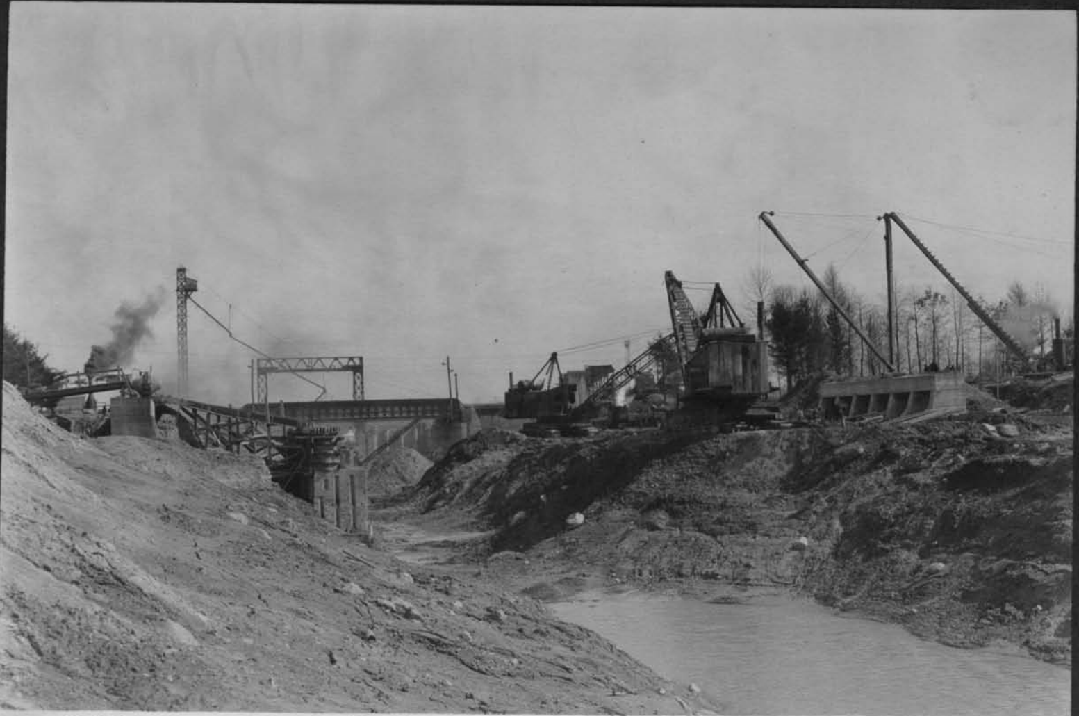
11720 Excavation at Main drive bridge South Park Looking east Cont 59 April 4 1918
