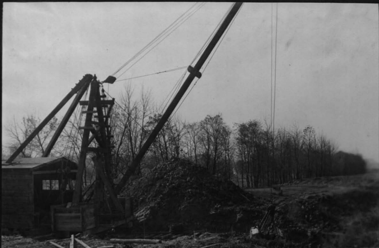
11529 Derrick excavating for south pier of Penna crossing Cont 59 Oct 27 1917
