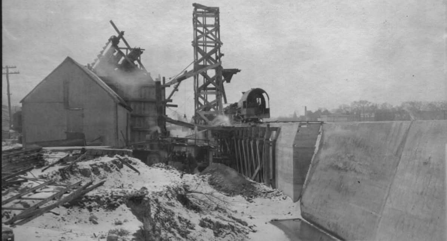
11570 River wall south of Lehigh Valley Round House Looking south Cont 59 Dec 5 1917
