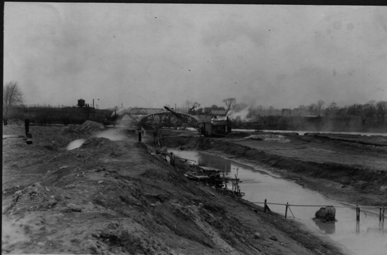
11770 Prism excavation in South Park Looking west toward Genesee River Cont 59 April 23 1918
