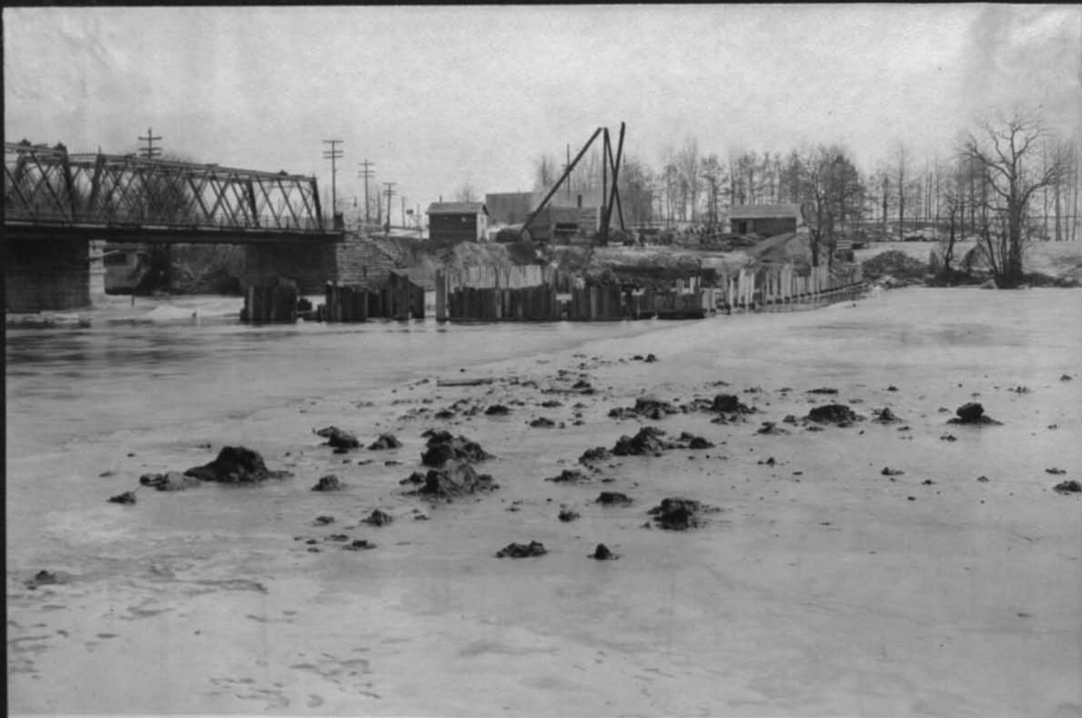
11644 Coffor-dam for temporary dam at high water Looking east Cont 59 Feb 13 1918
