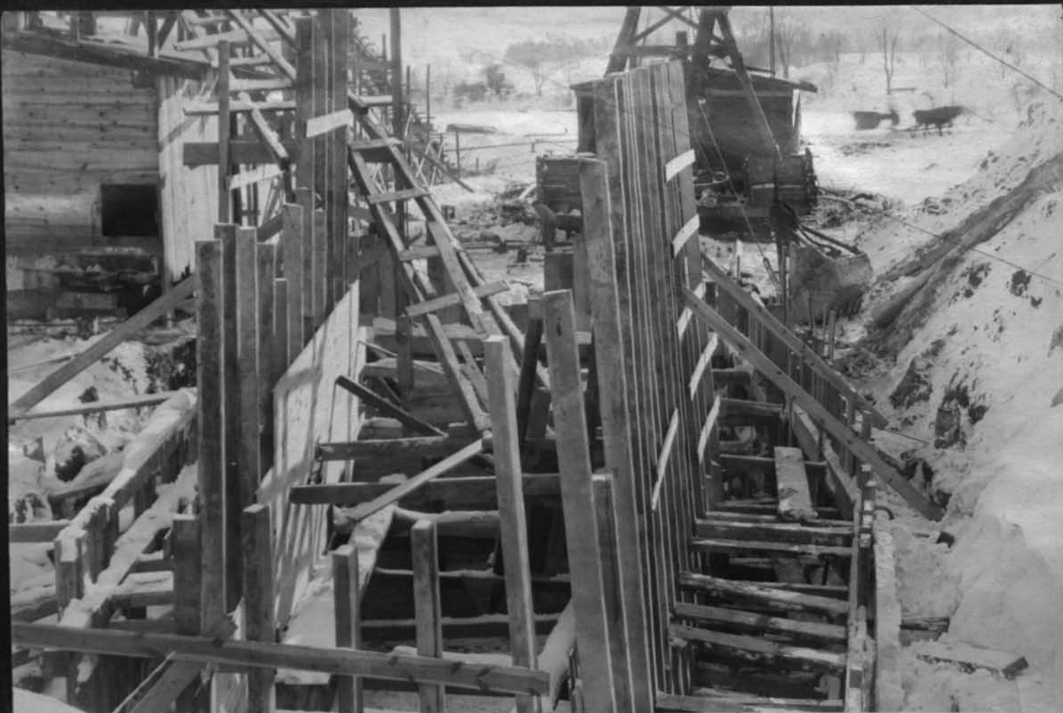
11586 Forms for south abutment of Penna R R crossing Looking east Cont 59 Dec 18 1917
