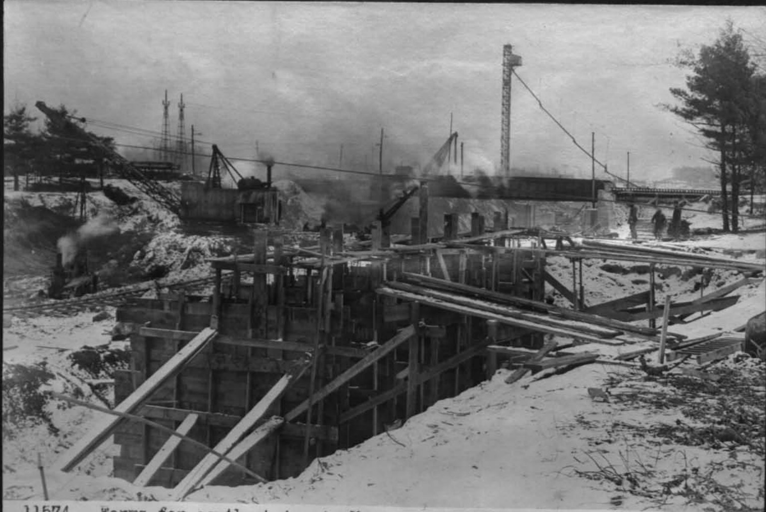
11574 Forms for south abutment Main drive bridge South Park Cont 59 Dec 5 1917
