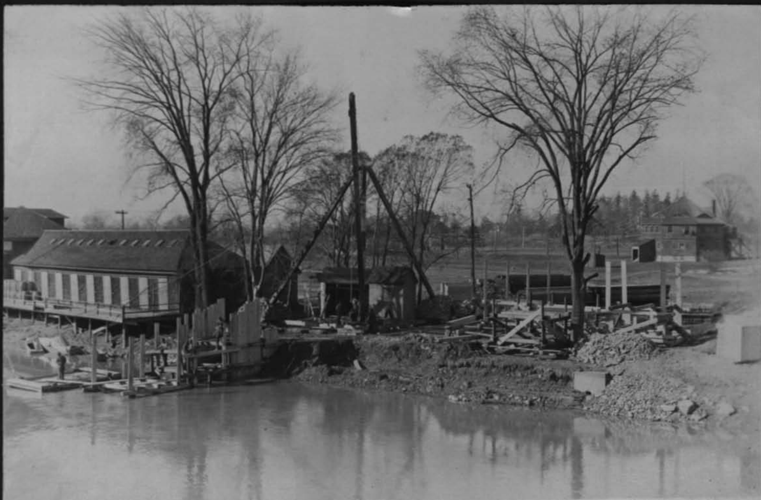
11536 Crib for temporary dam near Elmwood Ave Bridge Cont 59 Nov 5 1917
