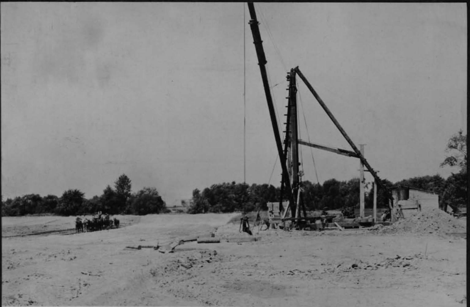
11410 Equipment for pier excavation East of Genesee Cont 59 Aug 7 1917
