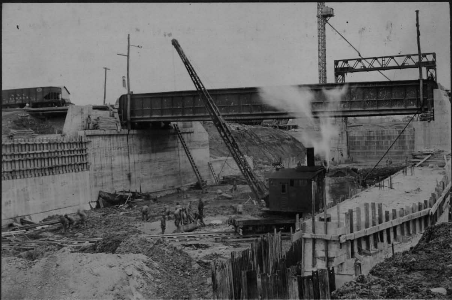
11728 Excavation under Lehigh Valley crossing Looking east Cont 59 April 23 1918
