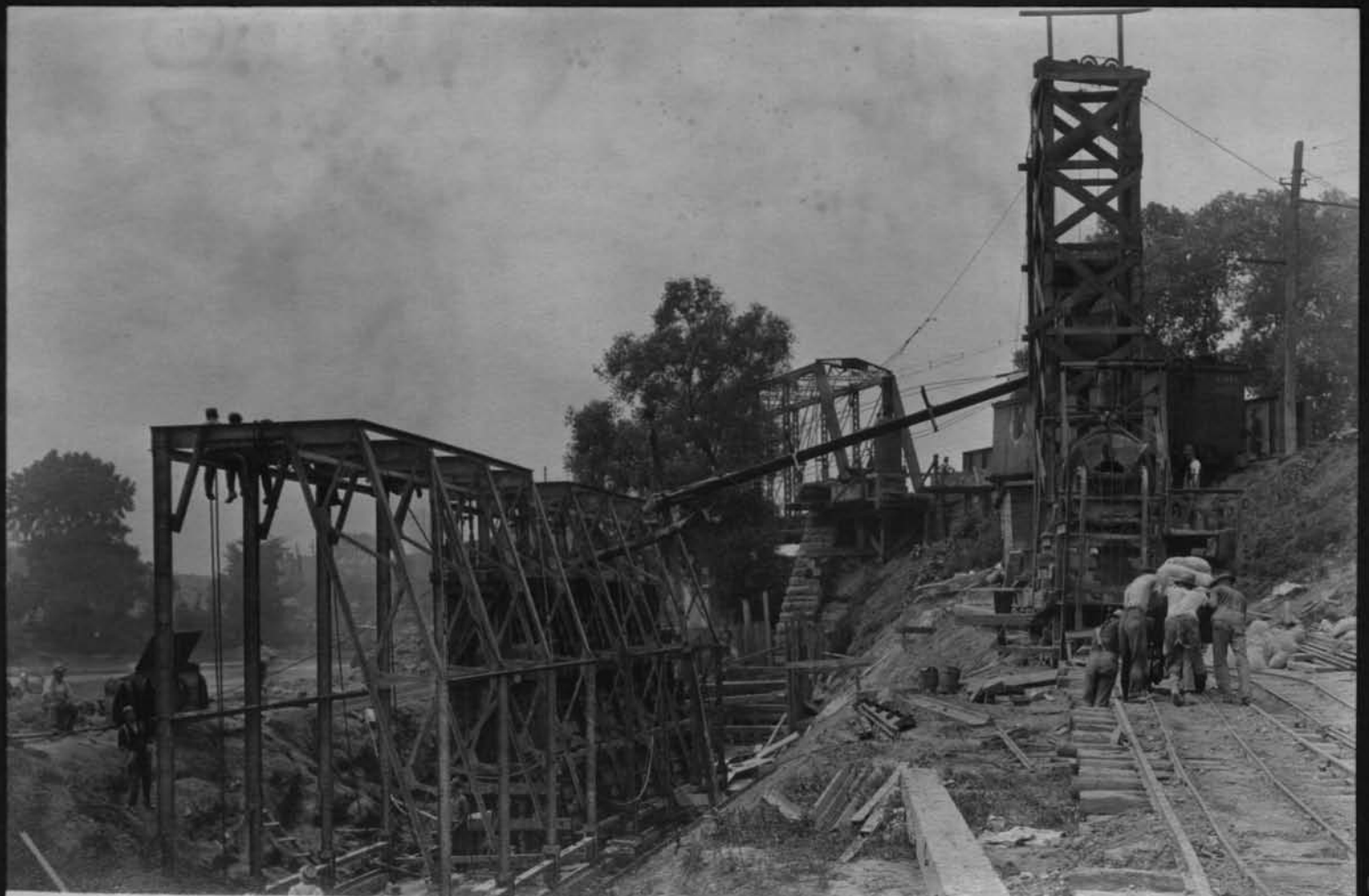
11391 River wall near Erie bridge Looking west Cont 59 July 24 1917
