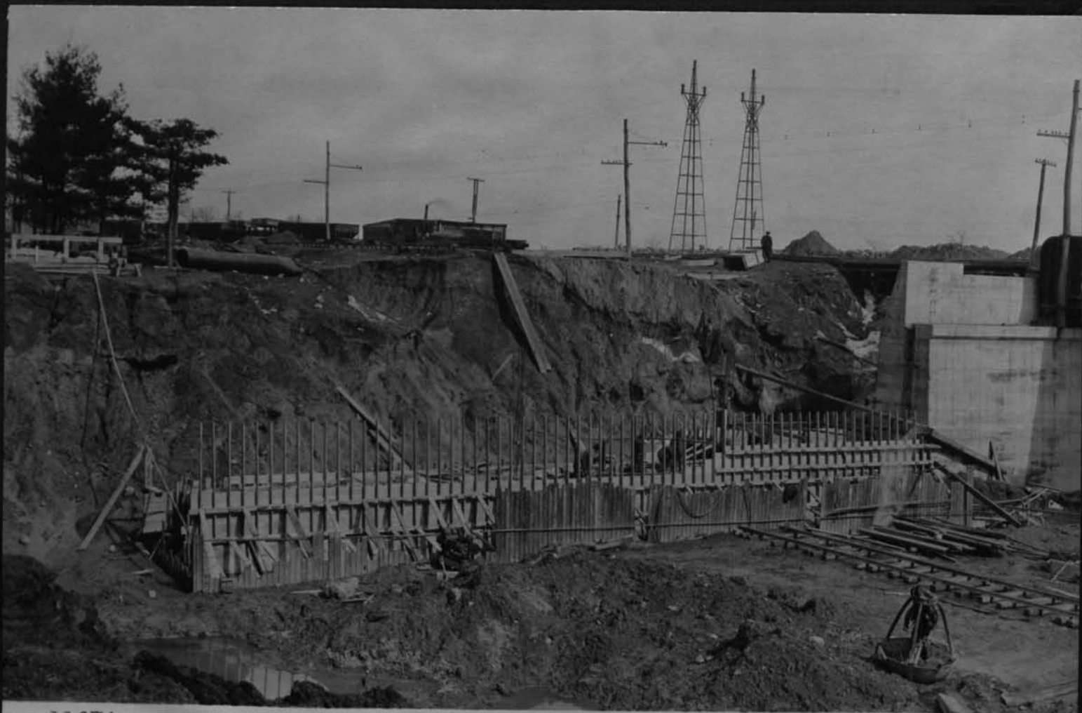
11674 North abutment for Erie R R crossing South Park Cont 59 March 13 1918
