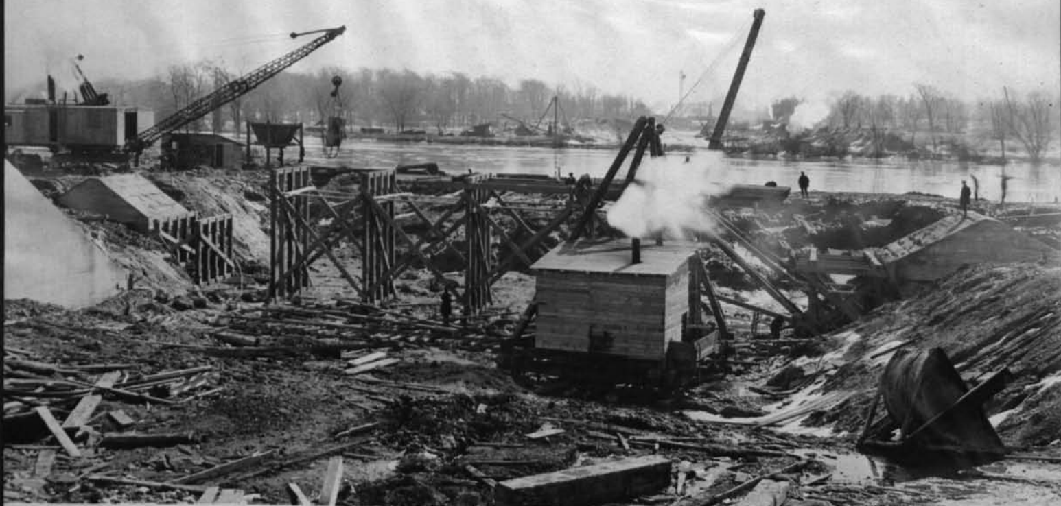
11673 Abutments and centering for foot bridge near Penna crossing Cont 59 March 13 1918
