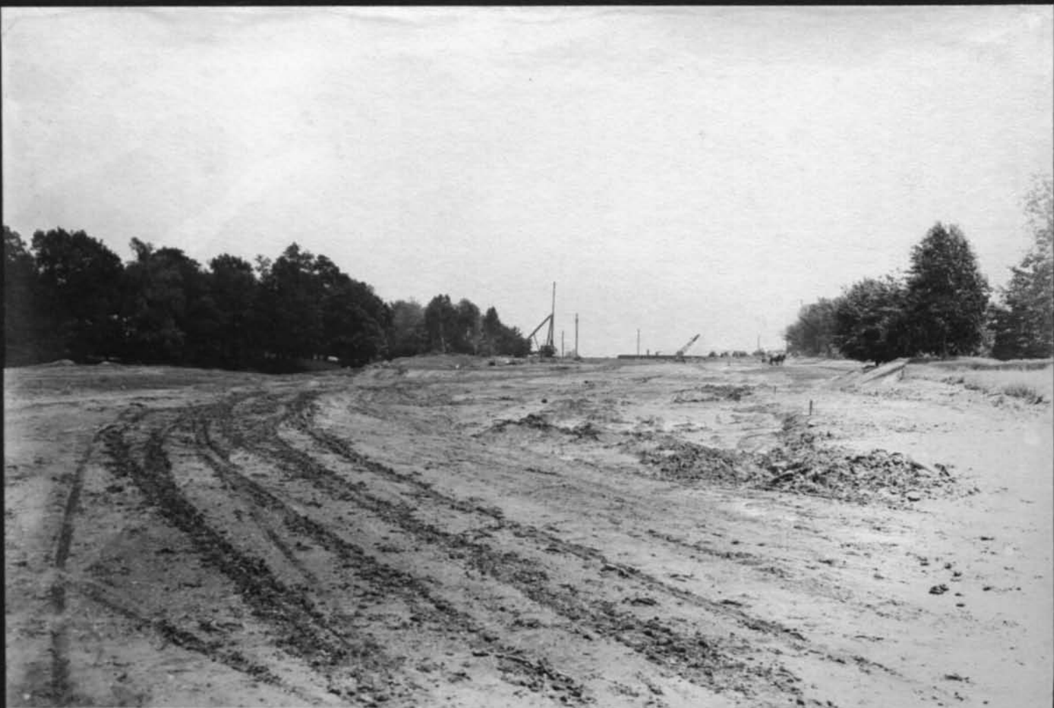
11332 Excavation in South Park Looking east toward Lehigh Valley Cont 59 June 20 1917
