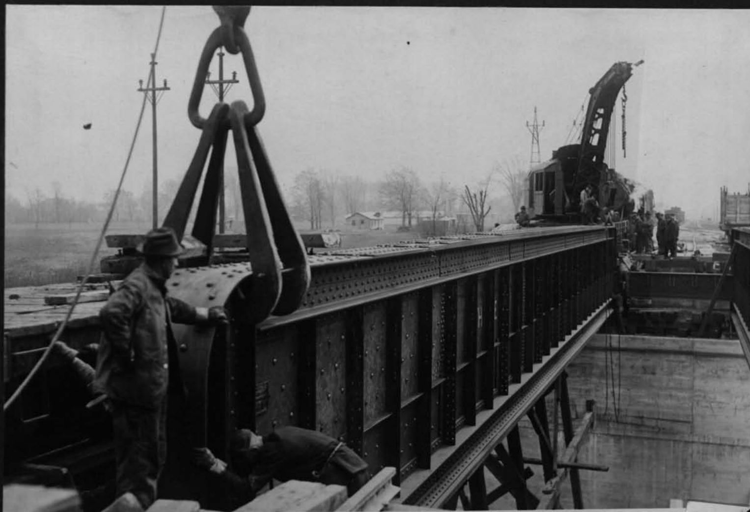
11310 Setting east girder, Lehigh Valley R. R., South Park. On Cont. 59. May 16, 1917.
