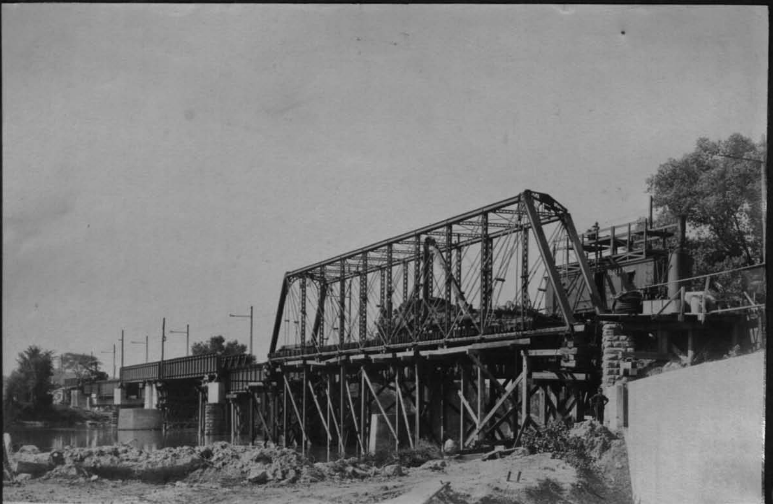
11446 Erie R R bridge over Genesee River Cont 59 Sept 13 1917
