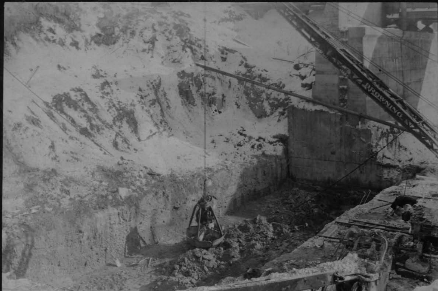
11588 Excavation for north abutment of Erie R R crossing Cont 59 Dec 18 1917
