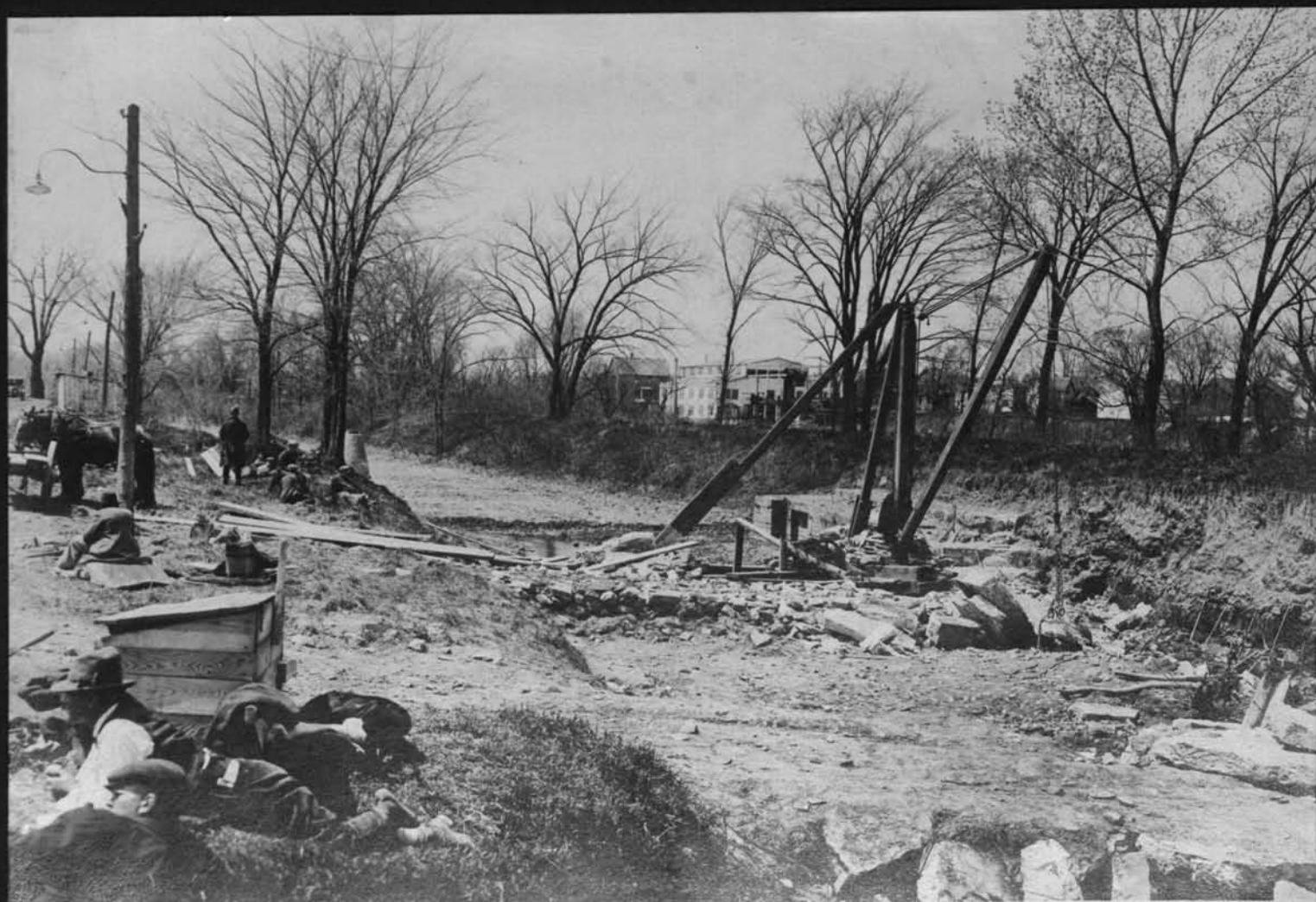
11293 Removing old lock from feeder north of head gates. Cont. 59. May 14, 1917.
