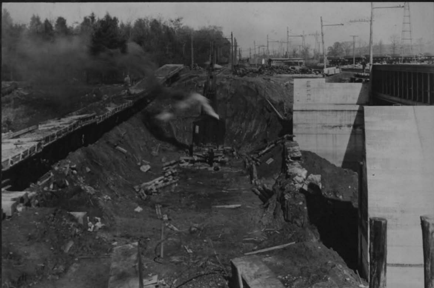
11526 Excavation for Erie crossing Looking north Cont 59 Oct 26 1917
