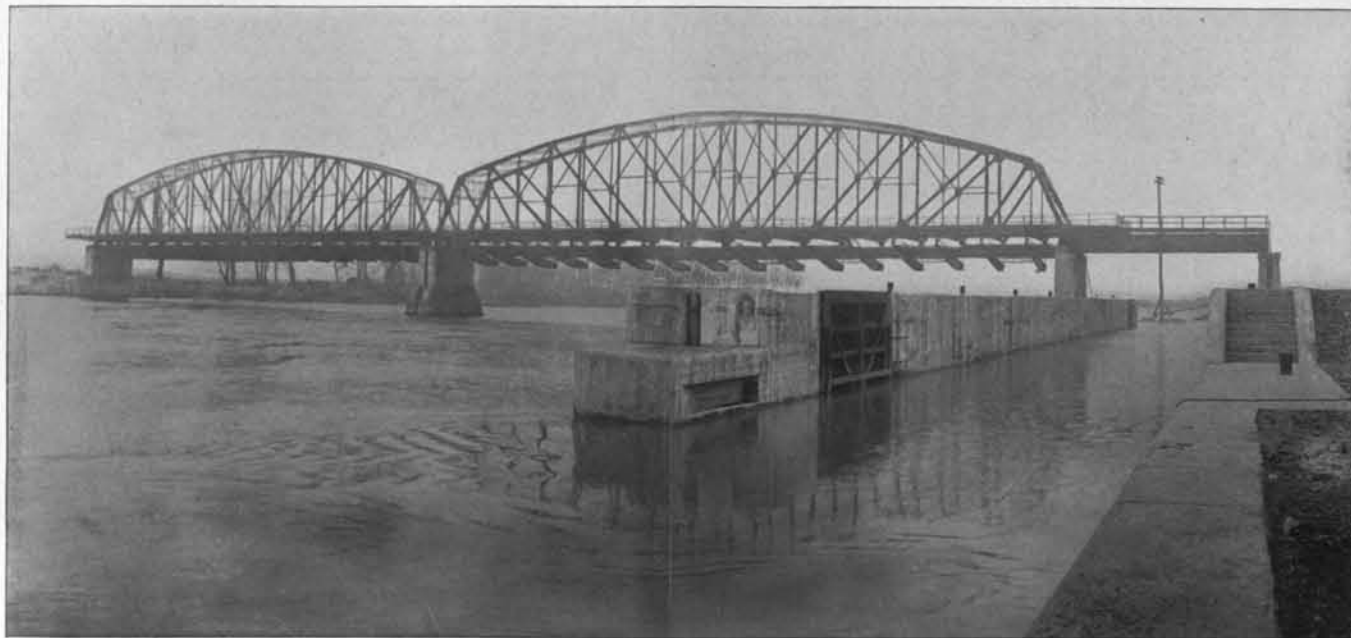
Another lock and movable dam of bridge type in the Mohawk. This view shows the gates raised and the uprights upon which they slide swung to a horizontal position beneath the bridge floor, ready for winter or flood conditions.
