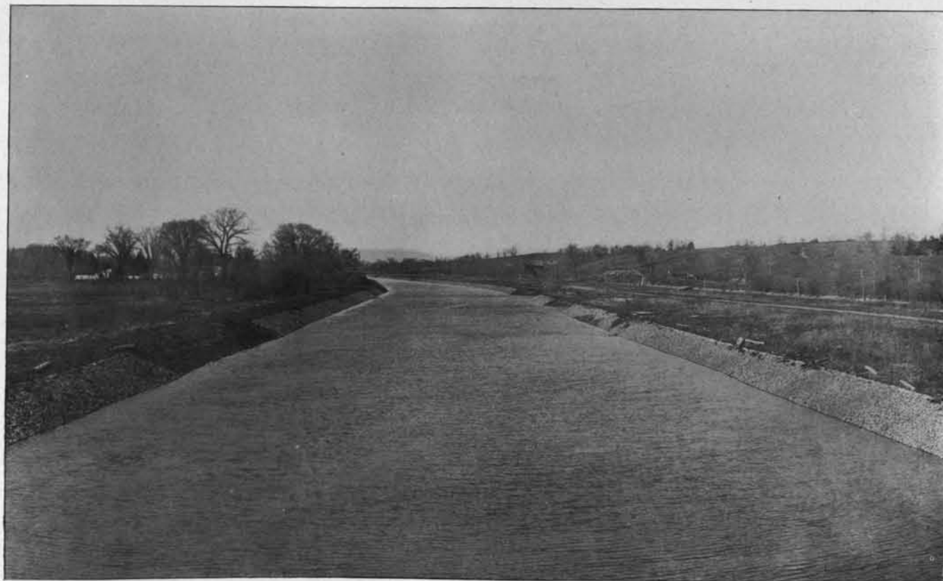
A section of completed canal, filled with water, where a land line of the Champlain division diverges from the Hudson river between Fort Miller and Crocker's Reef.
