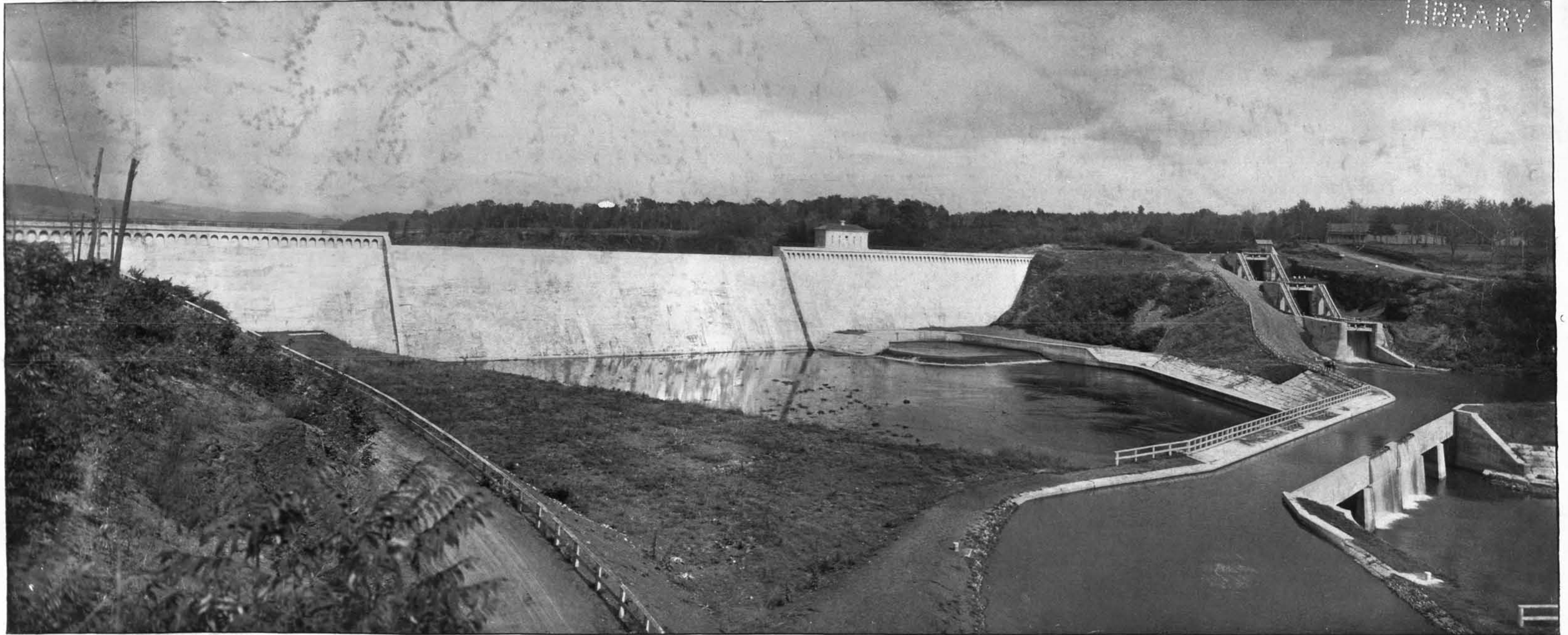
The dam at Delta reservoir. Also the relocated Black River canal, crossing the Mohawk on an aqueduct and ascending the precipitous river bank by a flight of three locks. This dam is 1,100 feet long and has a maximum height of 100 feet and a masonry content of 90,000 cubic yards. The reservoir is four miles long by two miles wide, having a capacity of 2,750,000,000 cubic feet.
