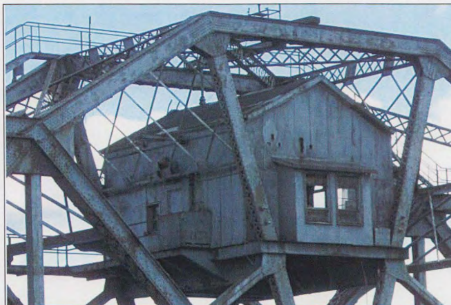
Figure 8. The north and west elevations of the control house.
