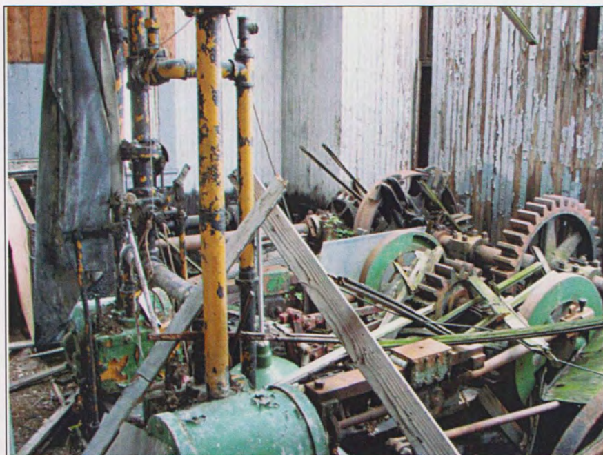
Figure 12. Machine room in the control house.
