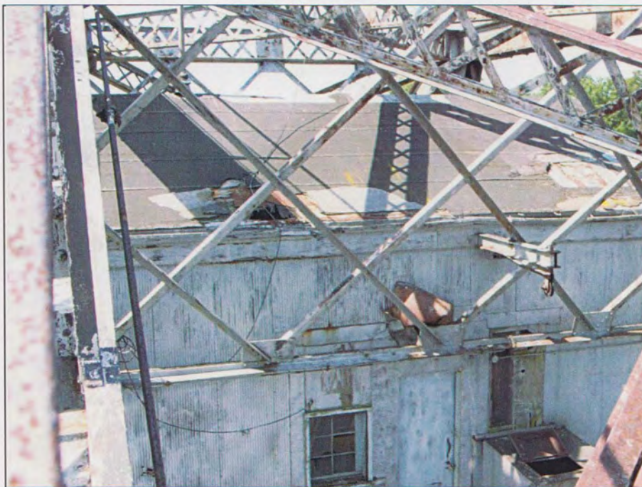
Figure 10. Detail of north side of roof of the control house.
