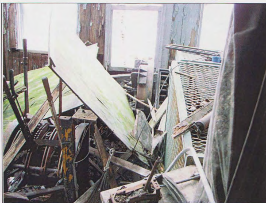
Figure 13. Machine room in the control house.
