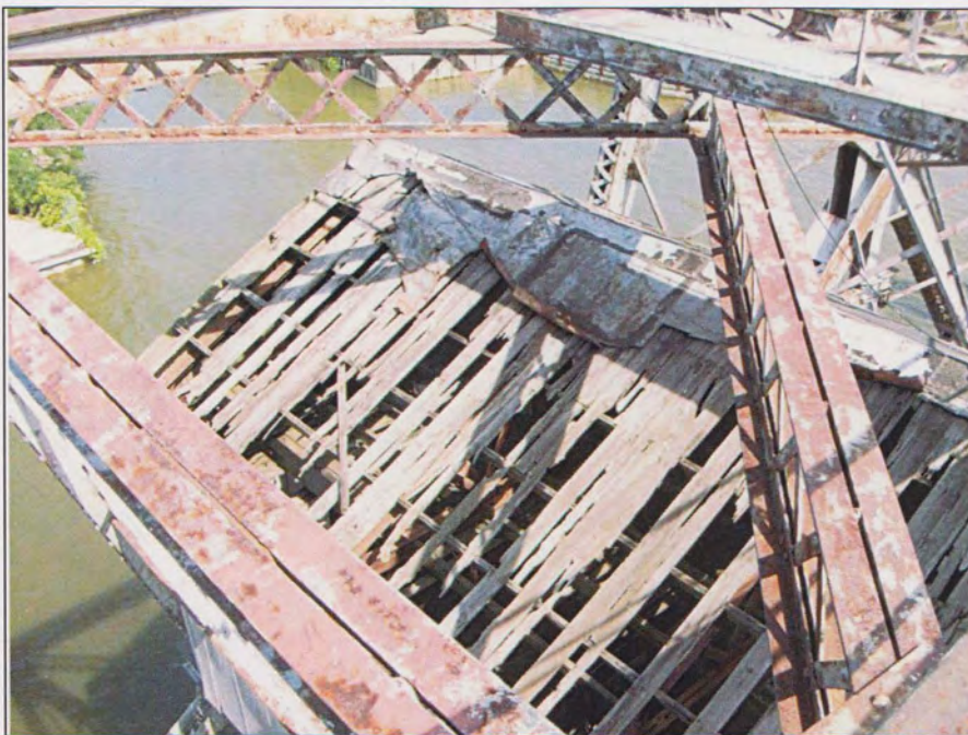
Figure 9. Detail of south side roof of the control house.
