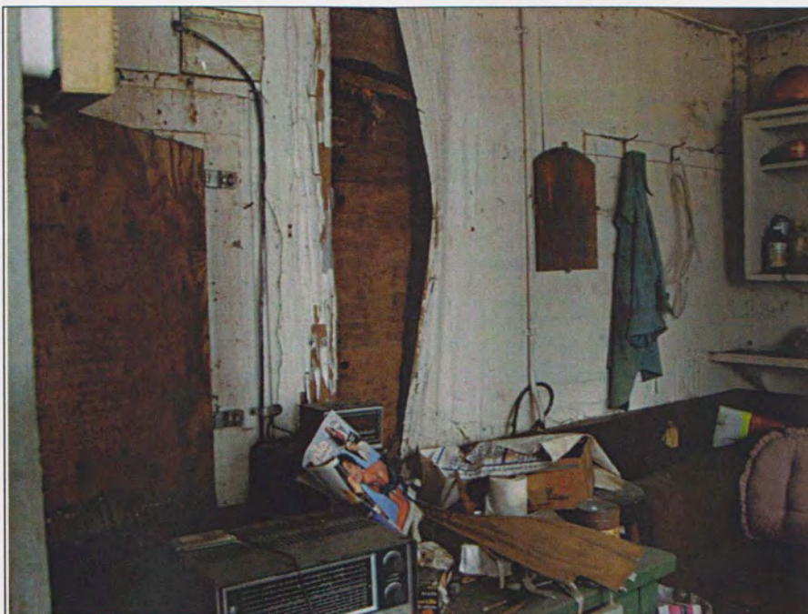
Figure 11. Interior office area of control house.
