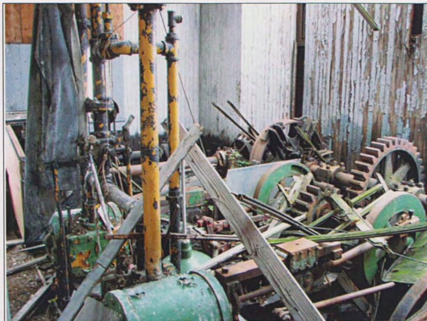
Figure 12. Machine room in the control house.
