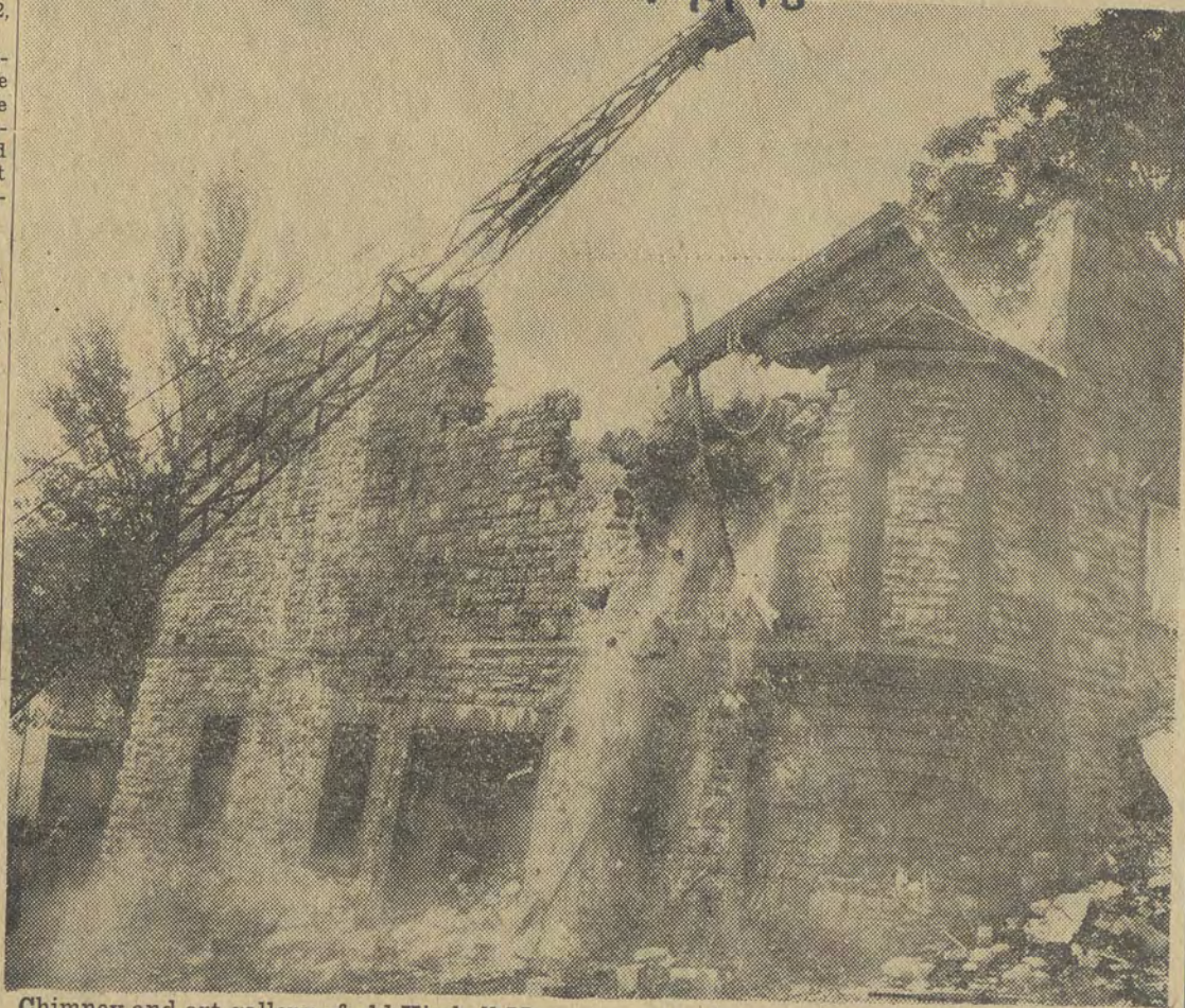
Chimney and art gallery of old Kimball Mansion crumbled yesterday and left city with one less landmark of Third Ward elegance as 1,200-lb. ball swung on derrick, connected.
