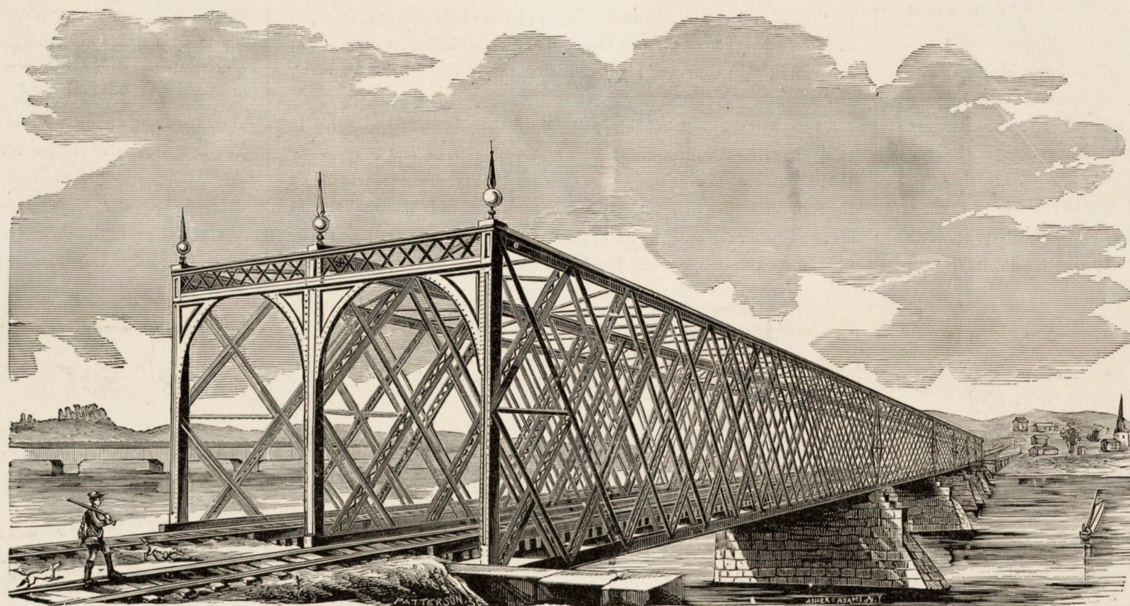
VIEW OF RAILROAD BRIDGE OVER CONNECTICUT RIVER, SPRINGFIELD, MASS.
