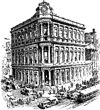
West Main Street Office 47 WEST MAIN ST.
