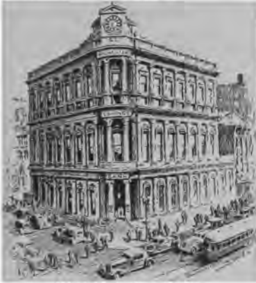
West Main Street Office 47 WEST MAIN ST.
