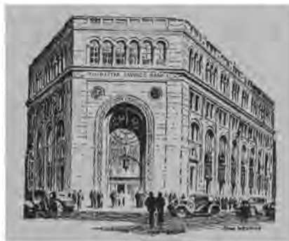
Franklin Street Office 40 FRANKLIN STREET
