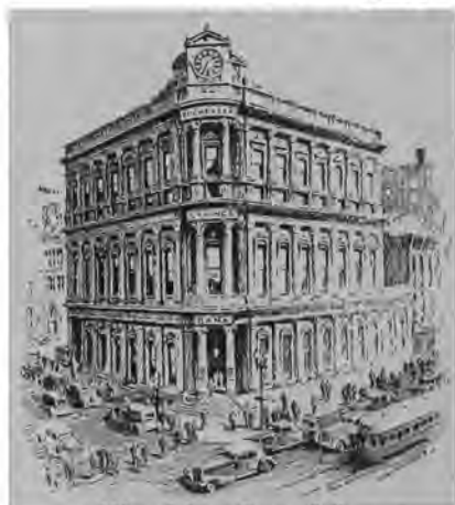
West Main Street Office 47 WEST MAIN ST.
