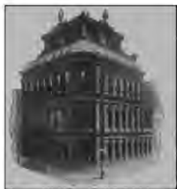
West Main Street Office 47 WEST MAIN ST.
