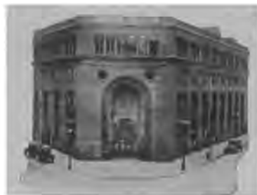
Franklin Street Office 40 FRANKLIN STREET
