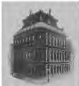
West Main Street Office 47 WEST MAIN STREET
