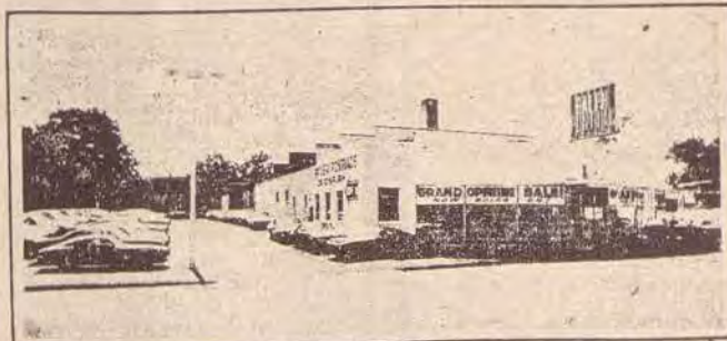
Visit Our Beautiful Air Conditioned Showroom...
