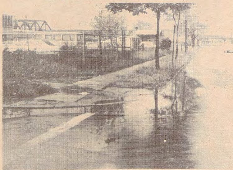
Flooded conditions at Wren and Driving Pk.
