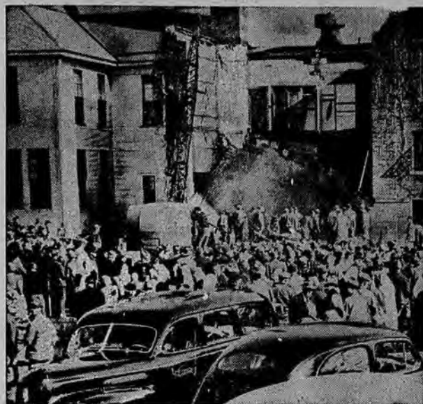
BLAST WRECKS SCHOOL . . . Crowds of anxious parents and volunteer rescue workers gathered quickly at the Baroda consolidated school at Baroda, Mich., following a boiler explosion in the basement of the school which killed one child and injured at least 16 others. When reports were first received at Chicago rescue planes with medical supplies were rushed to the scene.
