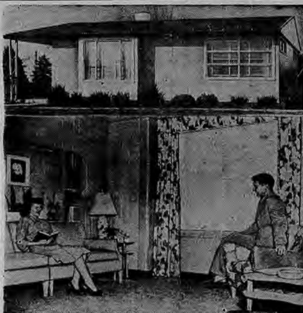
VETERANS FACTORY HOUSE. . . . First Lustron home to be completed was recently opened for inspection by the housing officials in Chicago suburban Hinsdale. Elmer Thiedel, former seabee, is shown in living room of the all-steel and porcelain-enameled house. This house, the first of a huge mass production, is designed to sell for approximately $7,000, not including lot.
