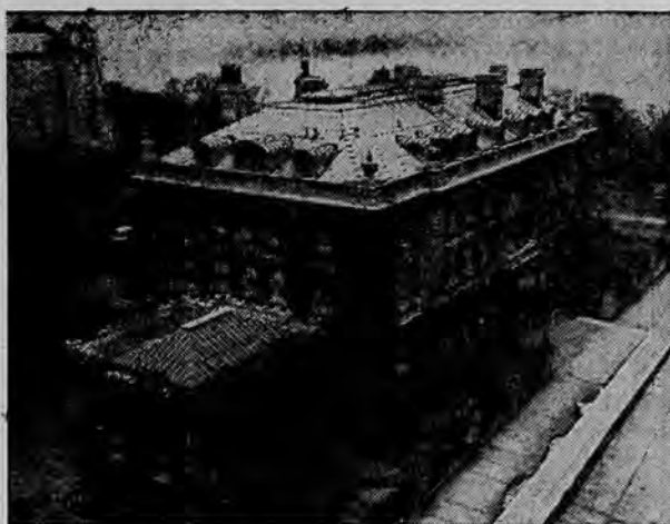
CARNEGIE MANSION TO UNITED NATIONS . . . View from an elevation of the palatial Carnegie mansion at New York City, which has been offered to the United Nations to serve as a club for delegates and an office building. The mansion, which covers an entire block front is said to have cost $1,000,000. It has been kept fully staffed for 44 years since it was first opened.
