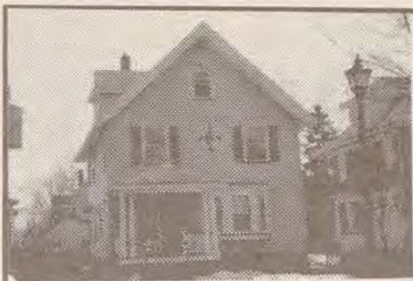
435 Augustine-picture perfect sided ,new carpeting, original woodwork
