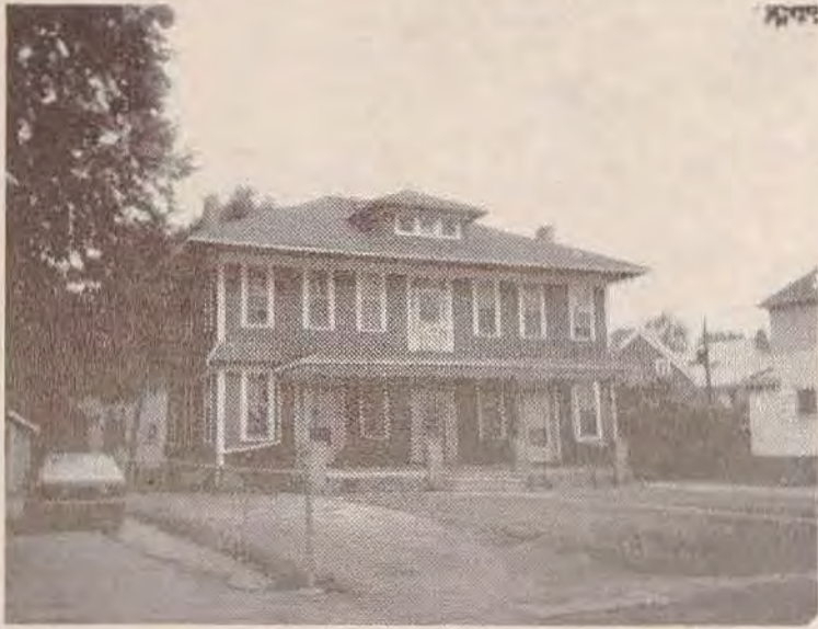
This home on Seyle Terrace was once a grand hotel which served the patrons of the Driving Park Race track during its hey day in the last century.
