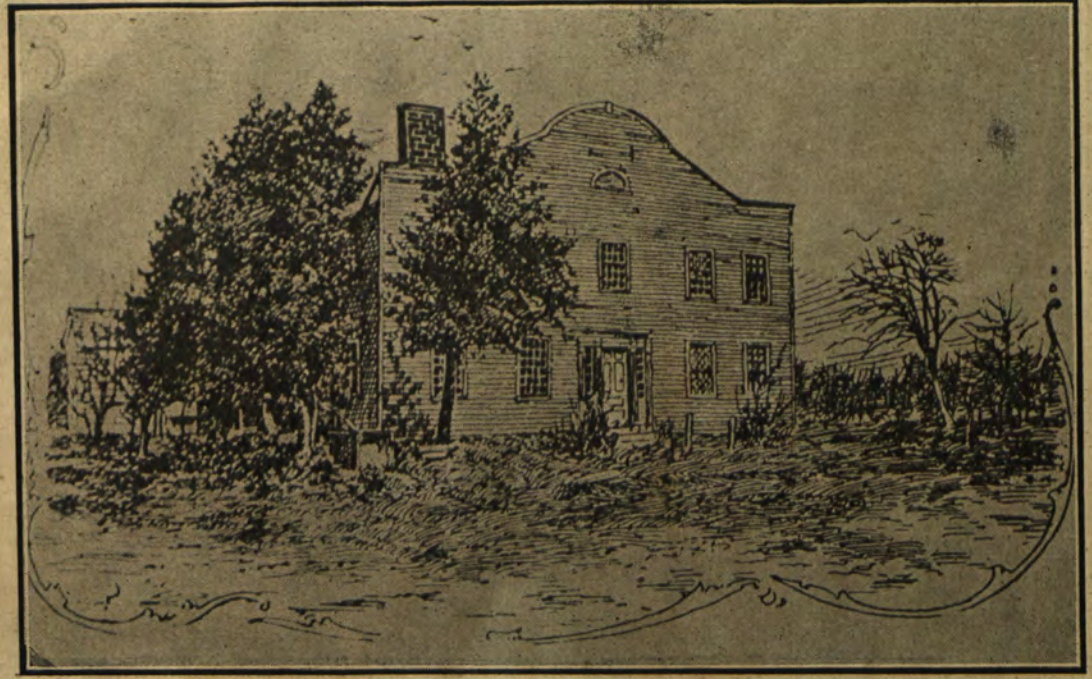
THE OLD "STEAMBOAT TAVERN" AT HANFORD'S LANDING.
