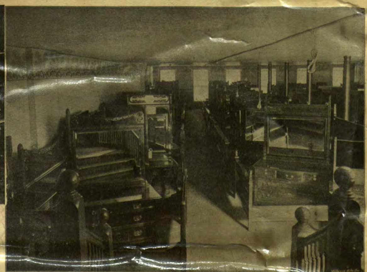
CHAMBER SUITES, Showing North Aisle of Third Floor, North Mill Street Building.
