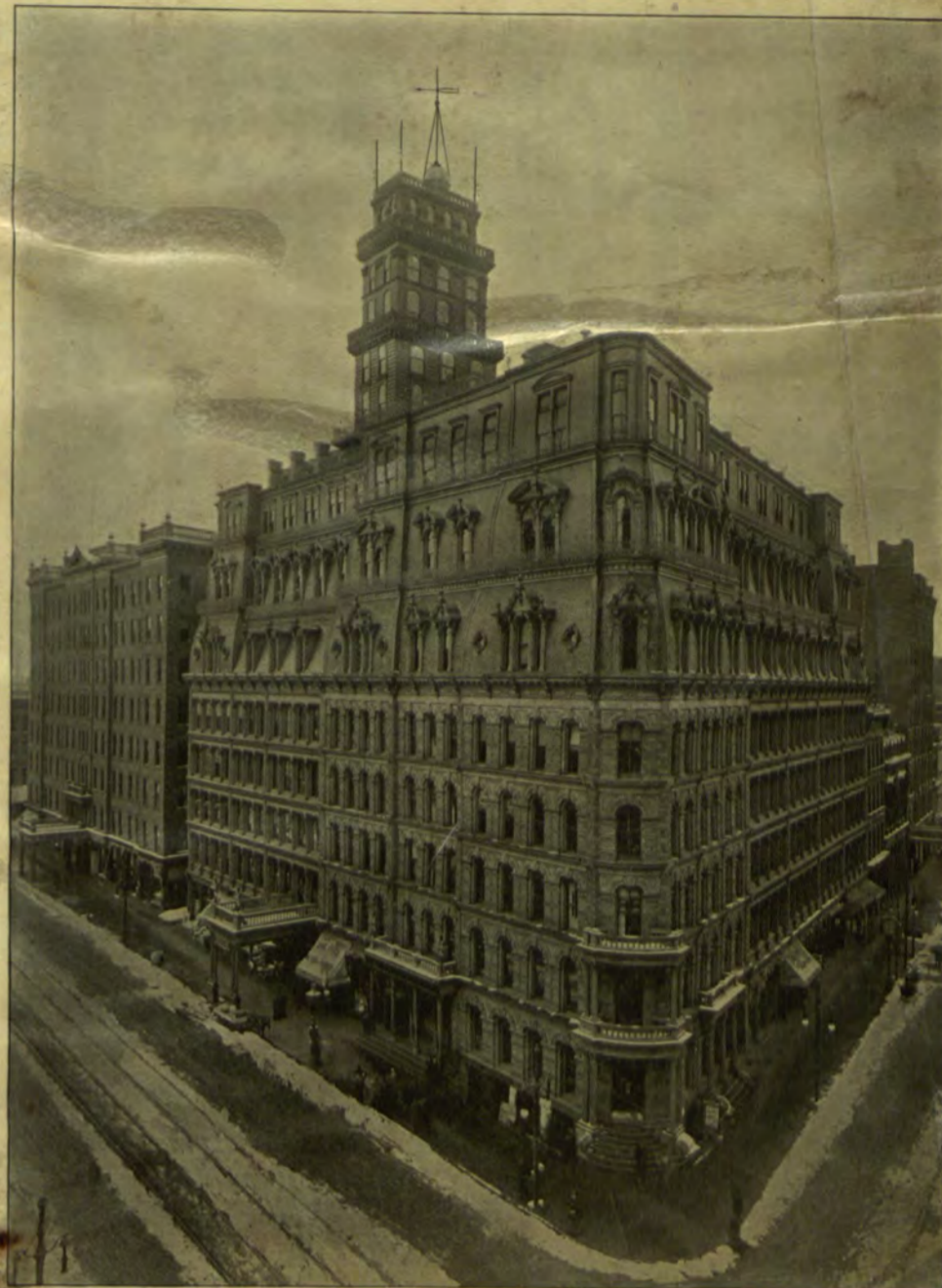
POWERS BUILDING AND POWERS HOTEL.
