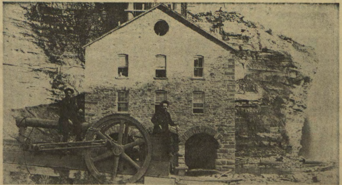
This view of generator station at the lower falls shows workmen posing on generating machinery being moved
