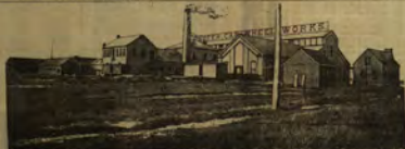
WATER WORKS, SOUTH SIDE.
