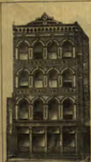
GEORGE C. STILES & CO. BOTTLEWORK BUILDING.
