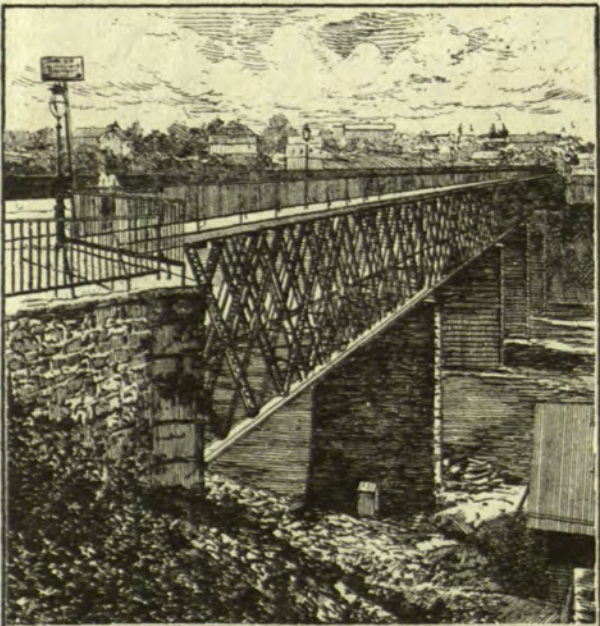
VINCENT STREET BRIDGE, BUILT AT LEIGHTON BRIDGE WORKS.
