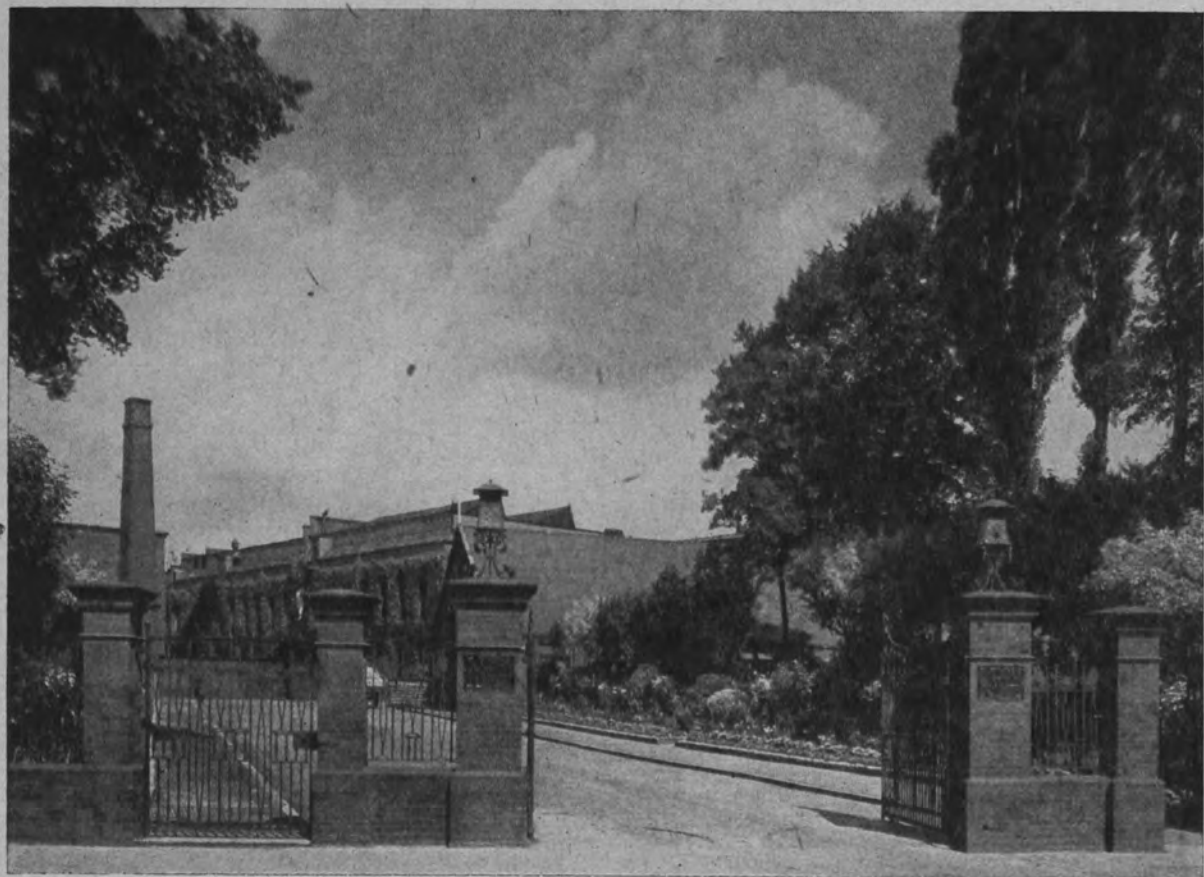
Trees, flowers and shrubbery beautify the entrance to the Eastman Kodak Works at Harrow, England.
