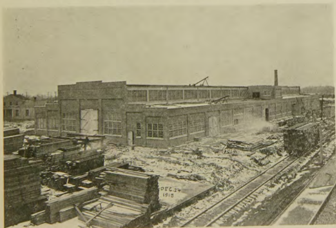
PHOTOGRAPH B: BUILDING OF THE GENERAL RAILWAY SIGNAL COMPANY, ROCHESTER, COMPLETED ON DECEMBER 4, 1915, HAVING TAKEN ONLY FIFTY-FIVE DAYS, TO ERECT. IN THIS BUILDING 80,000 SHELLS WERE MADE FOR THE BRITISH GOVERNMENT.
